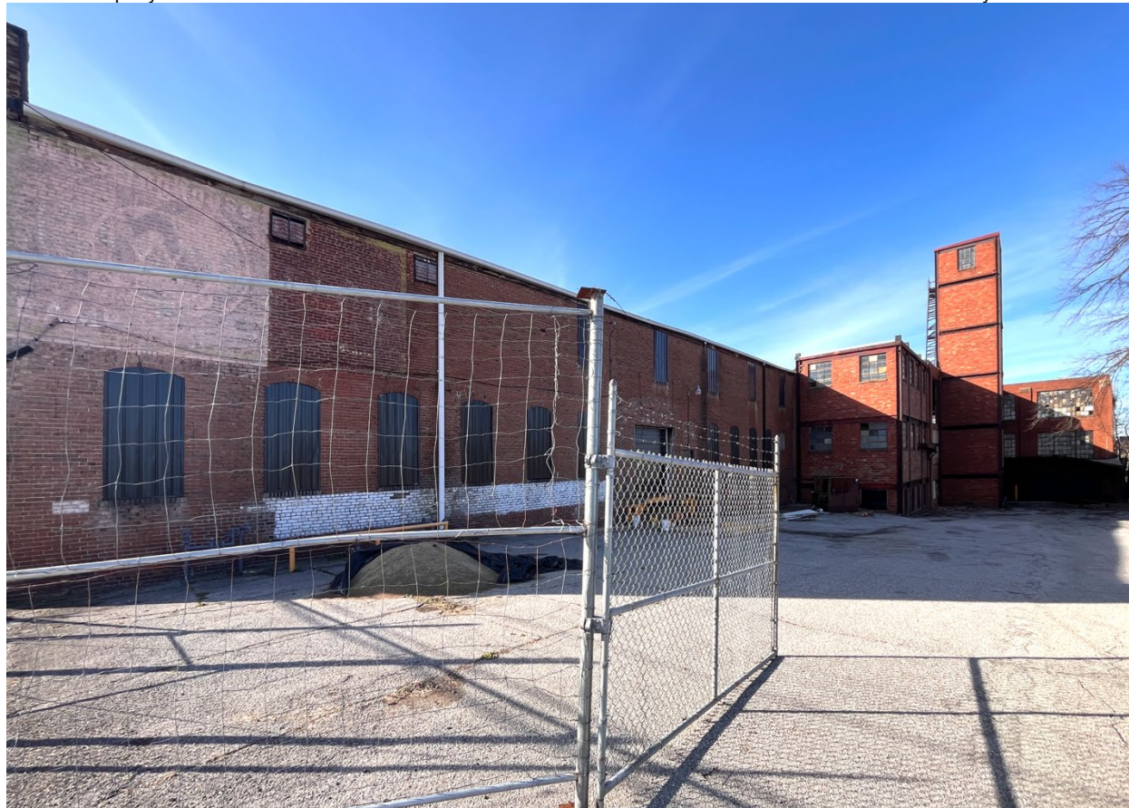
South elevation (const. 1944, 1950s) and east elevation (const. 1919)
