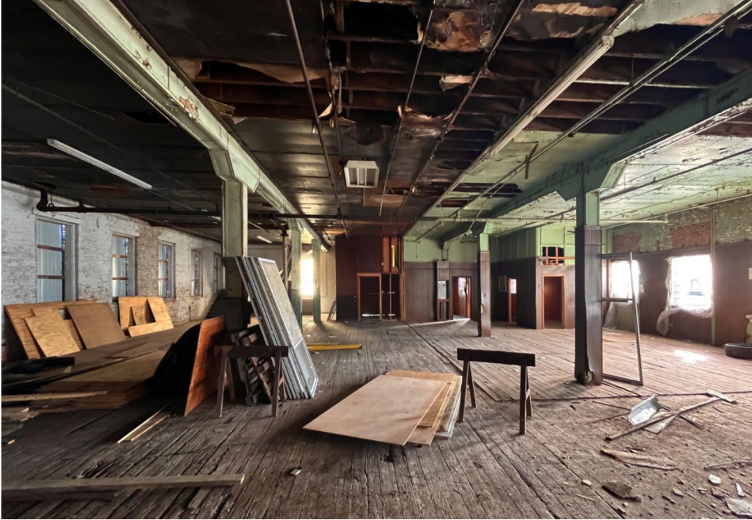
First floor, 1919 section of plant, facing south
