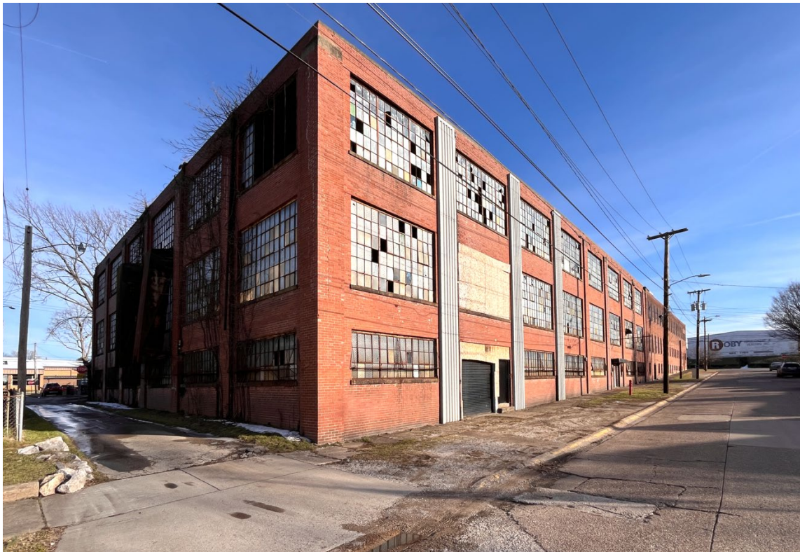
North elevation (const. 1944) and west elevation (const. 1919, 1937, 1944)
