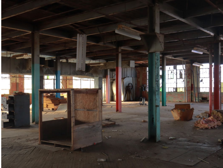
1944 addition third floor, facing northwest
