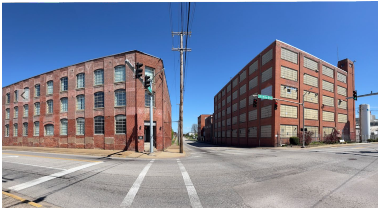
Photograph of Ken-Rad main tube plant c. 1937 wing (right), April 2026. Photo credit: Jason Schubert
