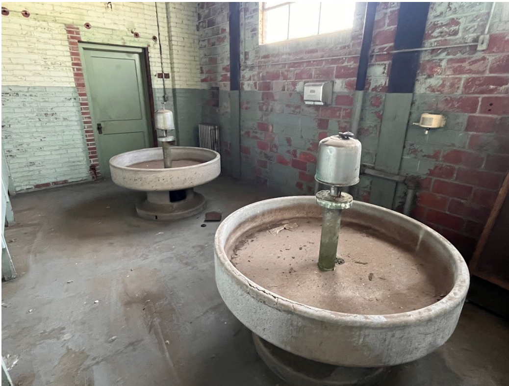
Restroom in 1946 addition
