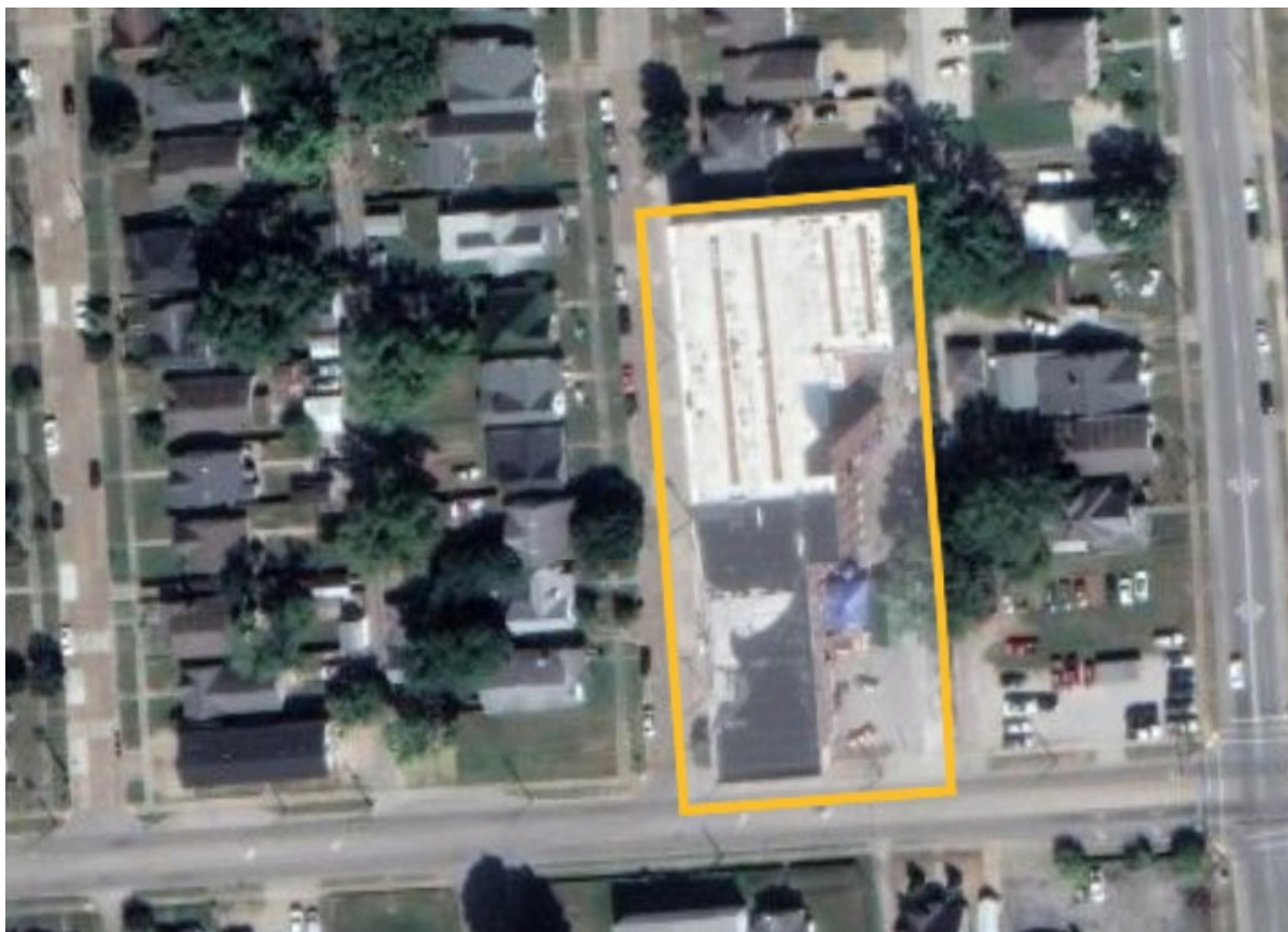
Ken-Rad Plant, Owensboro KY
