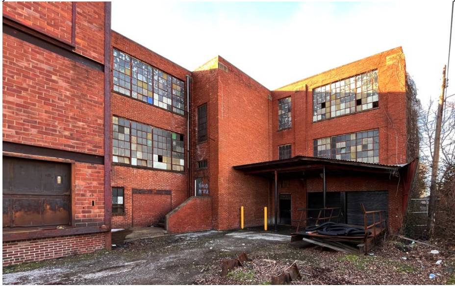
South elevation (const. 1944) and east elevation (const. 1944 and 1950s)
