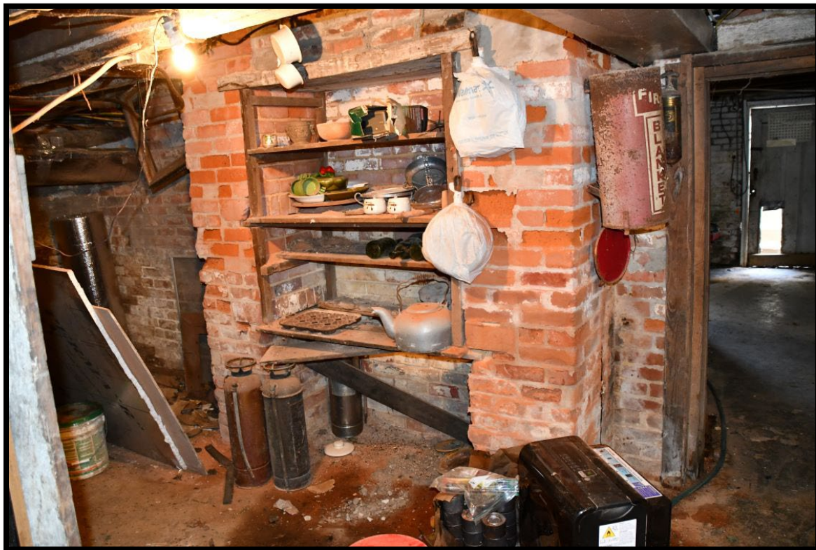
Plate 17 Basement level of detached kitchen, warming rack (on the west elevation of the chimney), note repointed brick. (Photo 0017).
