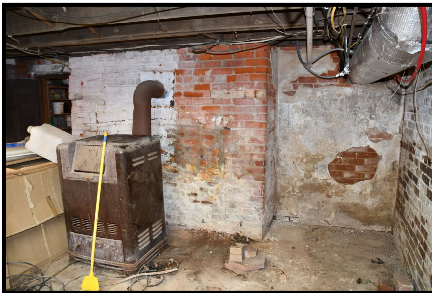
Plate 16 Basement level of detached kitchen, fireplace (on the east elevation of the chimney) enclosed but lintel visible. (Photo 0016).
