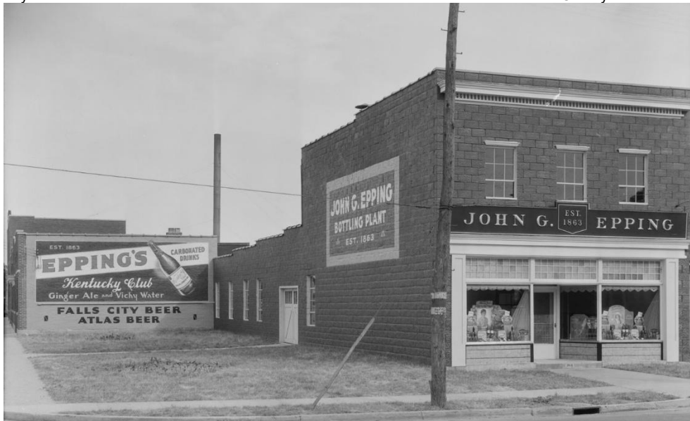
Front facade, John G. Epping Bottling Works, Year of Opening - 1933. 4
