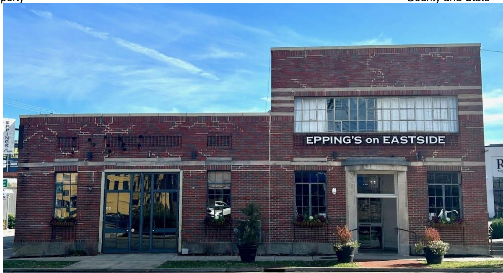
Front facade, John G. Epping Bottling Works, 2024. 3
