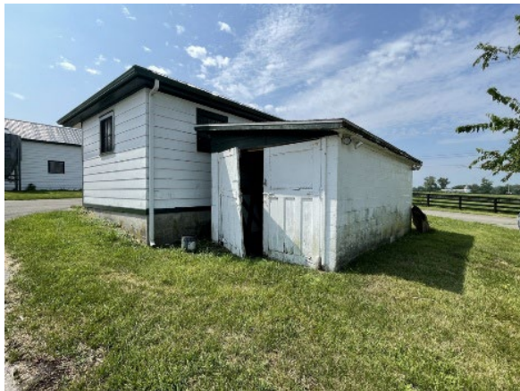
#9 Concrete Block Shed
