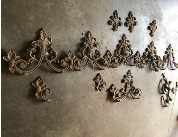
Photograph of iron porch parapet elements
