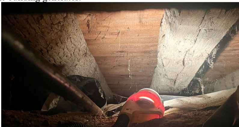
Photograph of original, bark-covered joist under house's central block
