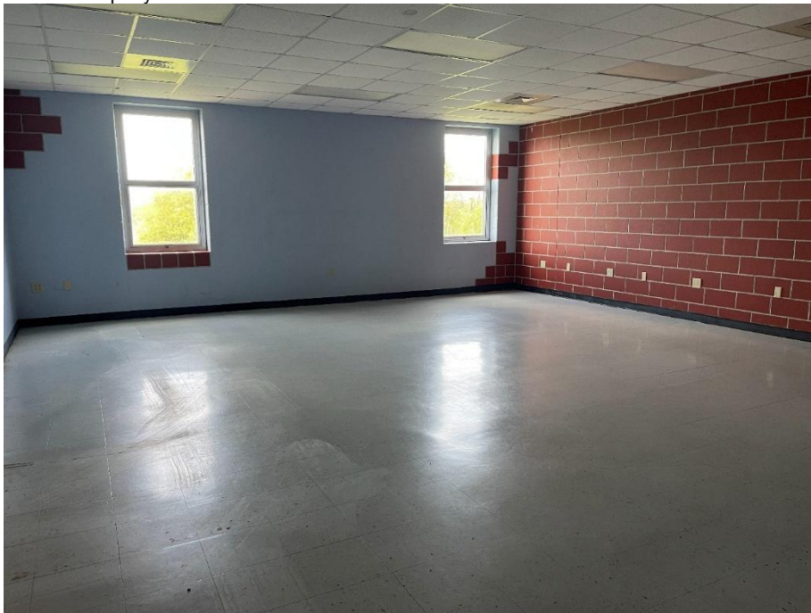
Typical of 4 classrooms in the addition looking Northeast.
