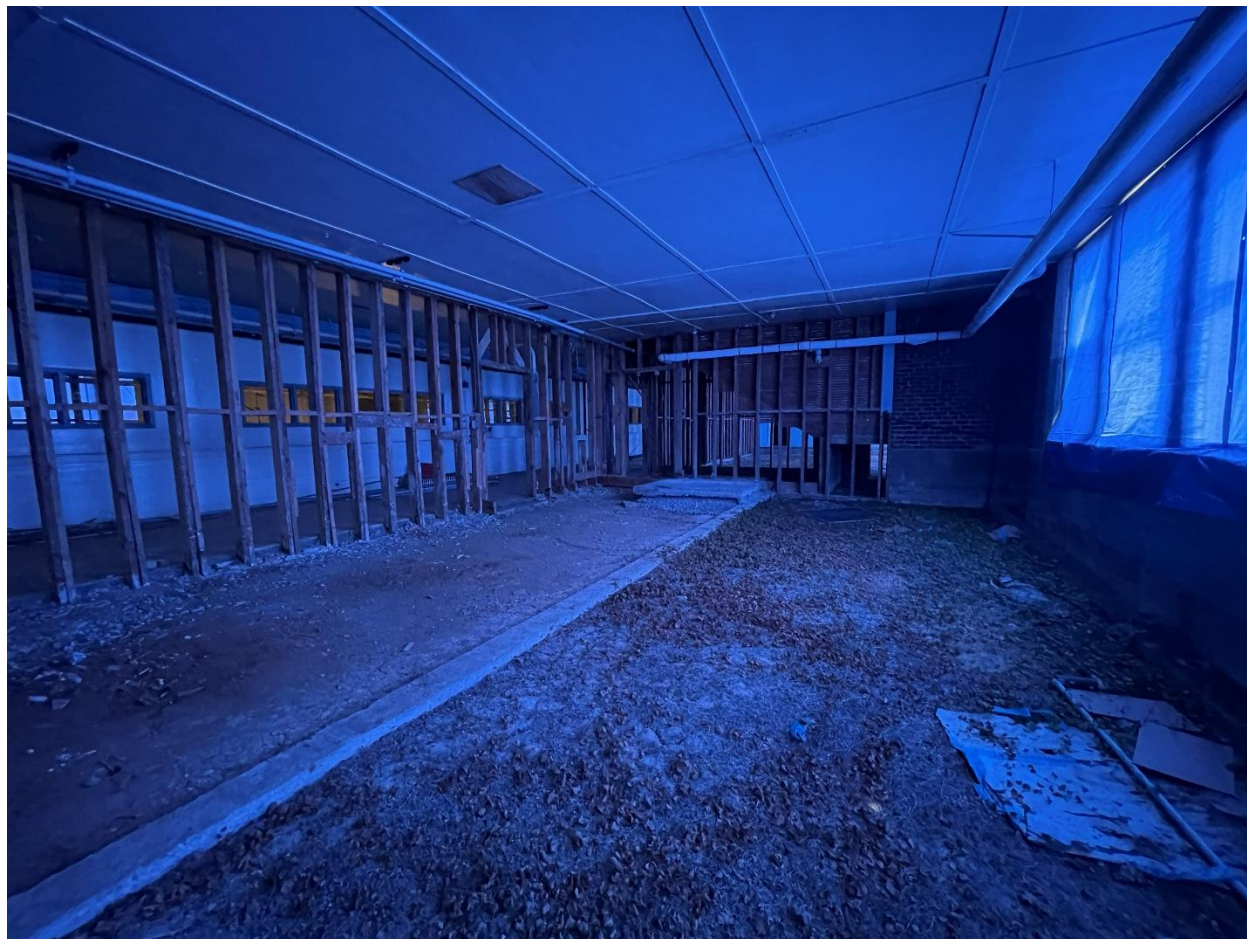
Lower level: Original kitchen converted to a classroom looking East.
