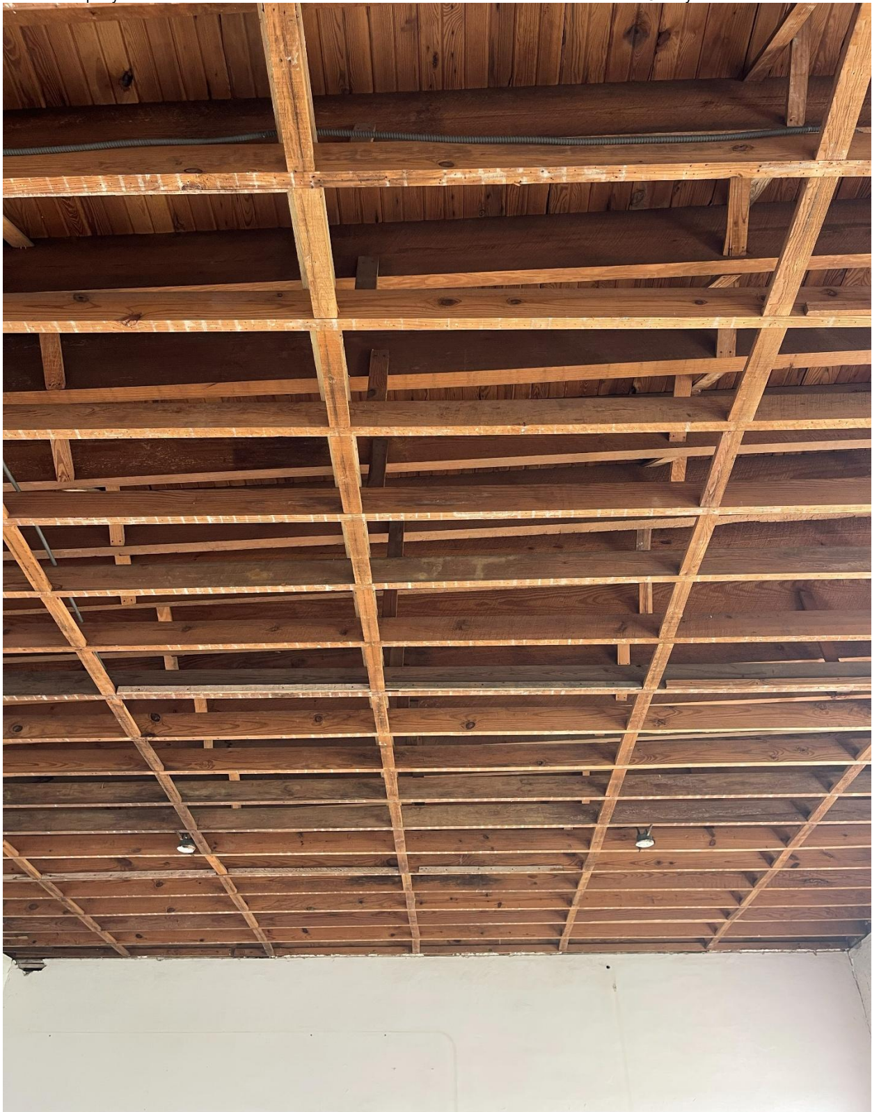
View of ceiling joist and roof rafters.
