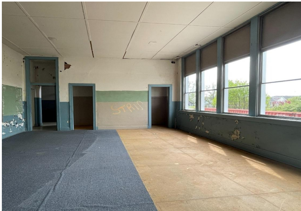
Second level classroom where the windows face West. Note the entrance and exit for cloak room, the original door and transom frame.
