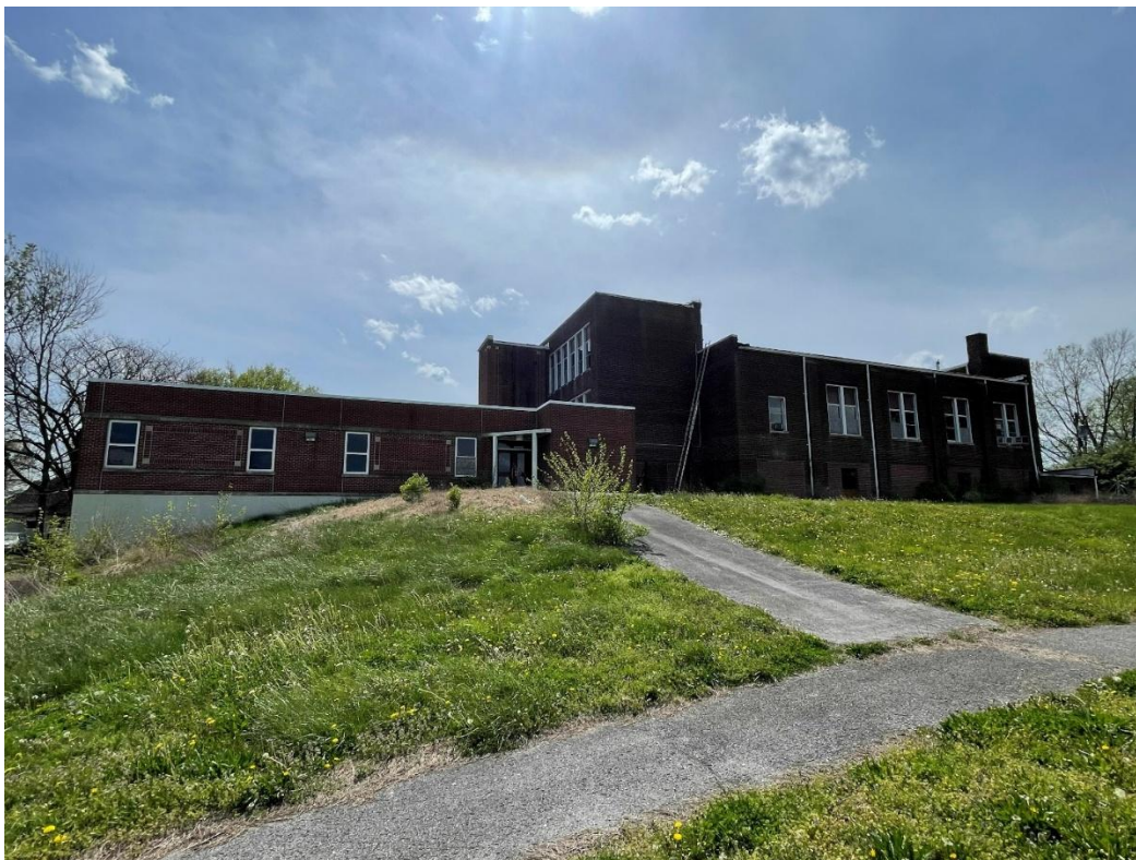
North elevation with addition.
