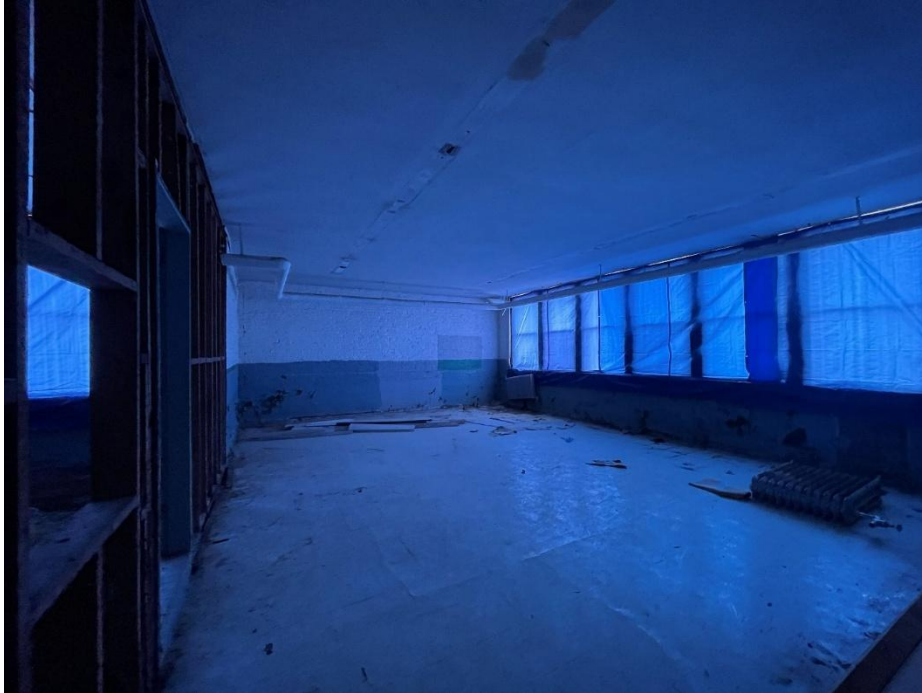
Lower level: Original cafeteria converted to a classroom looking Southwest.
