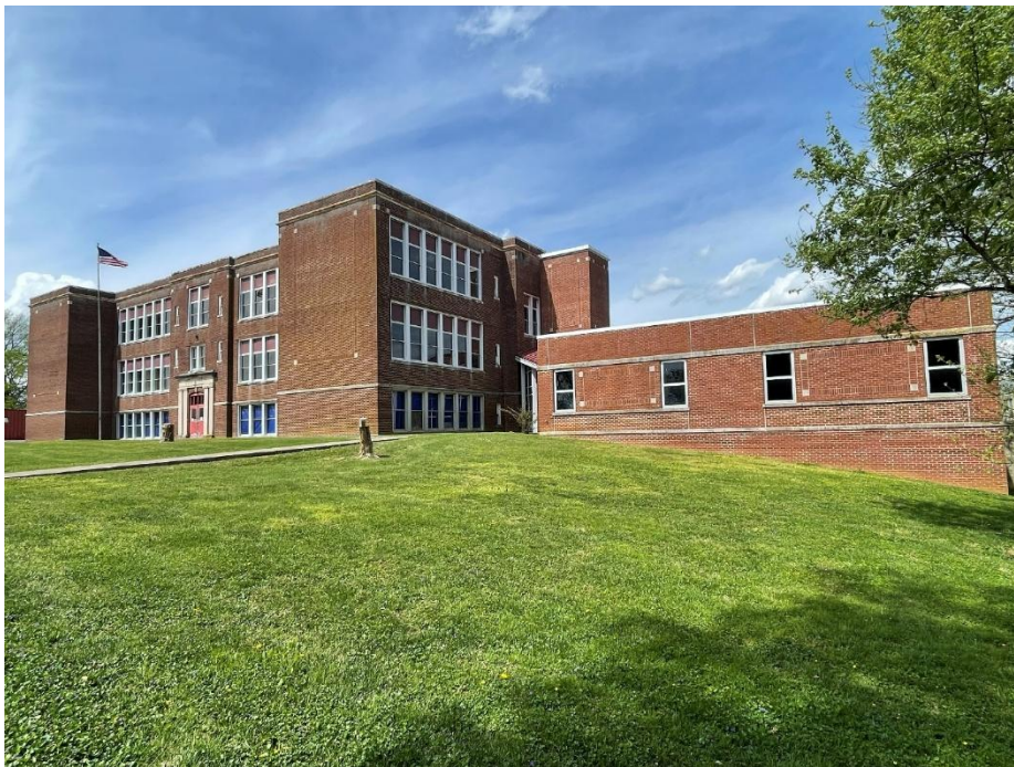
East side photo with addition looking Northwest
