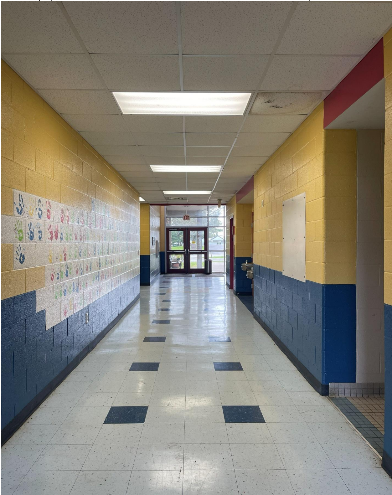
View of hallway and entrance to addition looking South.
