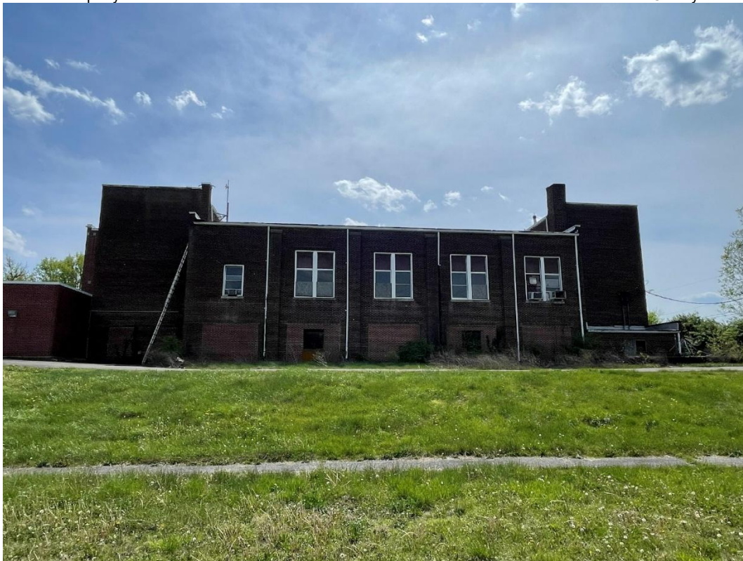
North elevation of the original structure.
