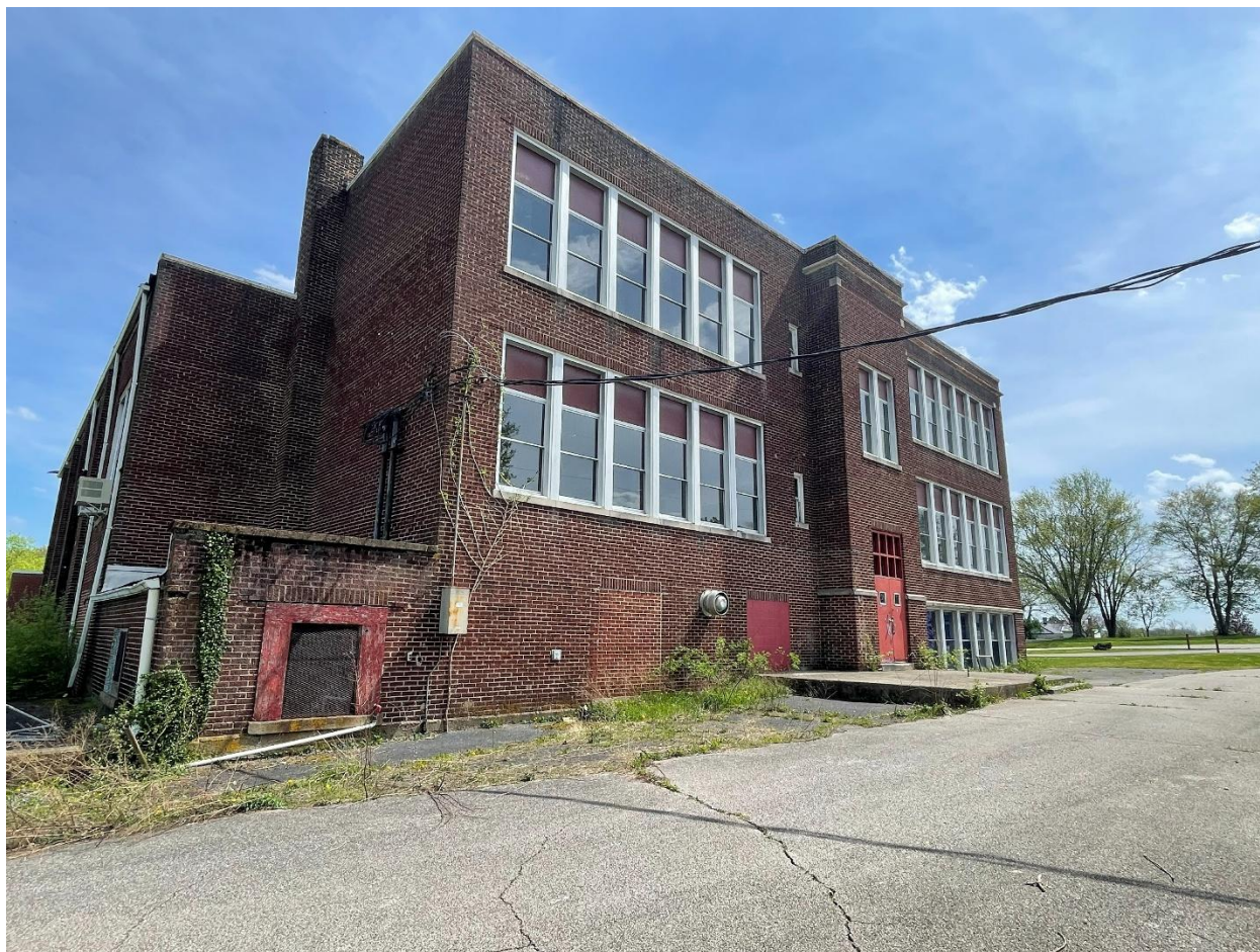
West side photo looking Southeast.
