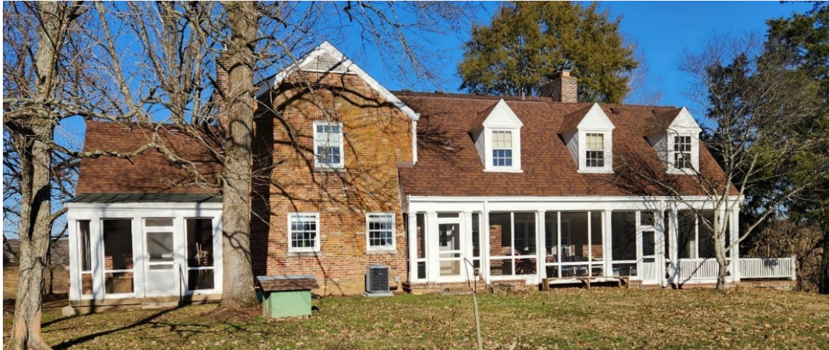
Julian Farm, Main House, South elevation
