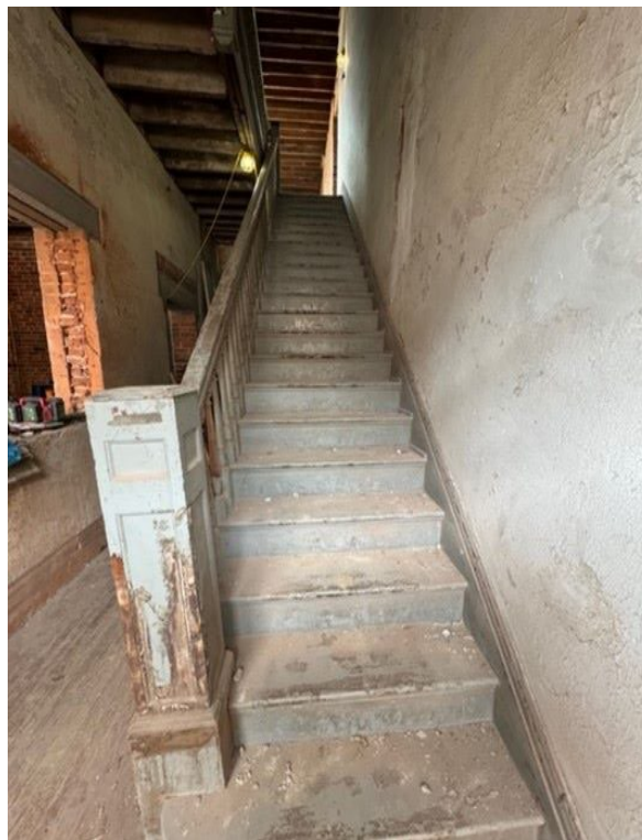
First Floor Stairway
