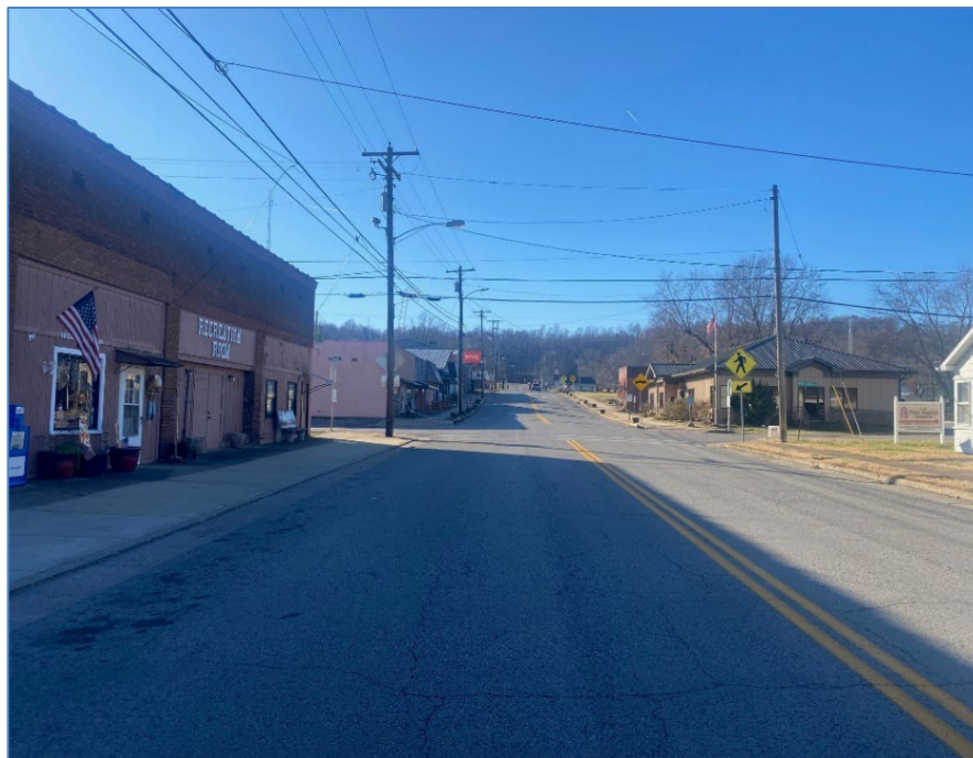
Figure 4 - Morton's Gap- looking west
