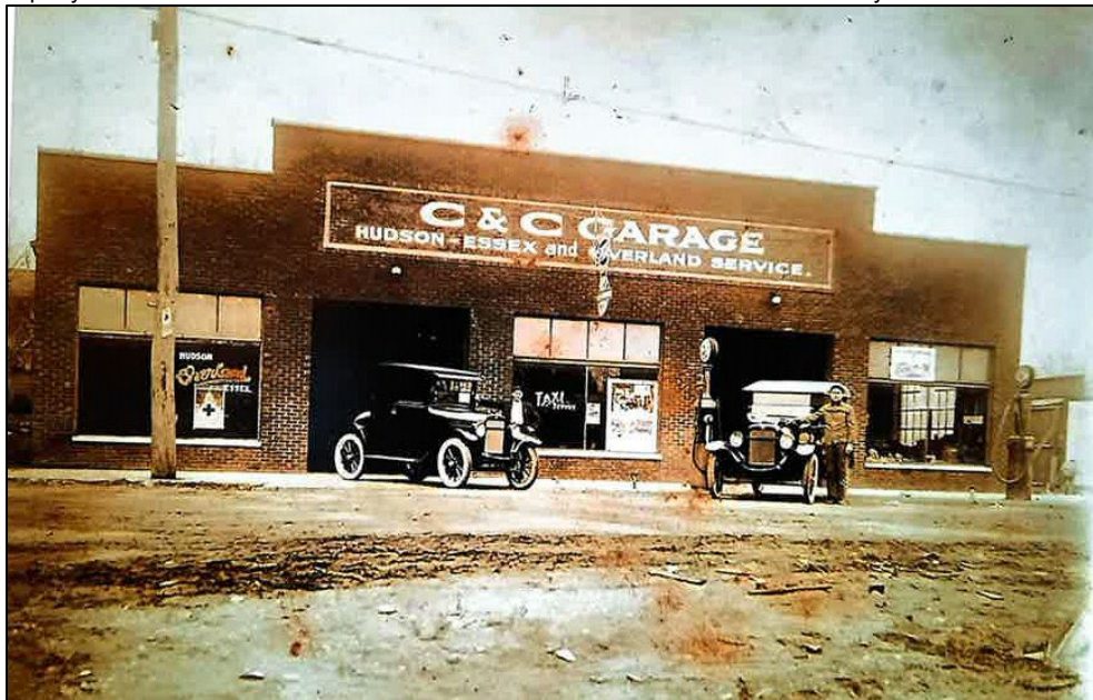
Figure 3: C & C Garage
