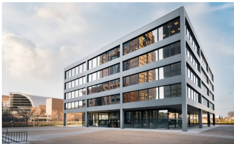
Main south facade [credit: PRG Commercial Property Advisors]
