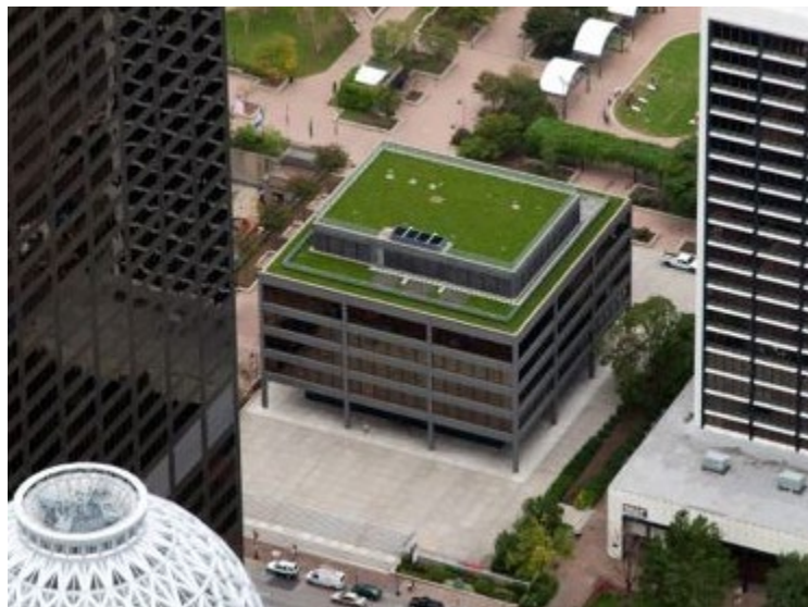
Vegetative roof and penthouse, photo ca. 2009 (GreenRoofs.com)
