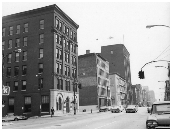
Ca. 1963, Keller Bldg at left before clearance.
