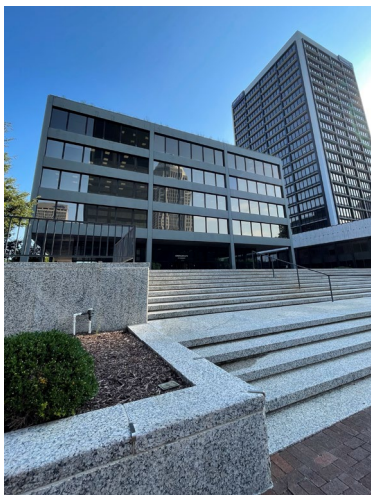
South façade and plaza steps
