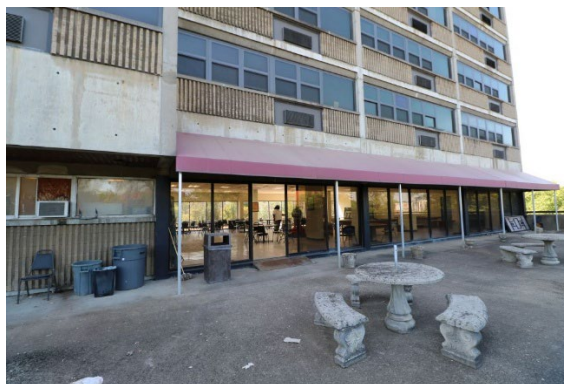
Photo 9, showing obscured balcony
