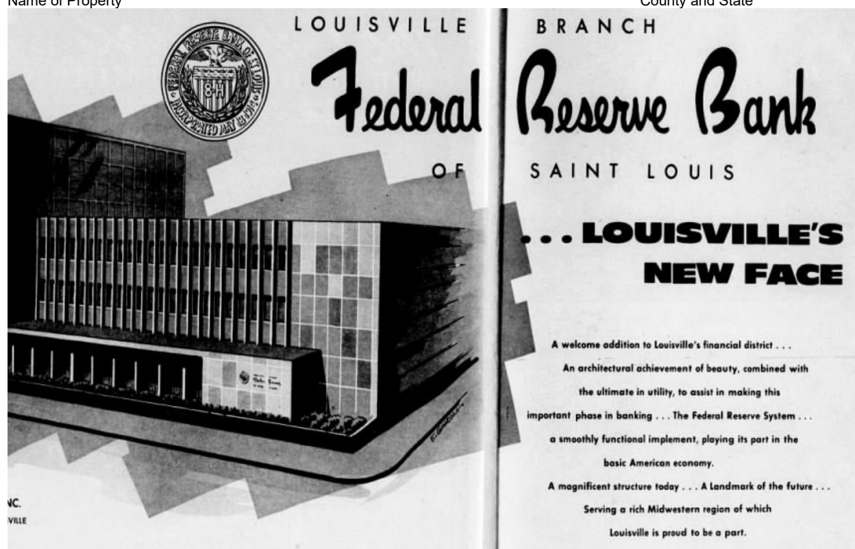
Advertisement for the new Louisville Branch Federal Reserve Bank. Caption reads, "A welcome addition to Louisville's financial district...an architectural achievement of beauty, combined with the ultimate in utility, to assist in making this important phase in banking...the Federal Reserve System...a smoothly functional implement, playing its part in the basic American economy. A magnificent structure today...A landmark of the future...serving a rich Midwestern region of which Louisville is proud to be a part." 43
