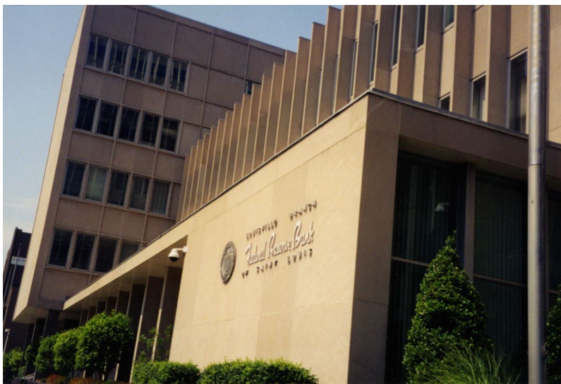
Louisville Federal Reserve Bank, showing old signage, courtesy of FRASER.
