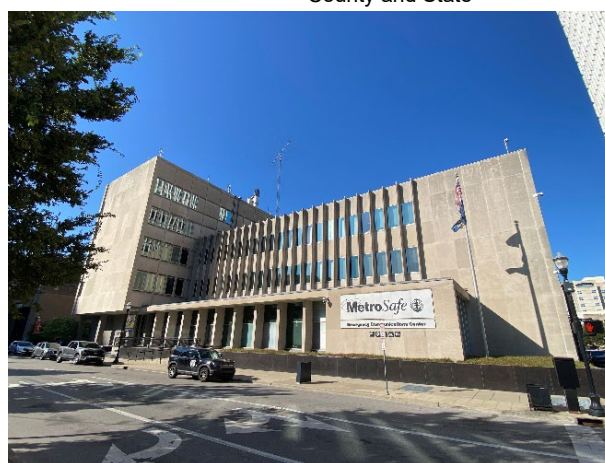
East Façade along 5 th St.
