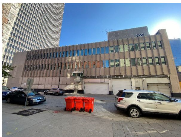
West Façade along Armory Pl.
