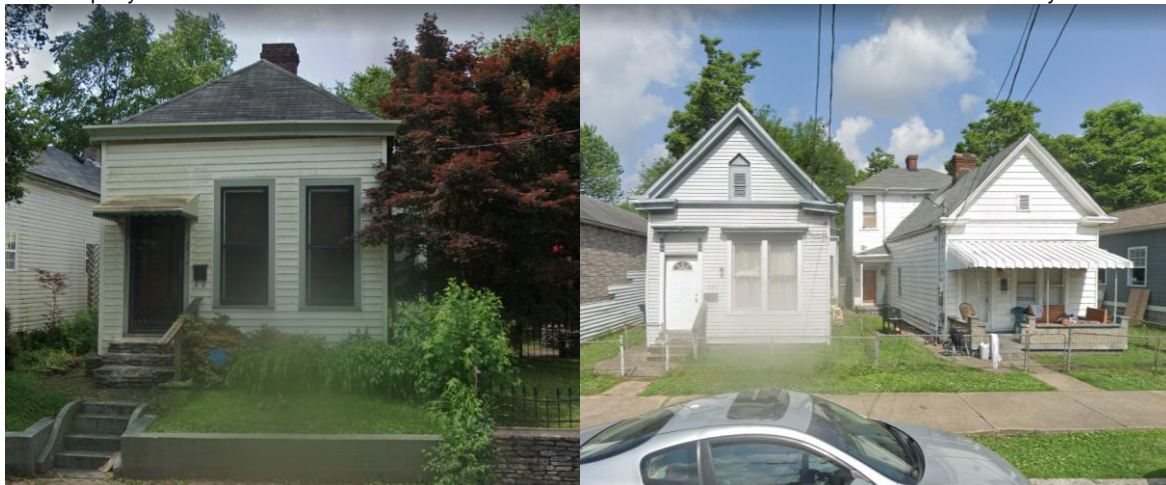
Rank 2: 2310 Griffiths Ave.-openings intact; material changes Rank 2: 334 & 336 N. 23 rd St.-openings intact; material changes
