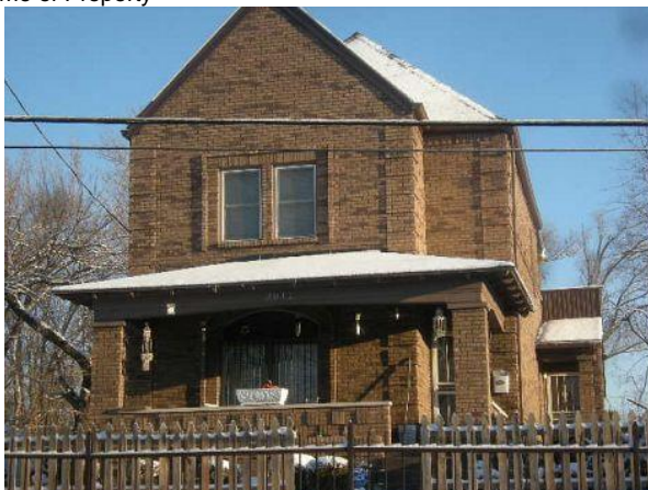
Rank 4: 3011 Bank St.-wood weatherboard siding replaced with brick
