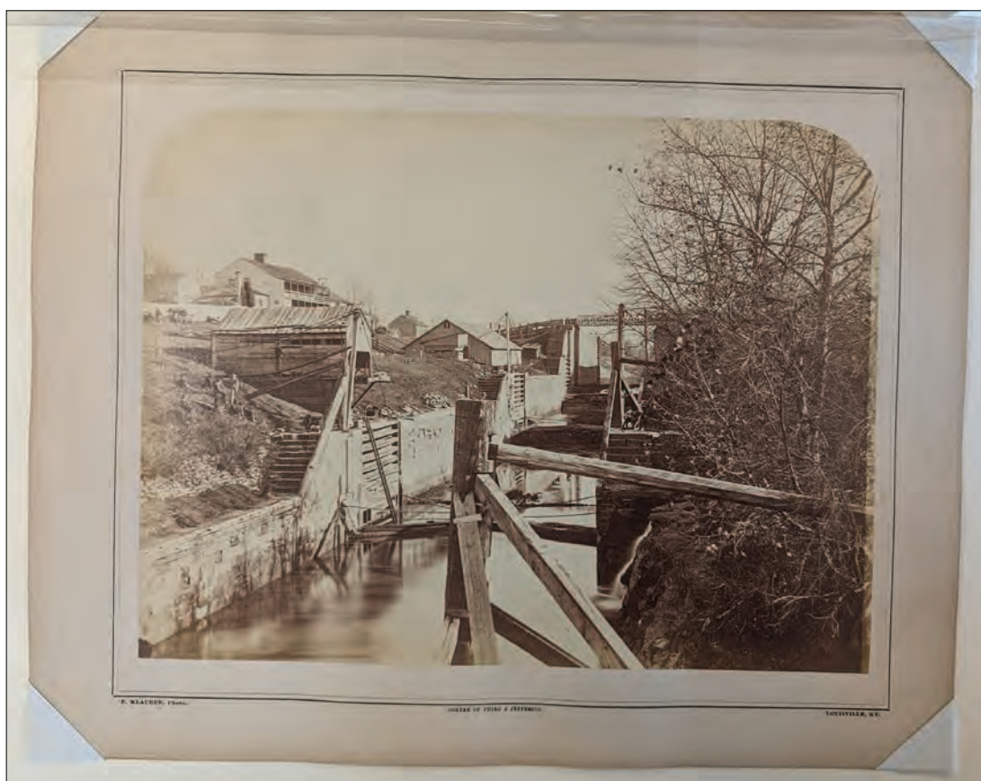
Photograph of the Scowden Locks at the Louisville and Portland Canal, circa 1871 (Source: Louisville & Portland Canal Collection, Filson Historical Society)
