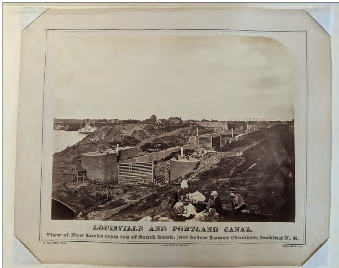
View of Construction of the Scowden Locks at the Louisville and Portland Canal, circa 1871 (Source: Louisville & Portland Canal Collection, Filson Historical Society)
