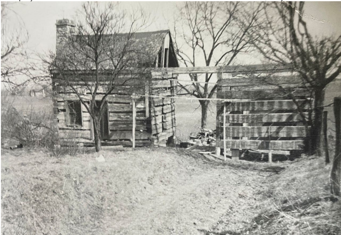
Figure 8. The two cabins being connected to create the dogtrot, ca. 1936.
