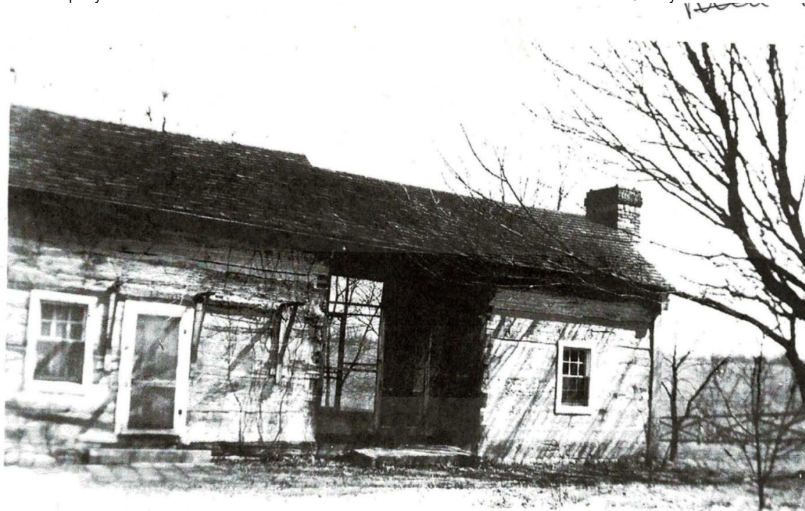
Figures 7 and 8. Historic Images C. 1940s showing the completed dogtrot and the screened-in opening (which occurred ca. 1947) before fully enclosing it in ca. 1950.
