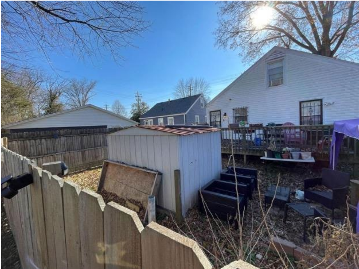
Photo 19: North Facing Side of the Braden House, Looking Southeast
