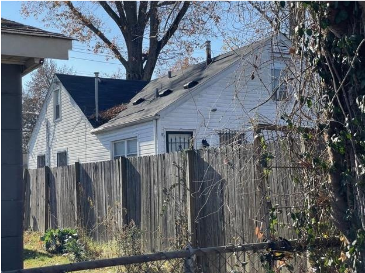
Photo 16: Northeast Facing Corner of the Braden House, Looking Southwest
