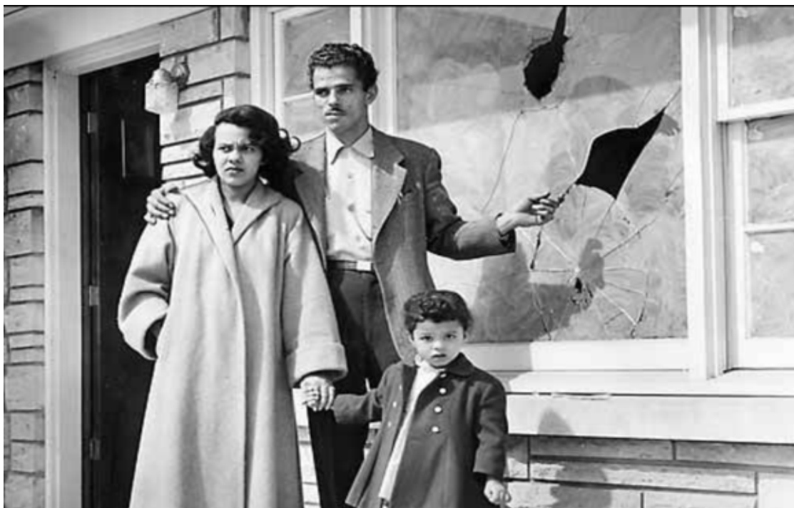
The Wade Family and the Damage Done to Their House, The Courier-Journal May 17, 1954
