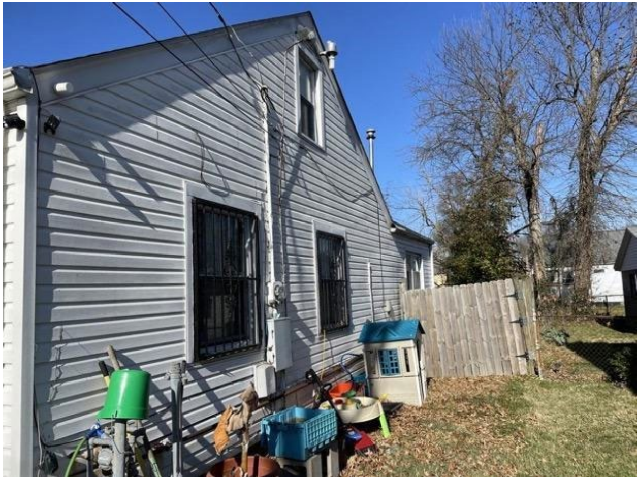
Photo 14: East Facing Side of the Braden House, Looking Northwest
