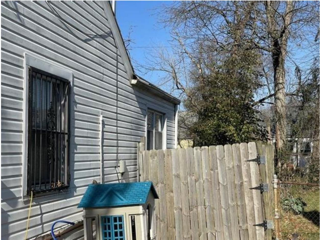
Photo 15: East Facing Side of the Braden House, Looking Northwest
