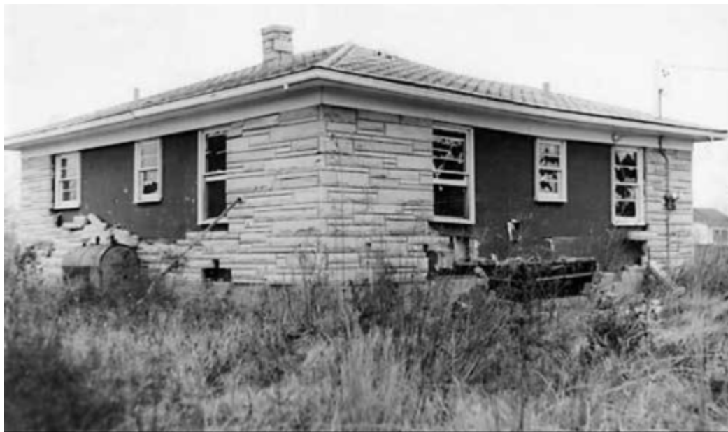
The Wade House After the Explosion, The Courier-Journal , 1954
