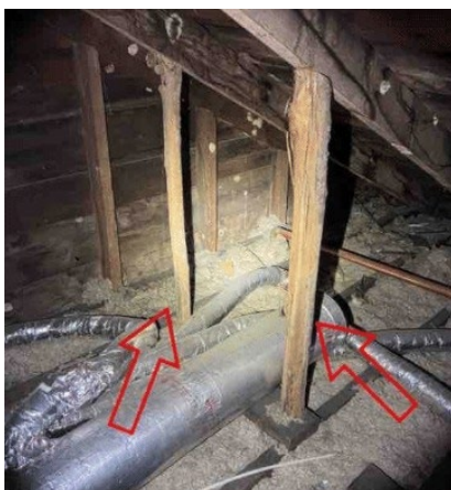
Locust Tree support beams
