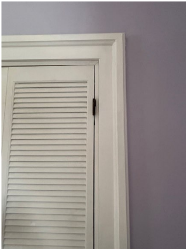
Close-up example to upstairs door trim
