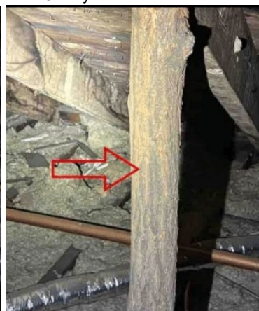
Locust tree beam (close up)
