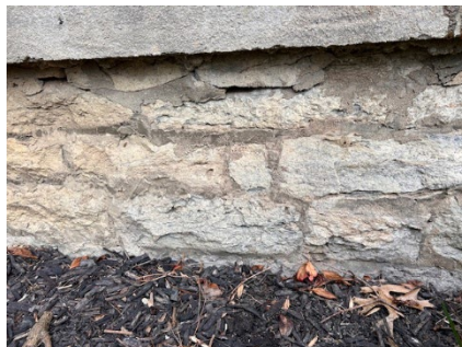
Raised coursed rubble stone foundation
