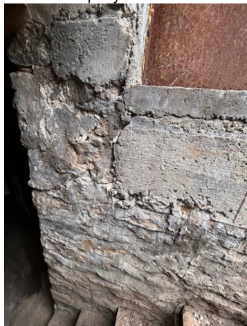
Raised coursed rubble stone foundation
