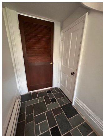
Original door trim and door of closet under the stairs
