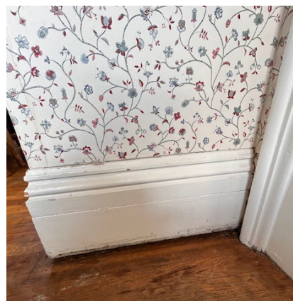
Example of First floor 11-in wood molding
