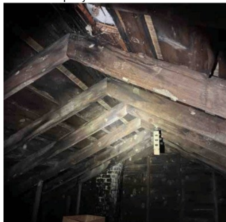
Underside of side-gabled roof
