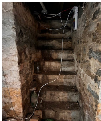
Thick stone steps (North)
