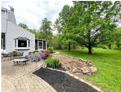
Kitchen under sloped roof/back porch
