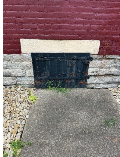
Iron Covers over basement window
