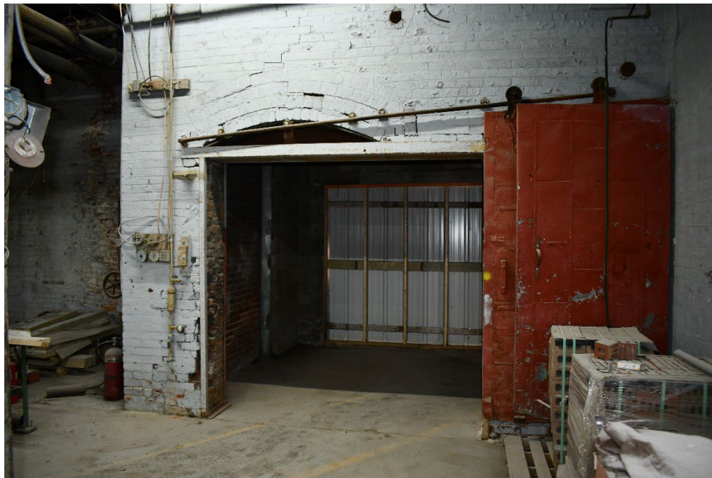
Figure 21 First floor, entrance to combined elevator and stair tower. (0015)
