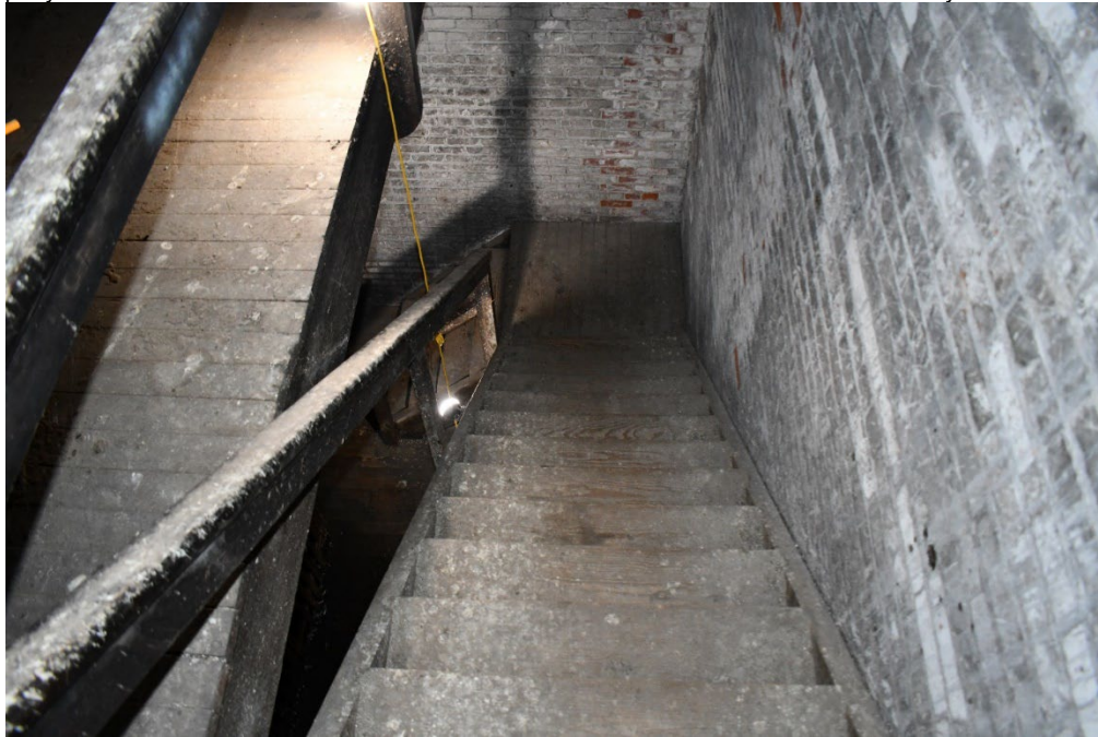
Figure 26 Fourth floor, stairs to third floor. (0020)
