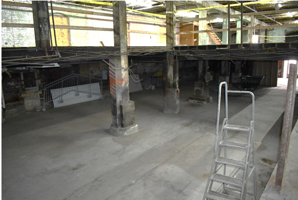
Figure 19 First floor, elevated wooden loft above the loading platform. (0013)
