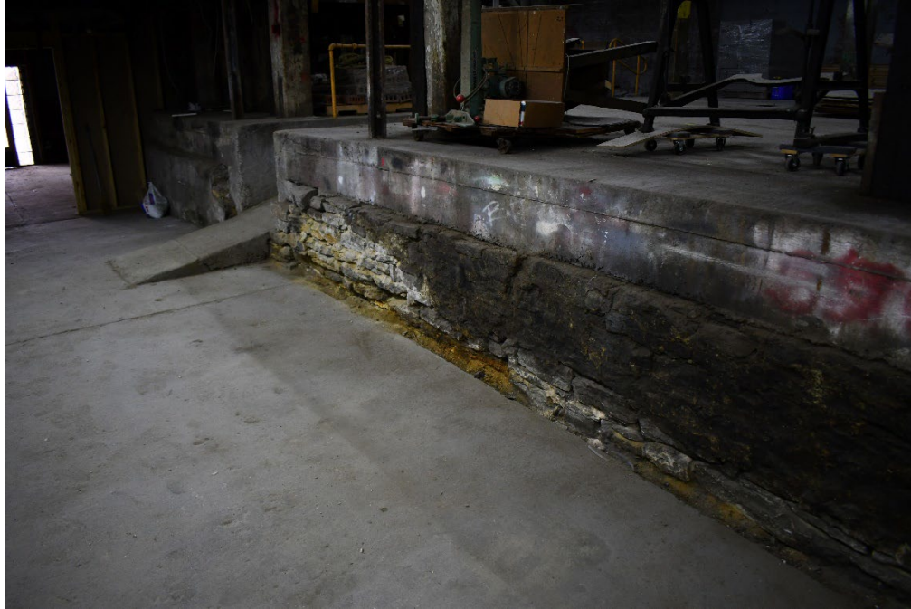
Figure 18 First Floor, elevated loading dock. (0012)
