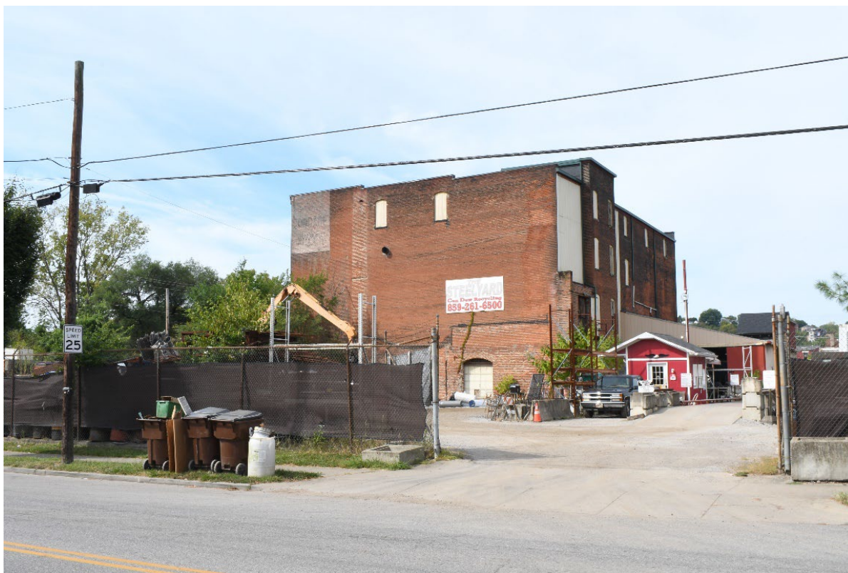
Figure 13 North elevation of Overman Schrader Cordage Company Building, looking SW, steelyard in foreground, note non-contributing modern shed. (0007)
