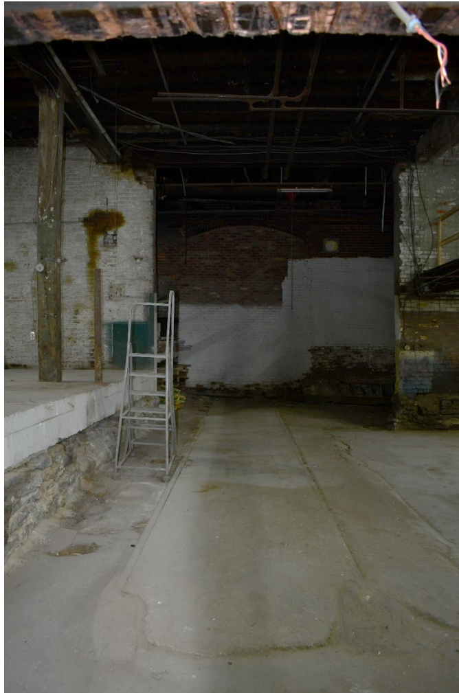
Figure 17 First Floor, elevated loading dock, note railroad track remnants. (0011)
