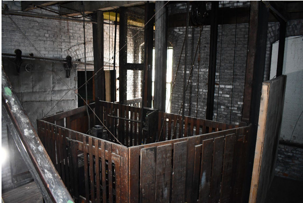
Figure 24 Third floor, combined elevator and stair tower. (0018)
