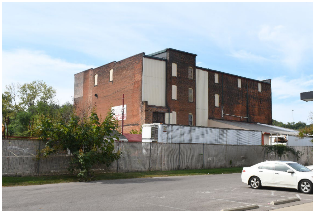
Figure 11 North elevation of Overman Schrader Cordage Company Building, looking SW. (0005)
