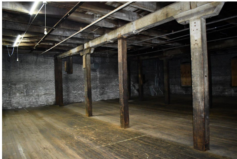
Figure 23 Third floor, former spinning room. (0017)
