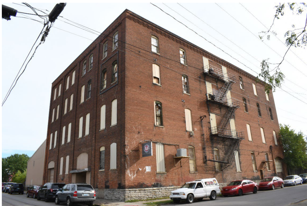
Figure 7 West elevation/Primary façade and south elevation of Overman Schrader Cordage Company Building, looking NE. (0001)
