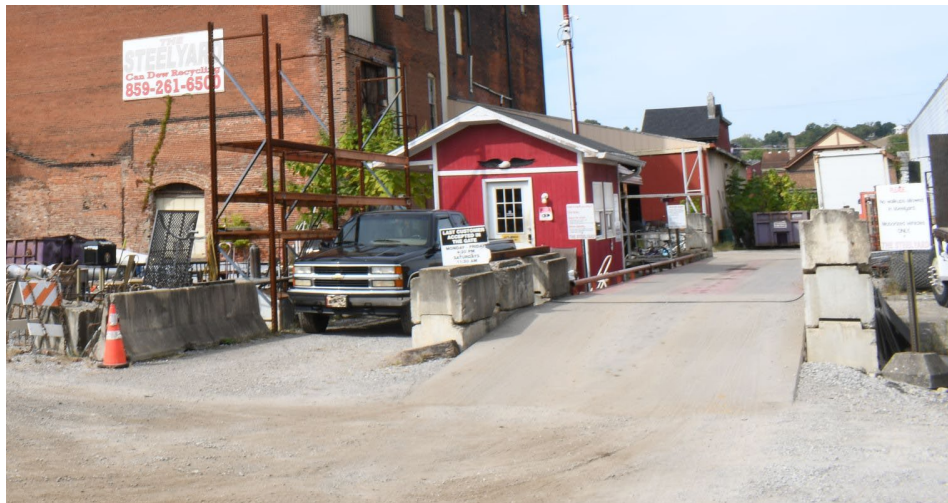
Figure 27 Non-contributing shed/office in steelyard, looking southwest.
