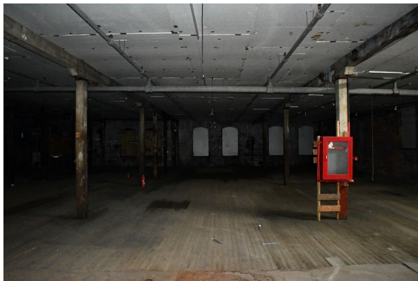
Figure 25 Fourth floor, note wooden posts more narrow than lower floors. (0019)
