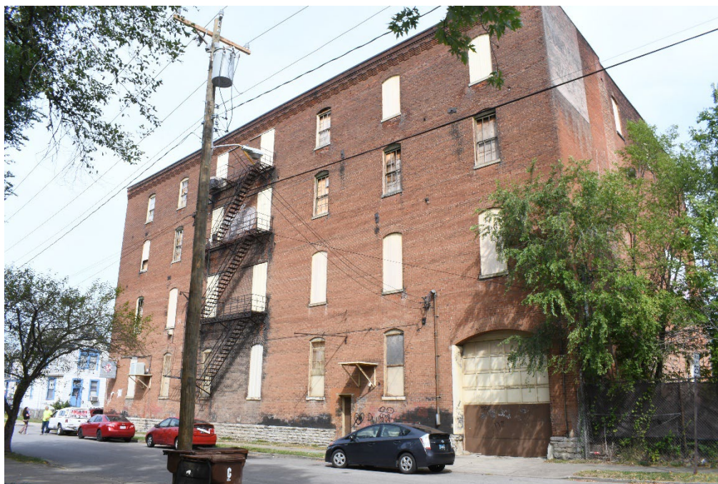
Figure 10 South elevation of Overman Schrader Cordage Company Building, looking NW. (0004)
