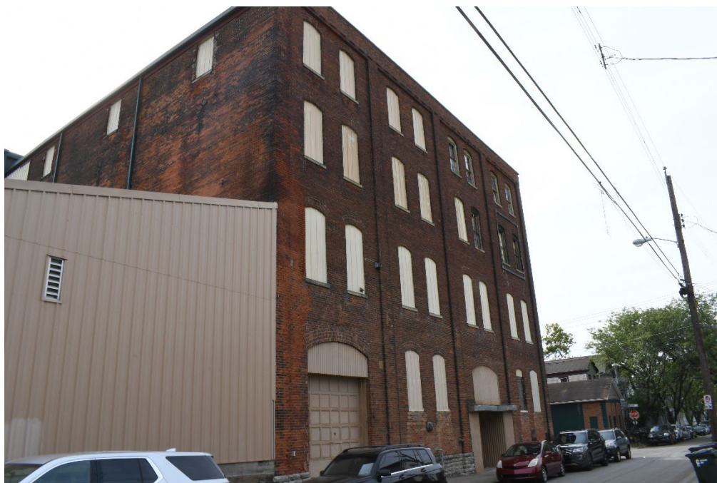
Figure 9 West elevation of Overman Schrader Cordage Company Building, looking SE, fourth bay of the first story and metal-clad lean-to addition on north elevation. (0003)
