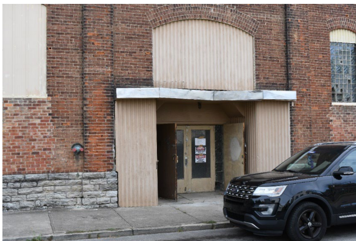
Figure 8 West elevation of Overman Schrader Cordage Company Building, looking east, recessed entryway second bay of the first story. (0002)
