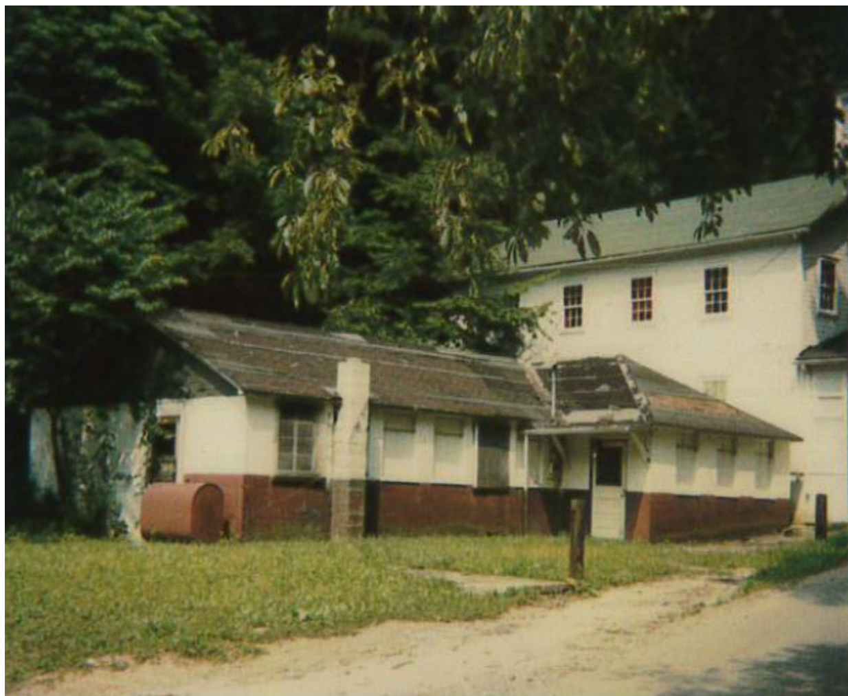
Dunham High School's 1950 addition. Letcher County PVA, photo date unknown Photo from Letcher County PVA's property card. Building in back is Mt. Olive Baptist Church
