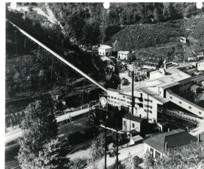
Tipple in Dunham (roof of #207 school pictured in bottom right)
