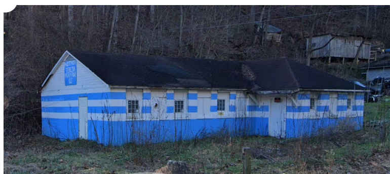
South and East sides of building
