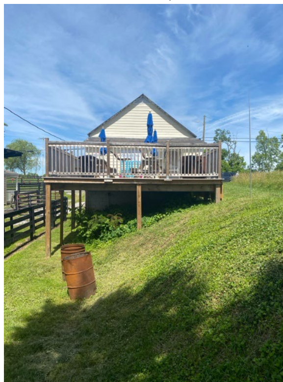
Back of store, camera facing Northwest
