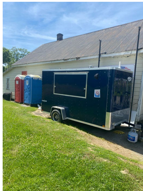
North Side of store
