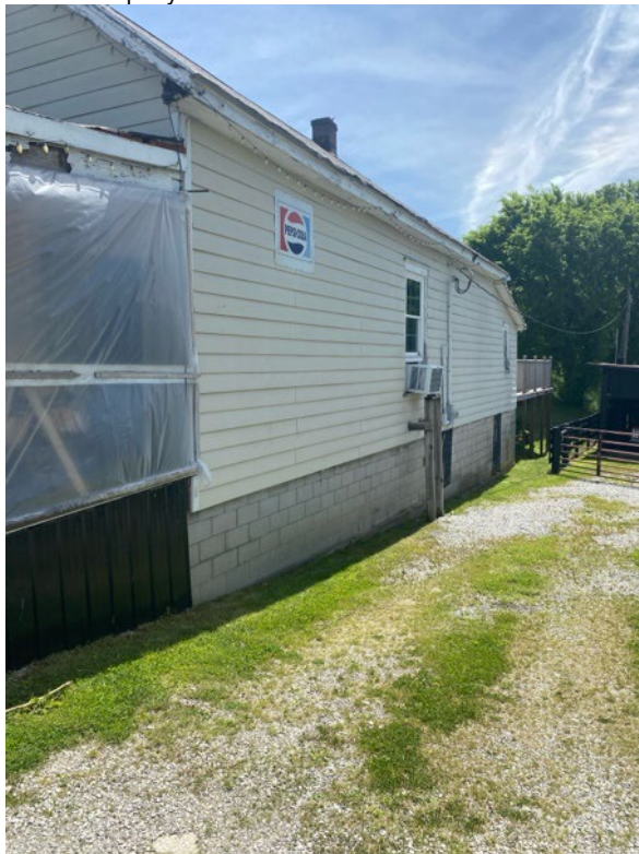
South Side of store, camera facing East
