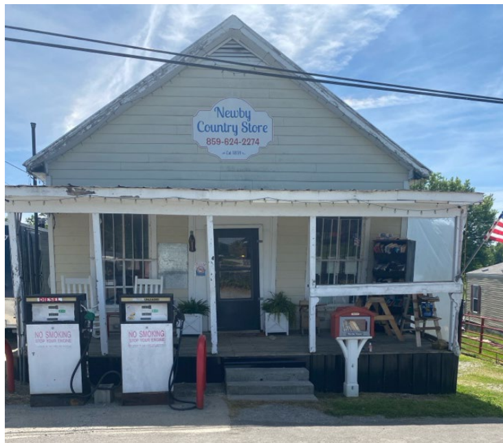
Front of store, camera facing Southeast
