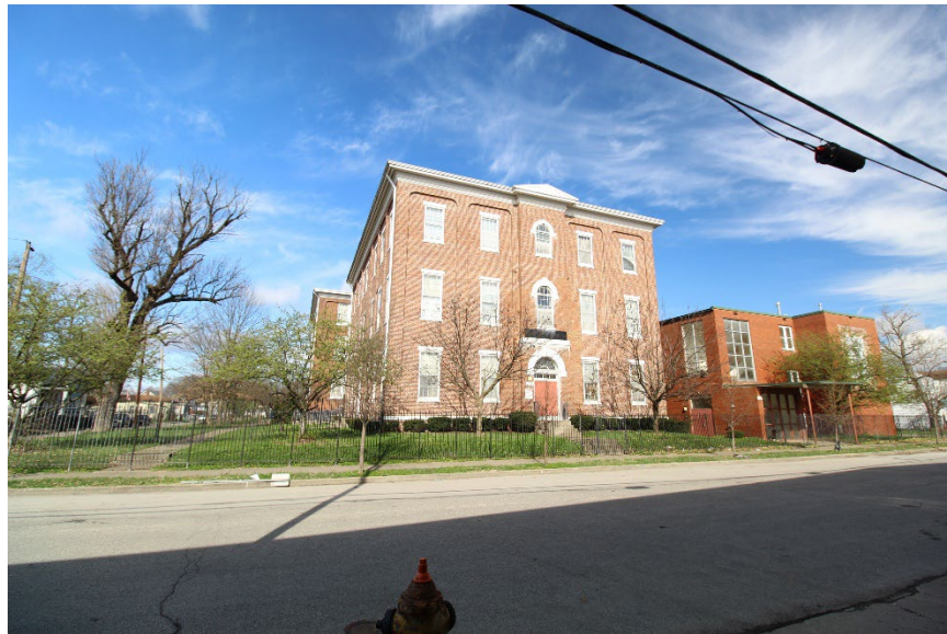
Theodore Roosevelt Elementary School (1866) in Jefferson County. NR #82002719 showing a 1915 addition in the background and a 1954 new building built next to it to serve the school's growing needs.
