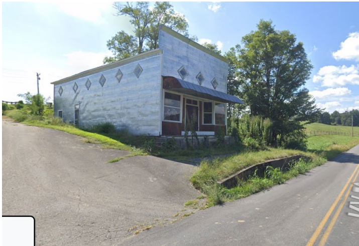
Smith General Store, view to west, prior to collision
