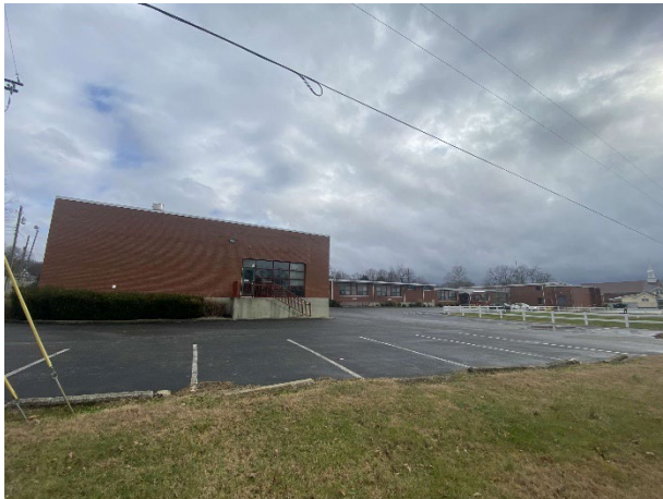
Photo 4, school facing southeast
