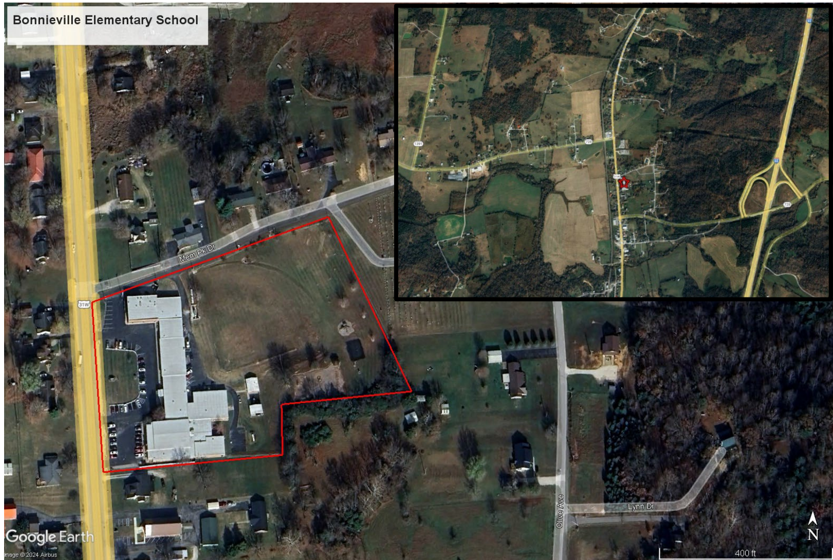
Figure 1. Boundaries of Bonnieville Elementary School, as shown on an aerial map (Google Earth). Location relative to the rest of Bonnieville and I-65 can be seen in the insert corner callout
