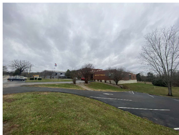
Photo 2, school facing southwest
