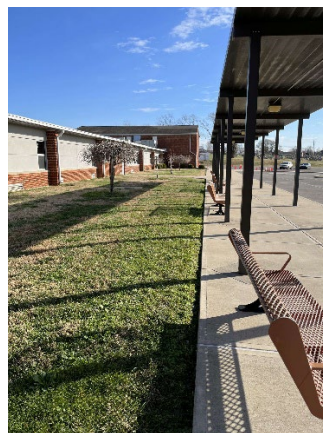
Photo 5, walkway and east wing
