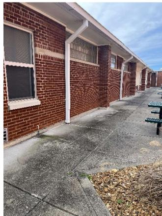
Photo 8, brick wall and glass block window
