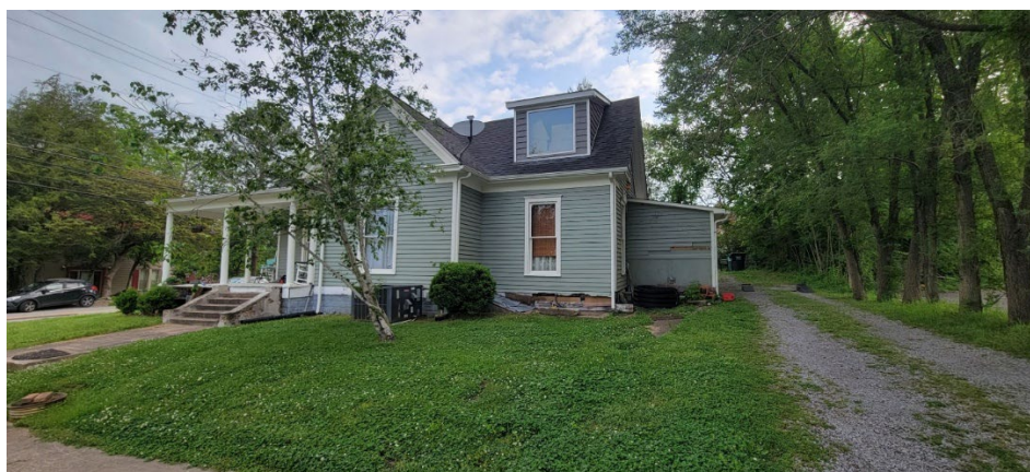
Southwest side of the building – view 2
