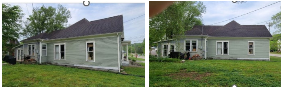
Two views of the Southwest side of the building
