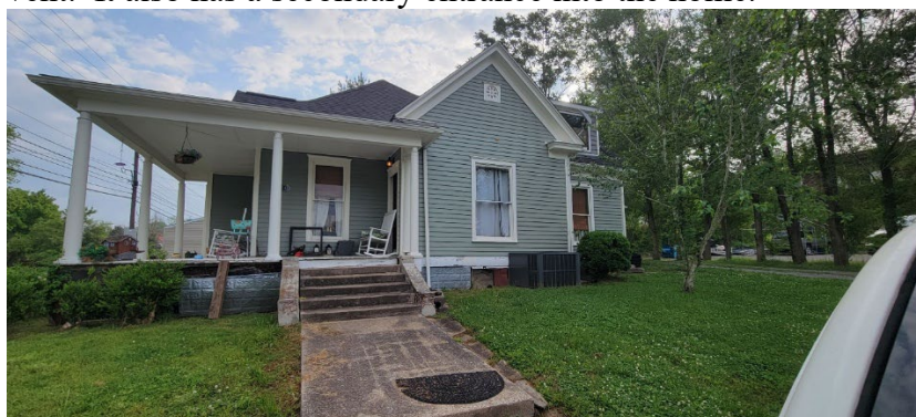
Southwest side of the building
