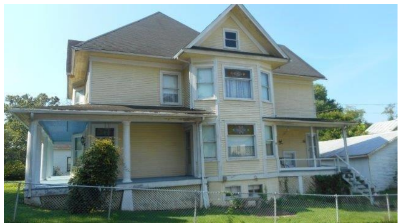
North façade, along 3 rd Street
