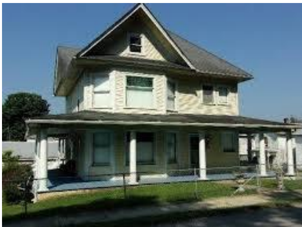
East (front) façade on Main St.
