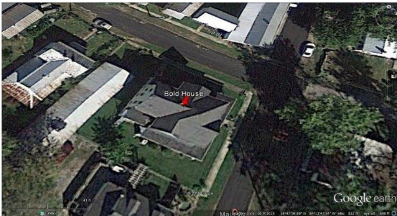
Bold House, 98 Main Street, Foster, Bracken County, Kentucky Longitude: 84° 12' 47.54" W Latitude 38° 47' 59.80" N
