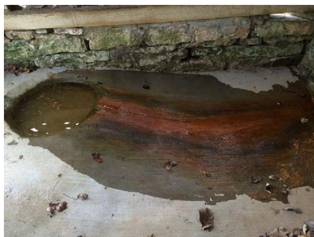
Interior of Frame Springhouse
