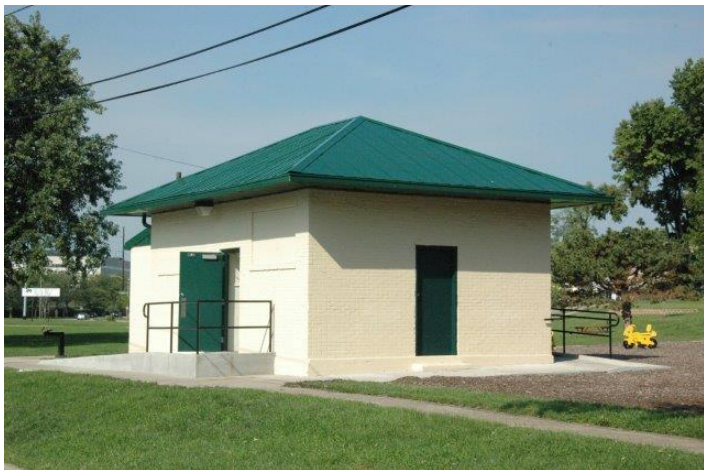
Photo 14: Restroom: view to west
