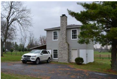
Former Garage/Home Office
