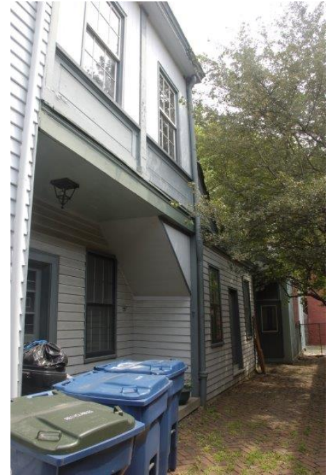
Photo 2: South façade's recessed area
