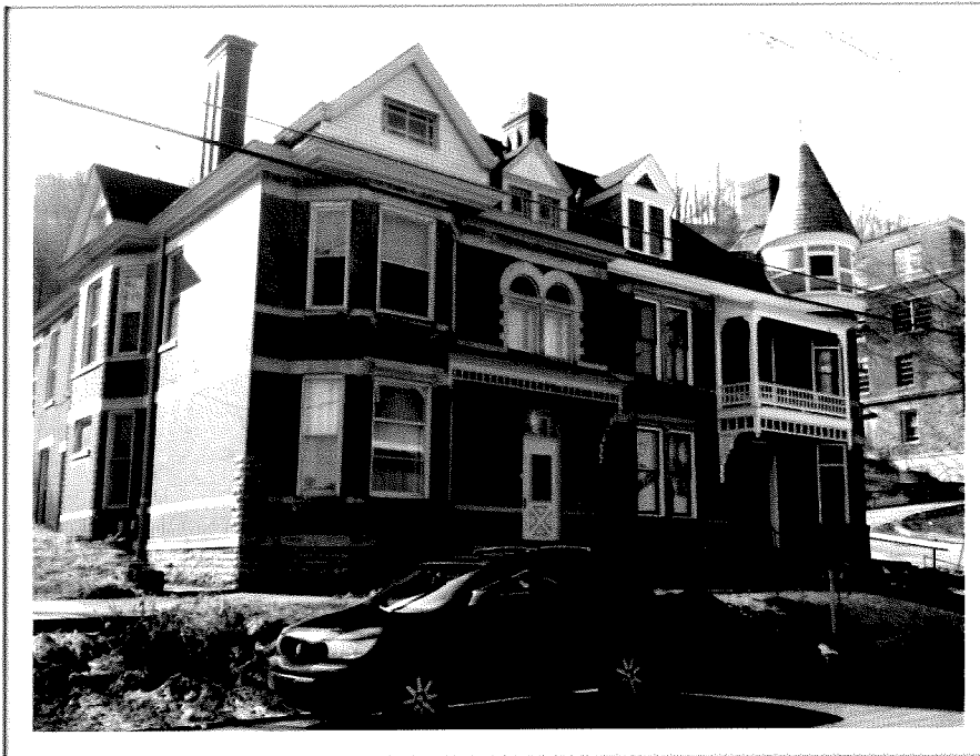
Photo 11 (Above) The Watson Duplex, MS-M-157. Mason County, Ky. East Fourth Street Facade Looking SSE
