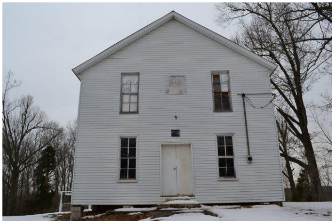
Photo 1: front (southeast) façade
