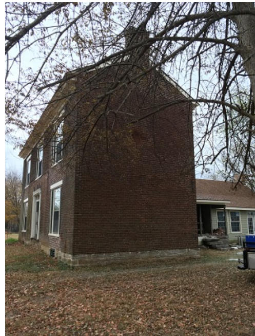
Greek Revival Addition, South façade
