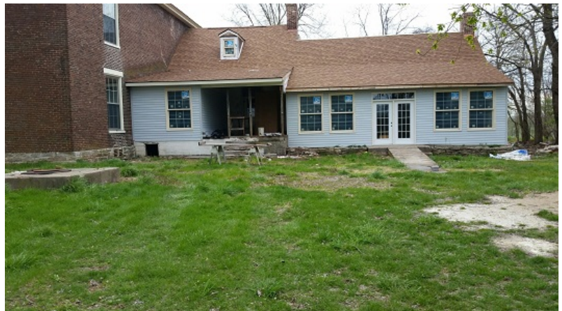
Rear Addition, South façade
