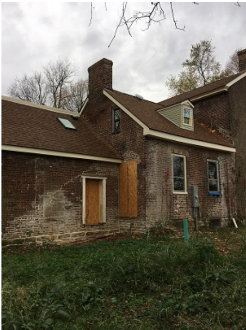
Rear Addition and Original Dwelling, North Façade
