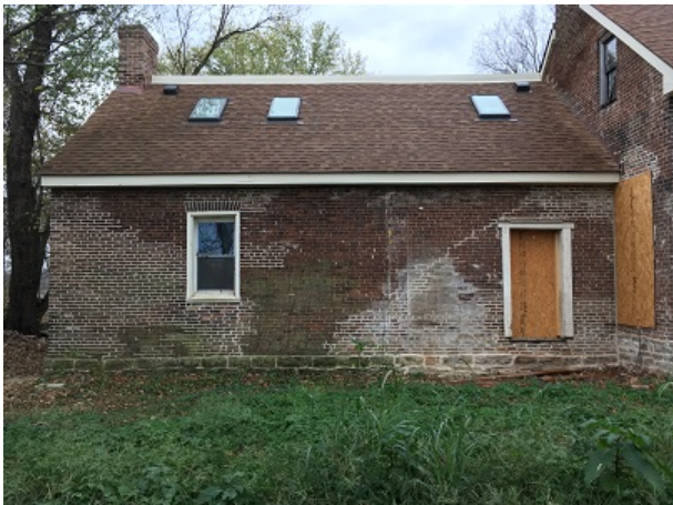
Rear Addition, North façade
