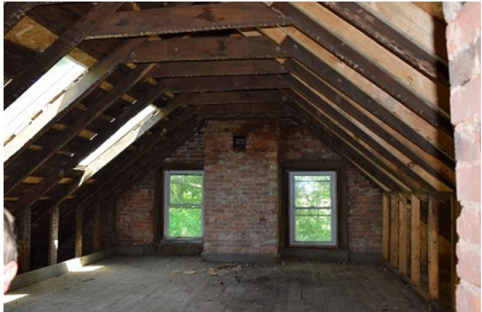
Rear Addition, Second Floor
