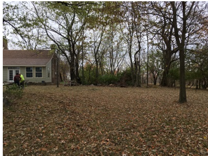
Photo 4 - Craig-Peak House - Ruins of Detached Structure
