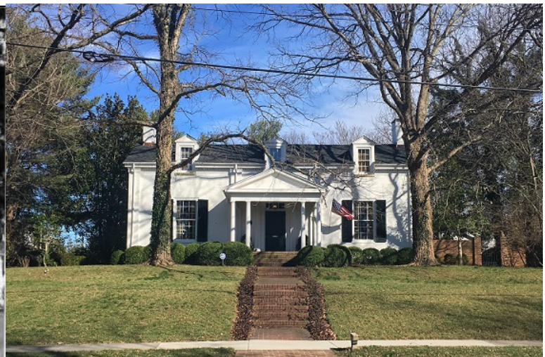
Lyon House, Georgetown, Scott County, Kentucky
