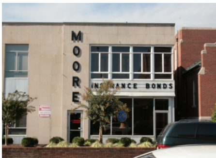
Charles M. Moore Building (1953) Photo 11
