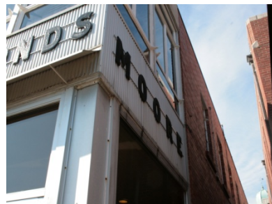
Right Exterior Wall (photo 6)
