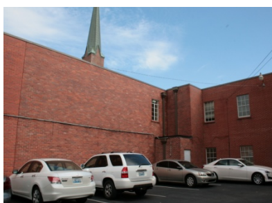
Back of the Building Photo 7
