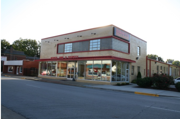
Gallaway Farm Equipment Building (1948)
