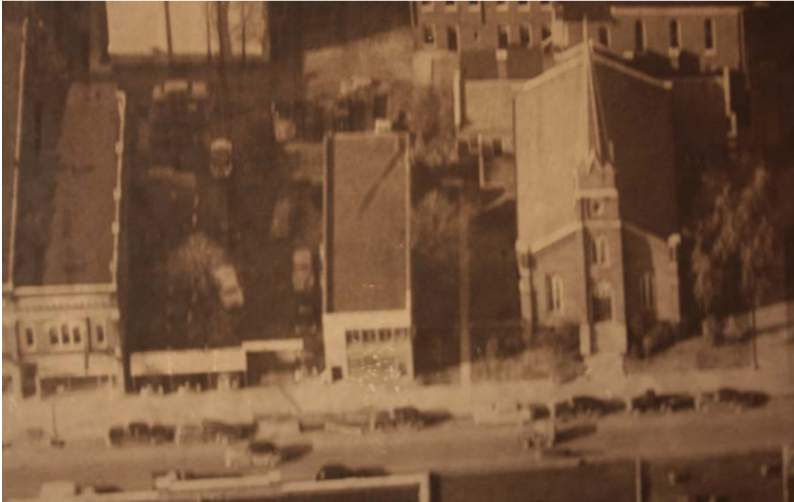
Charles M. Moore Insurance Company building, ca. 1960, center of image. Note the cars parking along the west of the building. The 1972 addition now occupies that parking area. (Photo 1)
