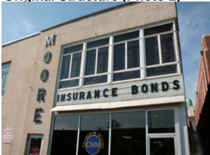
Original Structure (Photo 2)
