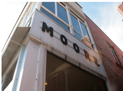
Right Exterior Wall (photo 5)
