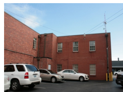
Back of the Building Photo 9
