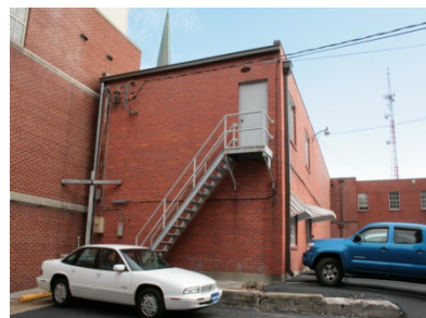
Back of the Building Photo 8
