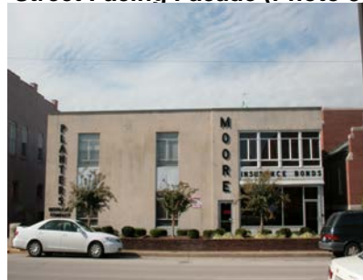
Street Facing Facade (Photo 3)
