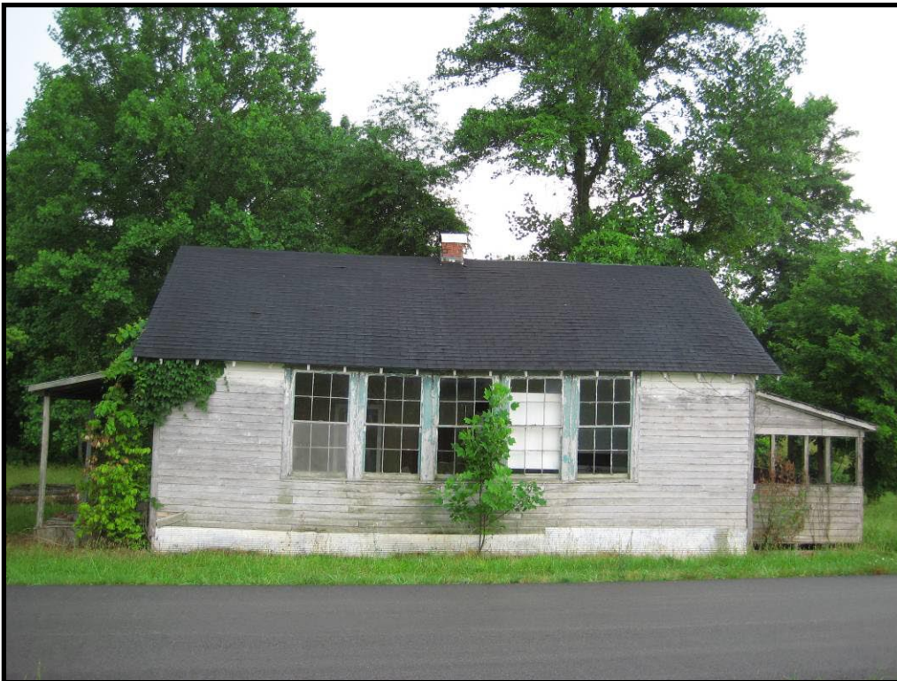
Figure 27 Caney Fork School, CS-138, a one-room school in the Liberty quad.
