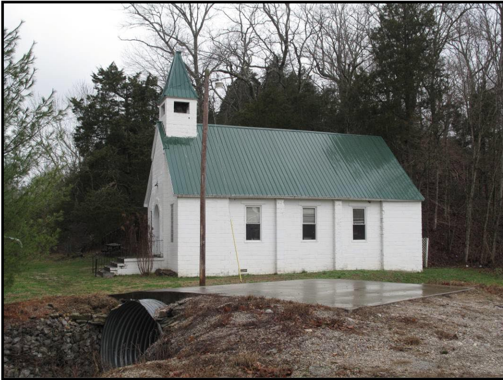
Figure 38 Frey Creek Church, CS-52, Ellisburg quad.
