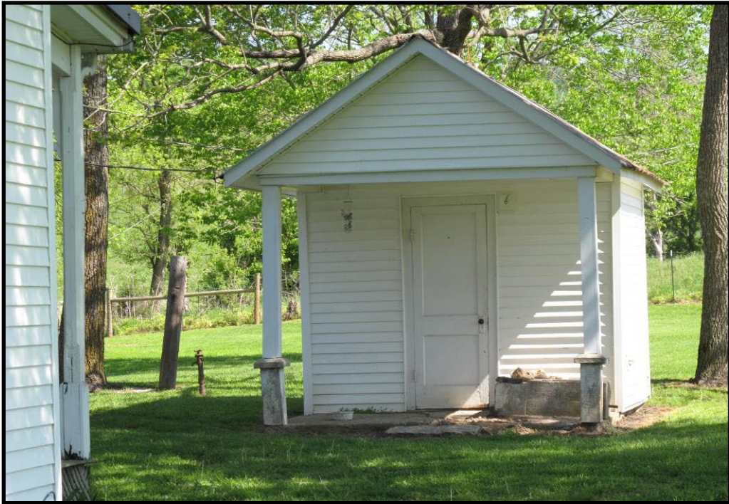
Figure 141 Well/pump house at CS-80, Ellisburg quad.
