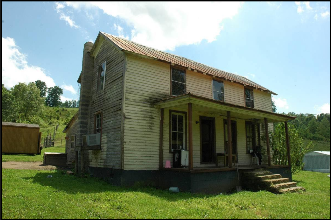
Figure 113 CS-141, a one-and-one-half story Cumberland on Poplar Hill Road, Yosemite quad.
