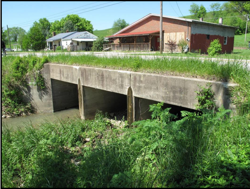
Figure 79 CS-81, a WPA-era culvert (1935) in the Ellisburg quad.
