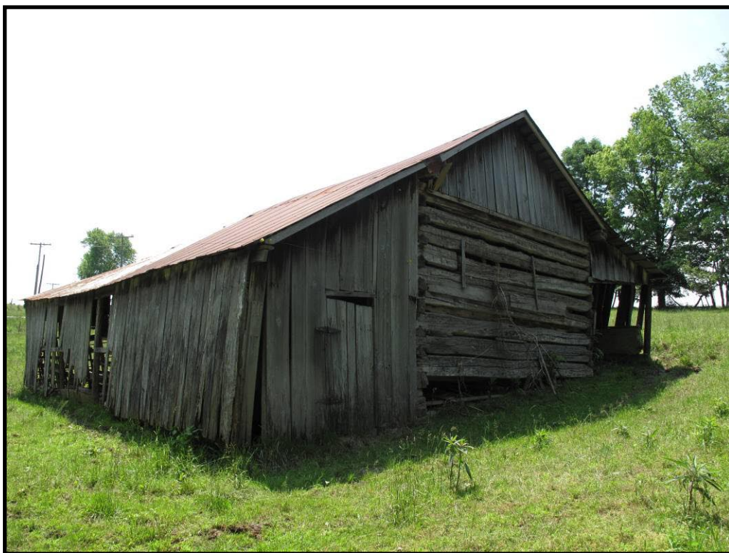
Figure 174 Log crib barn, CS-101, Mintonville quad.
