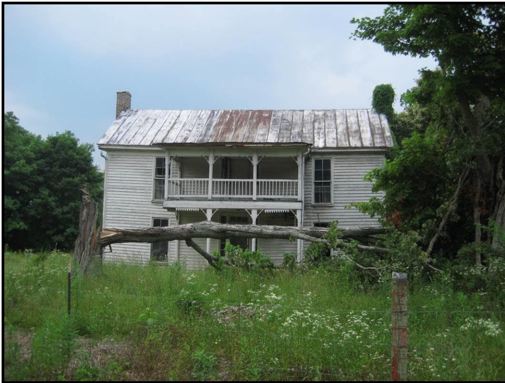
Figure 95 The Reynolds House, CS-134, a central passage in the Liberty quad.
