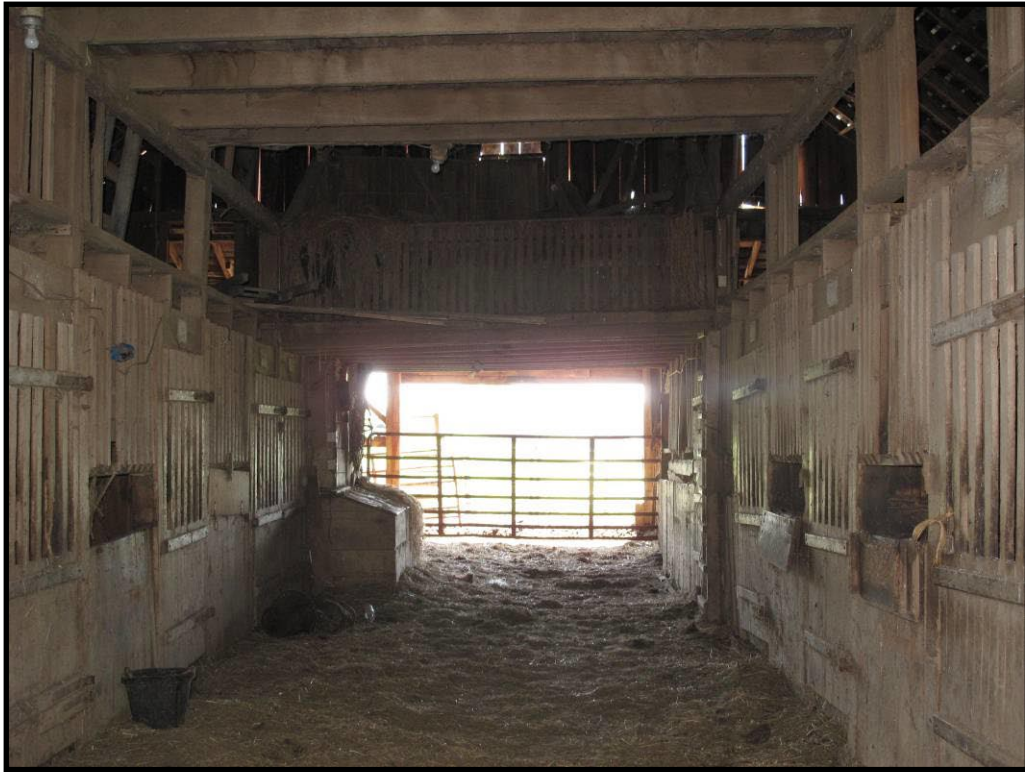
Figure 166 Interior of barn at CS-80, facing east.
