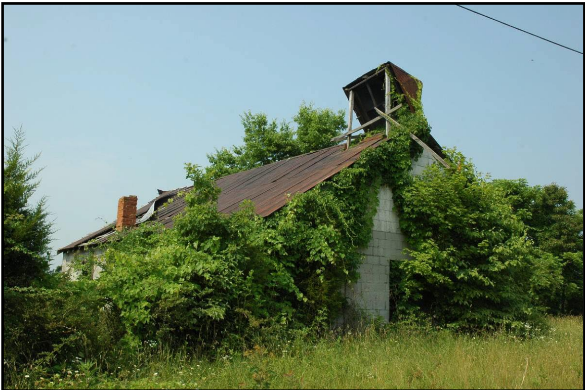
Figure 51 Church on Patsy Riffe Road, CS-127, Hustonville quad.
