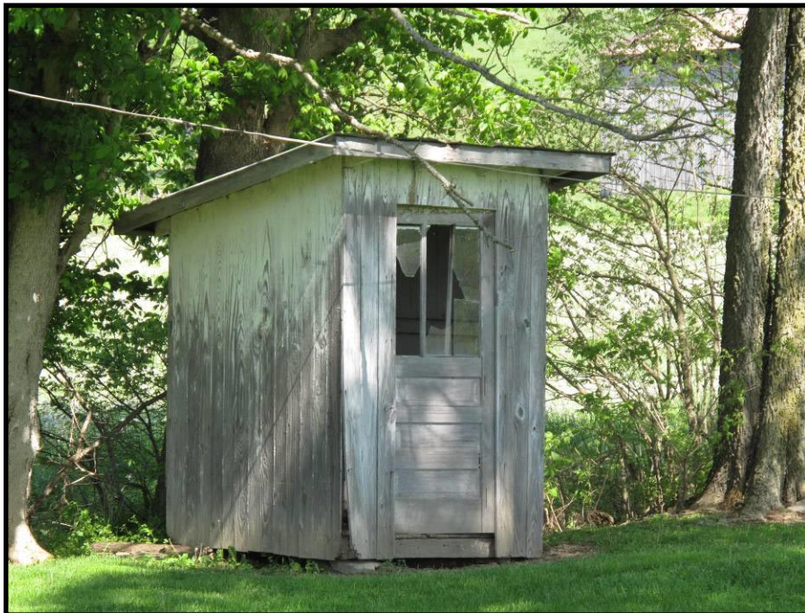
Figure 158 Privy at CS-80, Ellisburg quad.
