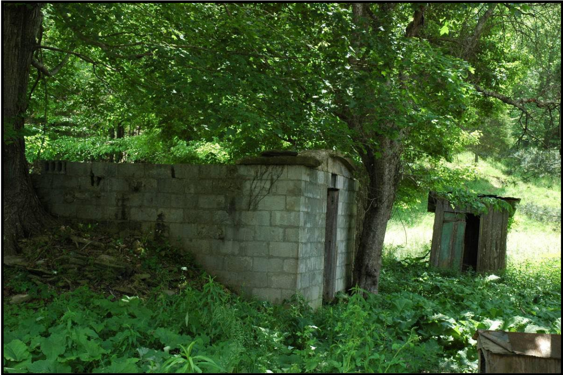
Figure 156 Concrete block root cellar at CS-115 on Upper Brush Creek Road, Ellisburg quad.
