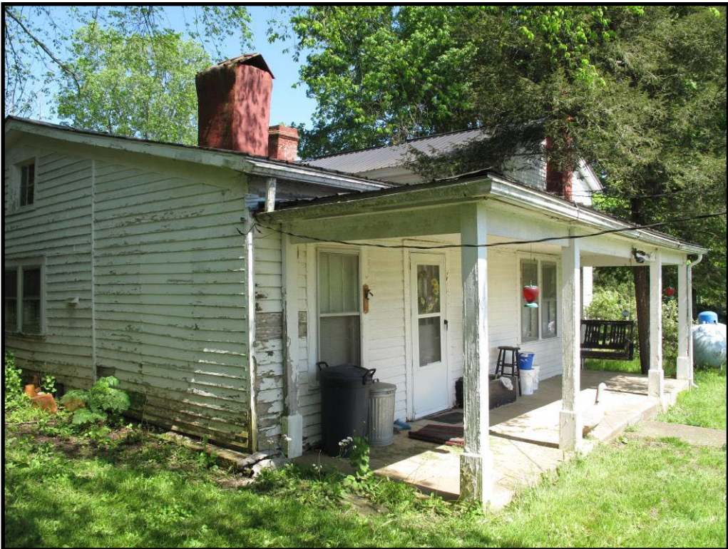
Figure 127 Detail of the rear ell of CS-90.
