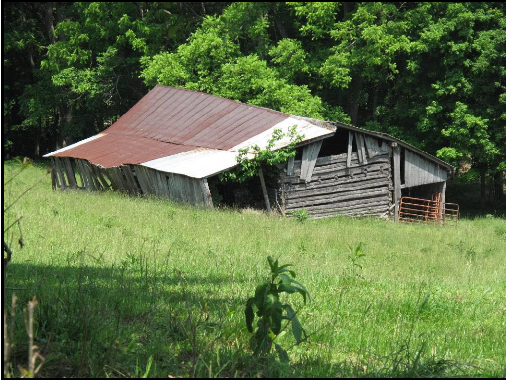
Figure 175 Log crib barn, CS-101, Mintonville quad.
