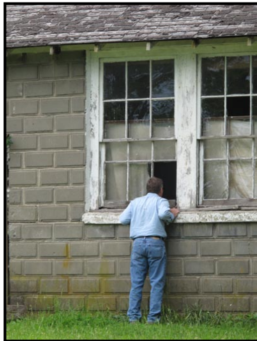
Ned Crankshaw examines the interior of a historic rural school.
