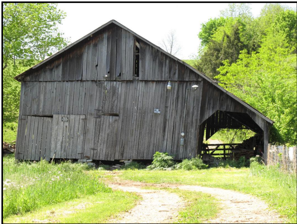
Figure 167 Stock barn at CS-90, Ellisburg quad.
