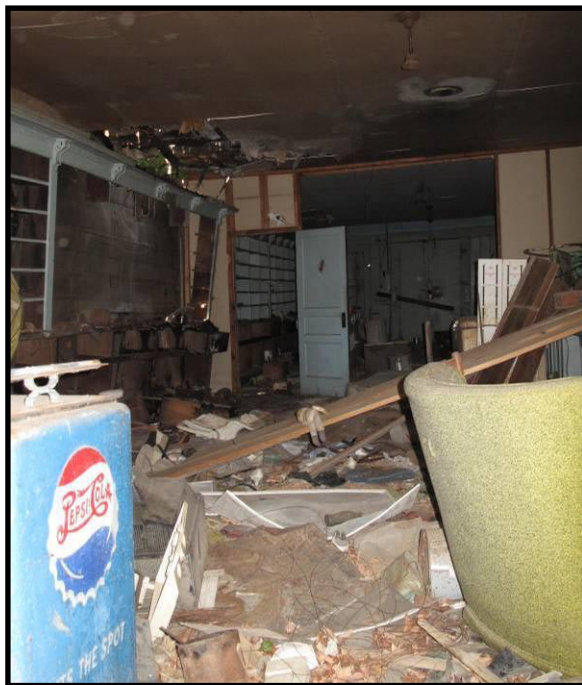
Figure 73 Interior of the Powers/Peyton's Store, CS-84.
