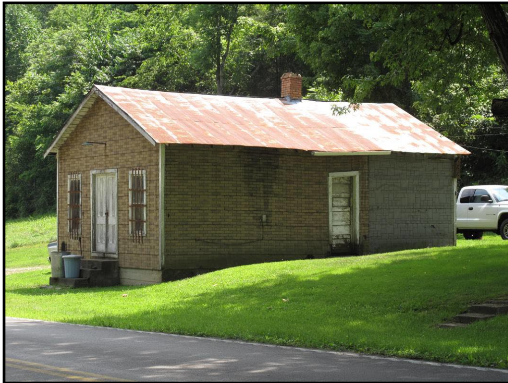
Figure 69 Store along Route 49, CS-166, Liberty quad.
