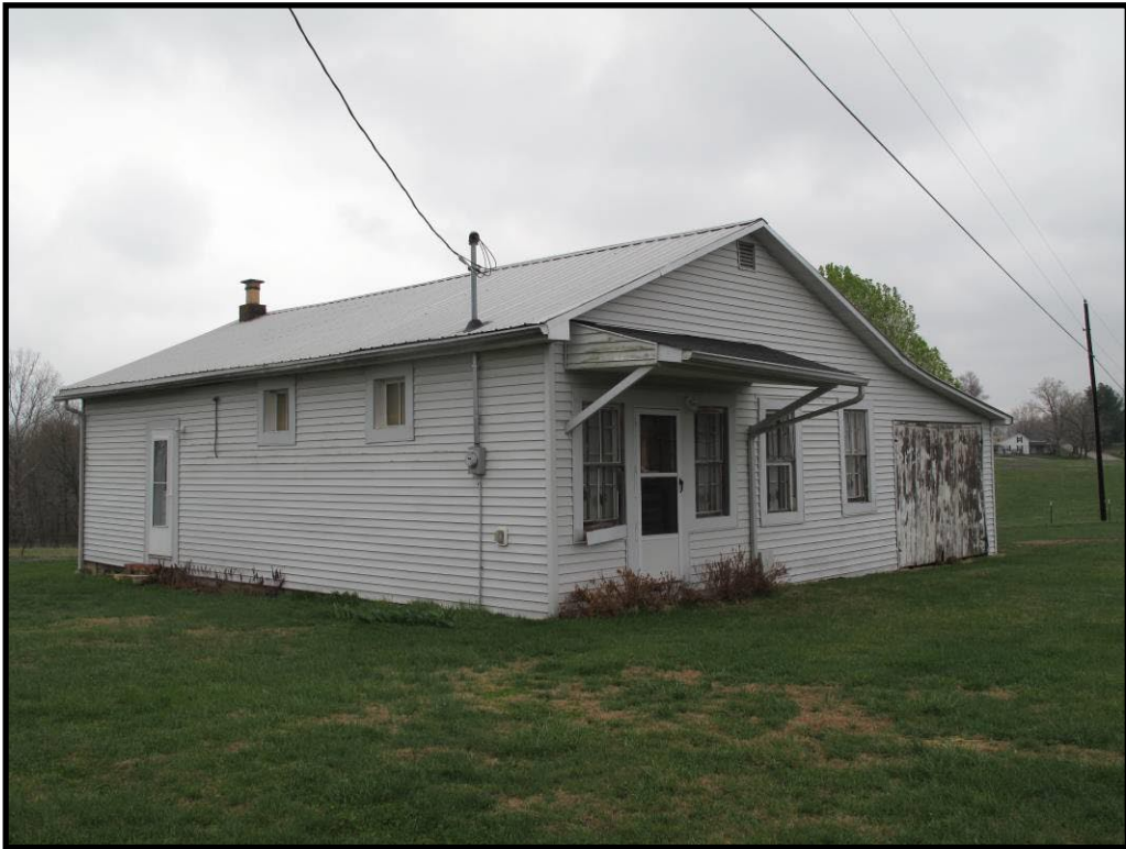
Figure 57 Campbell Store, CS-71, in the Clementsville quad.
