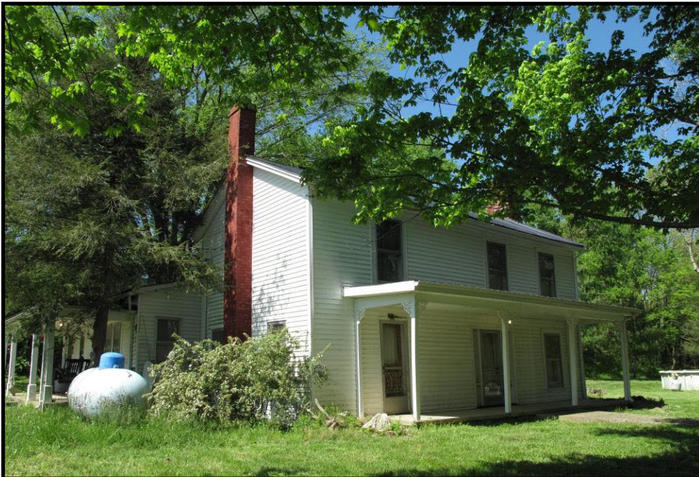
Figure 125 George Wilson Ellis House, CS-90, in the Ellisburg quad.
