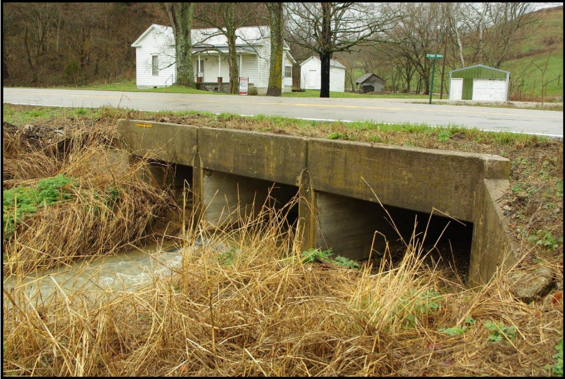
Figure 80 CS-87, a WPA-era culvert (1935) in the Ellisburg quad.
