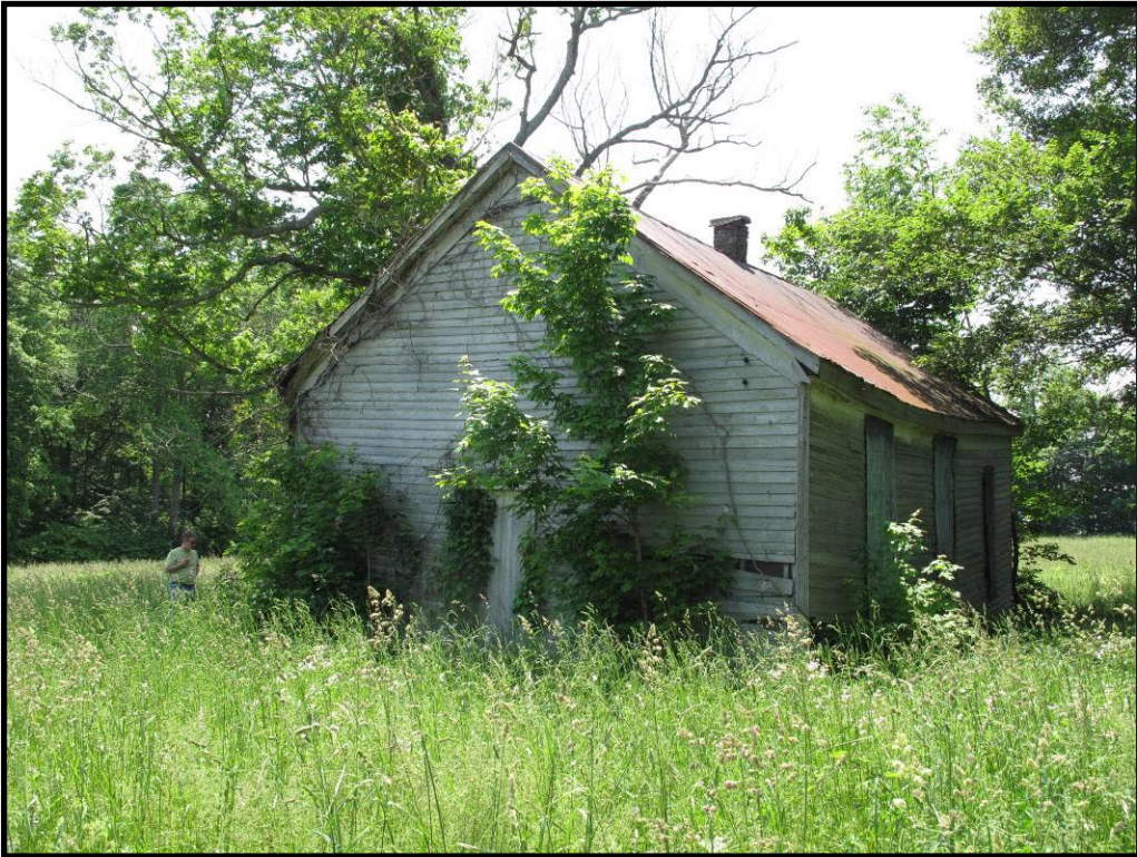
Figure 24 Woods School, CS-102, a one-room school in the Mintonville quad.
