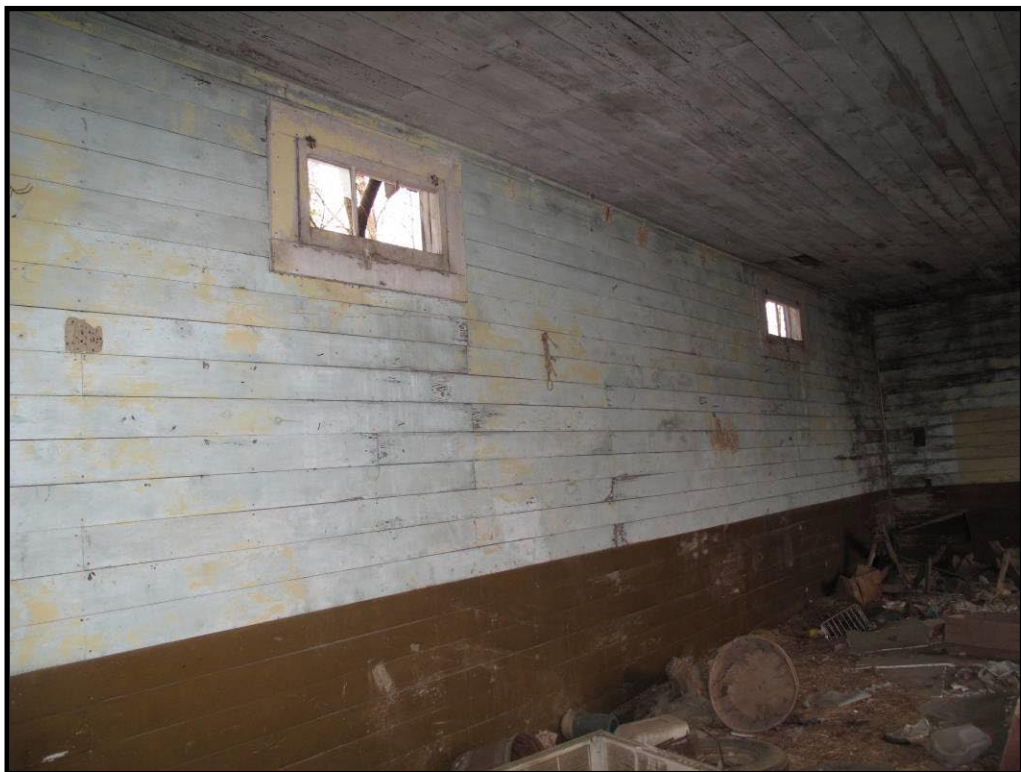
Figure 15 Detail of the transom windows in the Allen School (CS-74).
