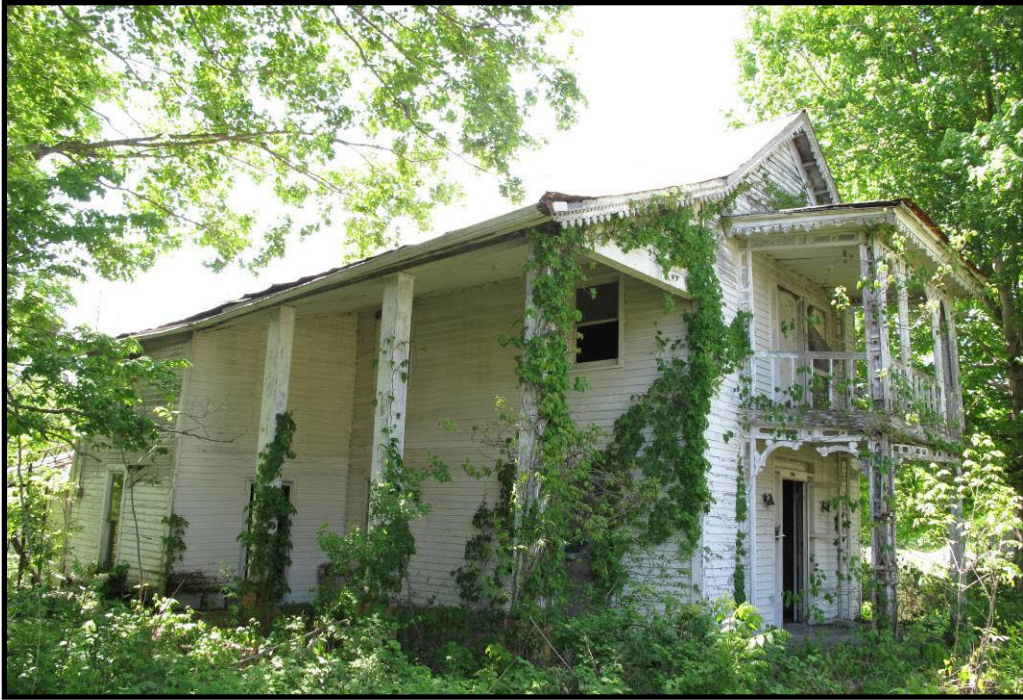
Figure 133 View of side porch of CS-85.
