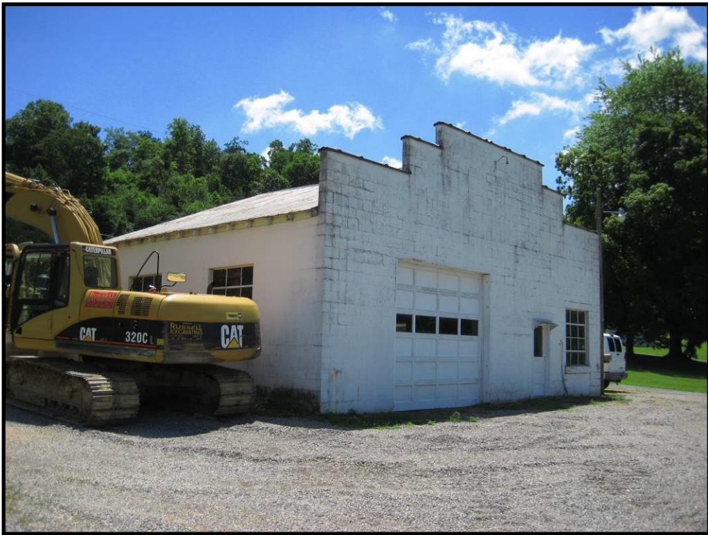
Figure 84 CS-151, a former Texaco Station on Route 910, south of Phil.
