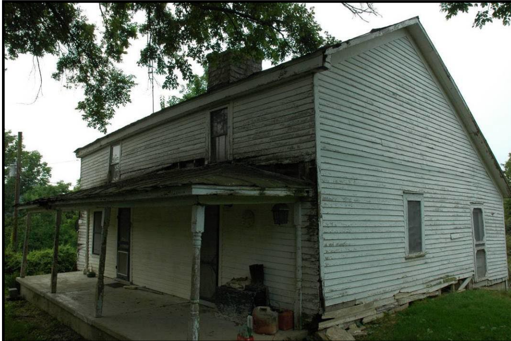
Figure 85 Log (with half-dovetail notching) and frame house, CS-132, on Route 78 in the Ellisburg quad.
