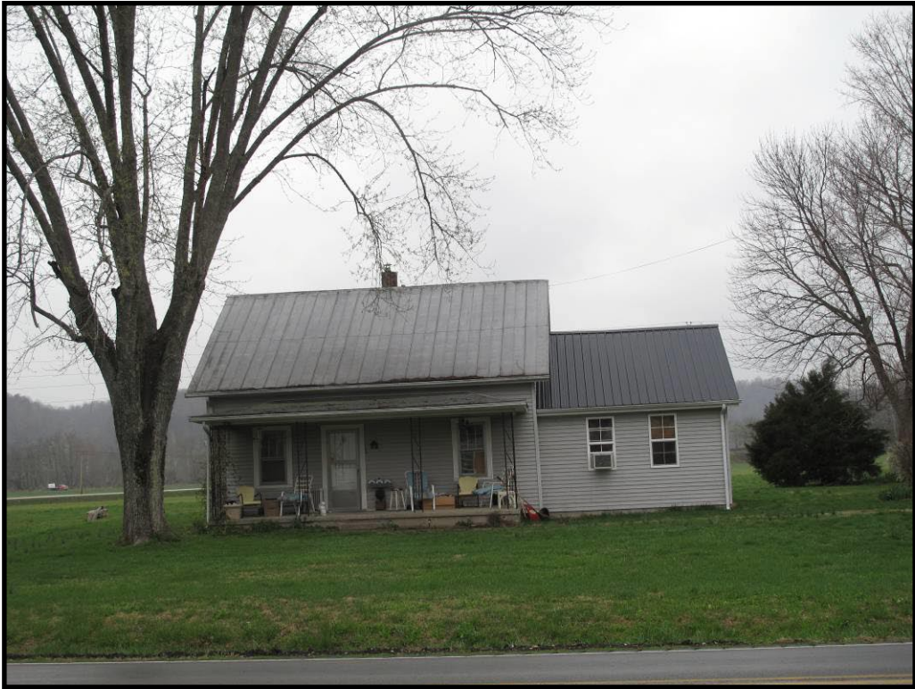
Figure 115 CS-63, a one-story Cumberland in Clementsville with one of its doors removed.
