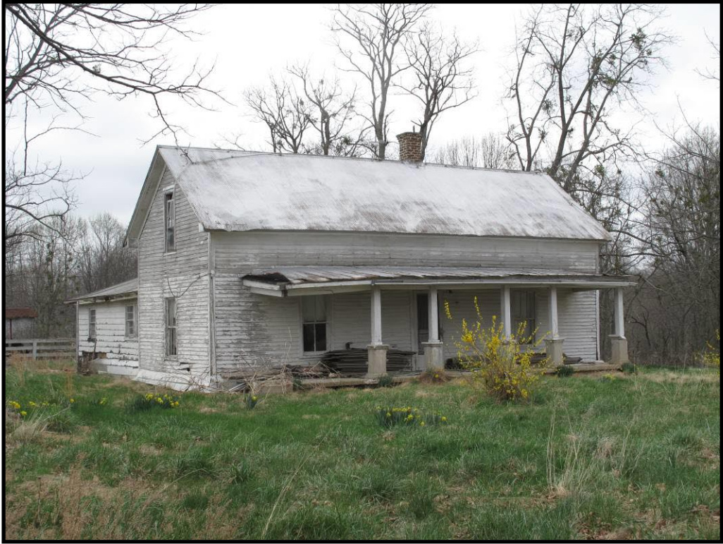
Figure 97 CS-58, a one-story central passage house in the Clementsville quad.
