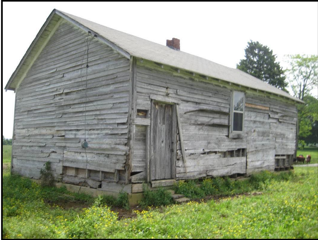
Figure 28 Cantown School, CS-92, a one-room school in the Liberty quad.
