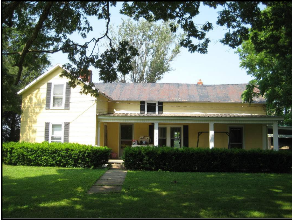
Figure 90 Façade of CS-121, Eubank quad, which appears to be a log saddlebag with a frame front gable addition.
