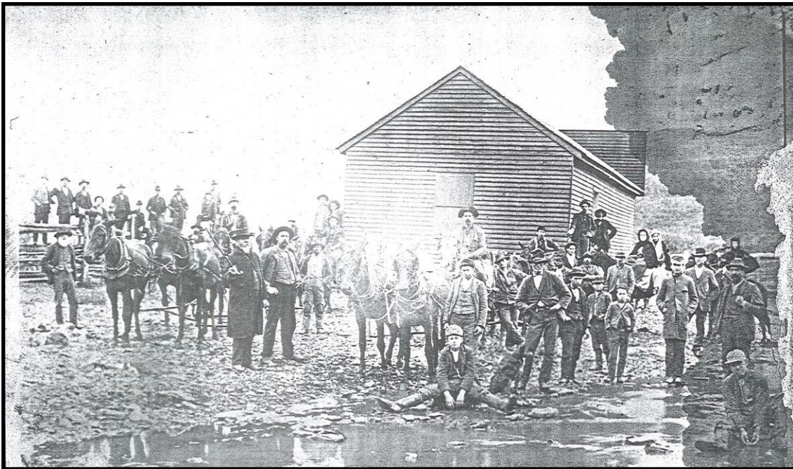
Figure 71 Circa 1880 photo of the rear of the Powers/Peyton's Store, CS-84. 45
