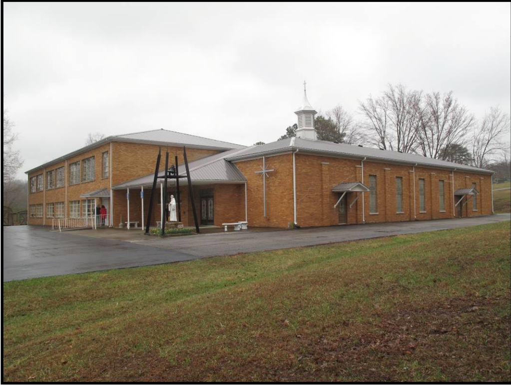
Figure 42 St. Bernard's Church and School, CS-61, in Clementsville.
