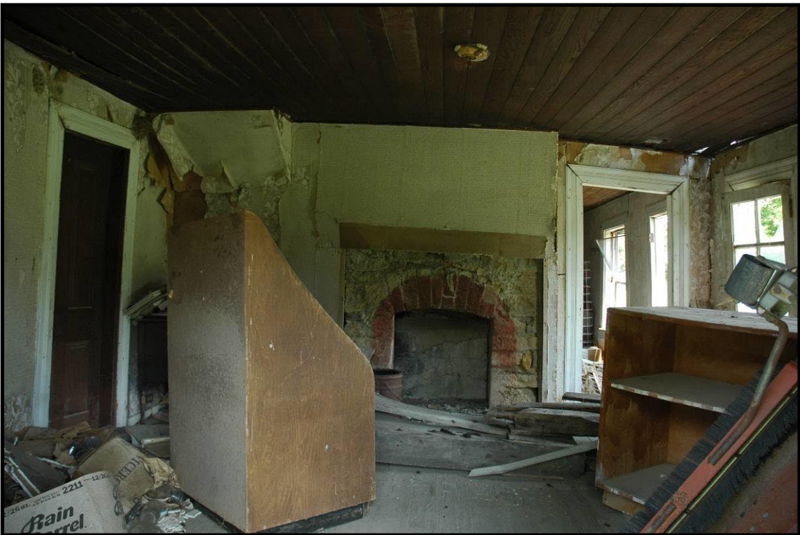
Figure 112 Interior of CS-114 on Brush Creek Road, Ellisburg quad.
