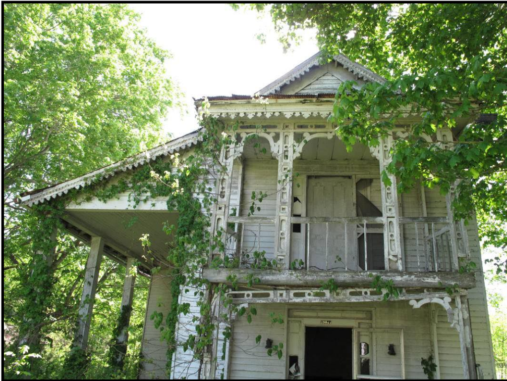
Figure 132 Detail of the porch of CS-85.
