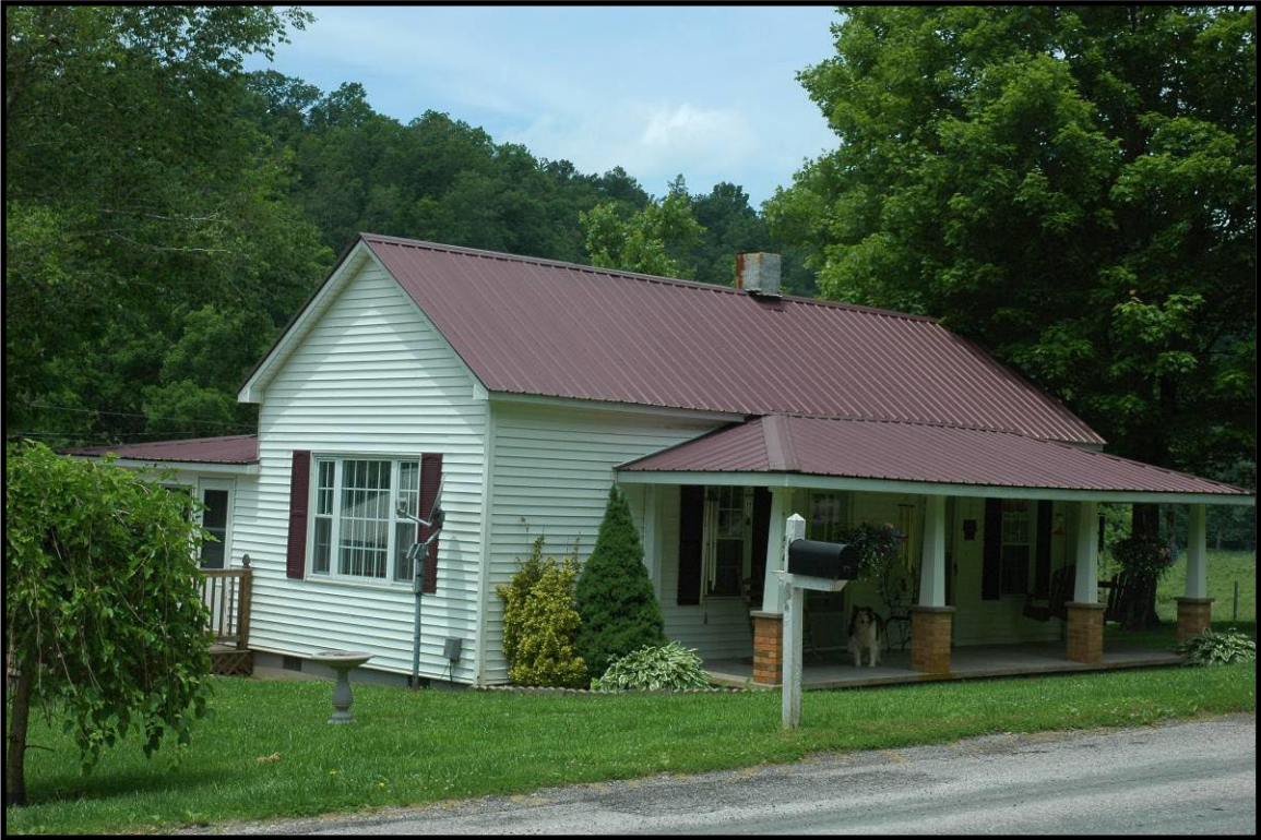
Figure 116 CS-111, 1549 Shucks Creek Road, Ellisburg quad.
