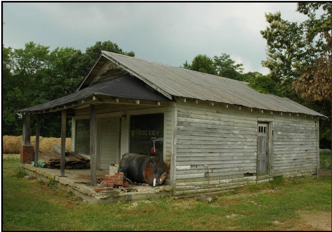
Figure 63 Grocery on Faulkner Road, CS-135, in the Liberty quad.
