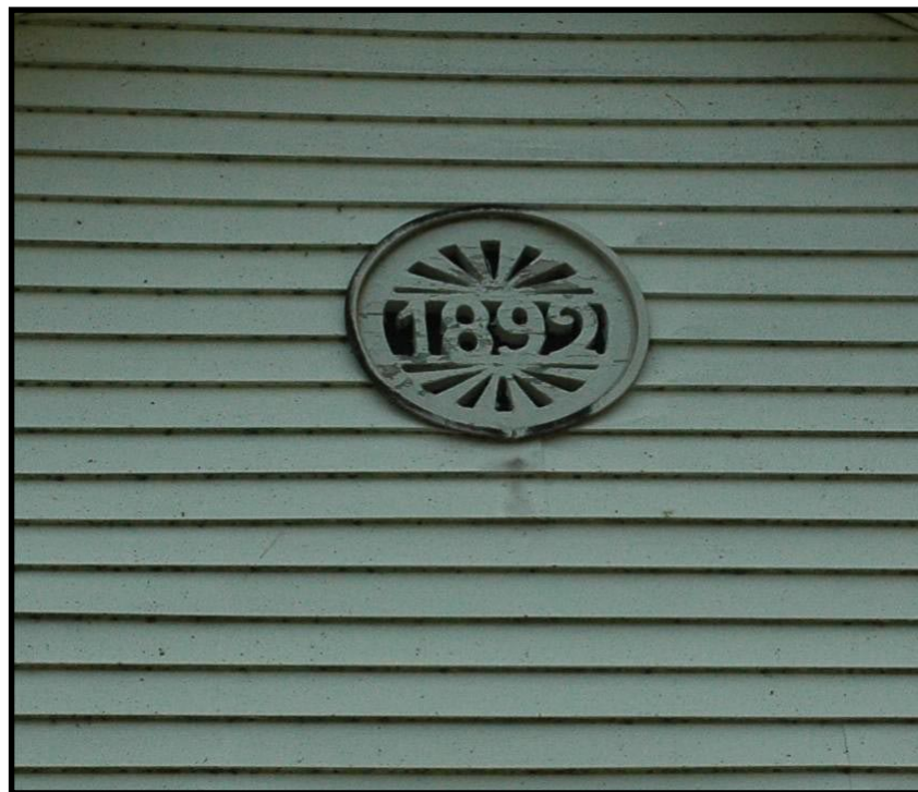
Figure 102 Detail of attic vent on CS-131.
