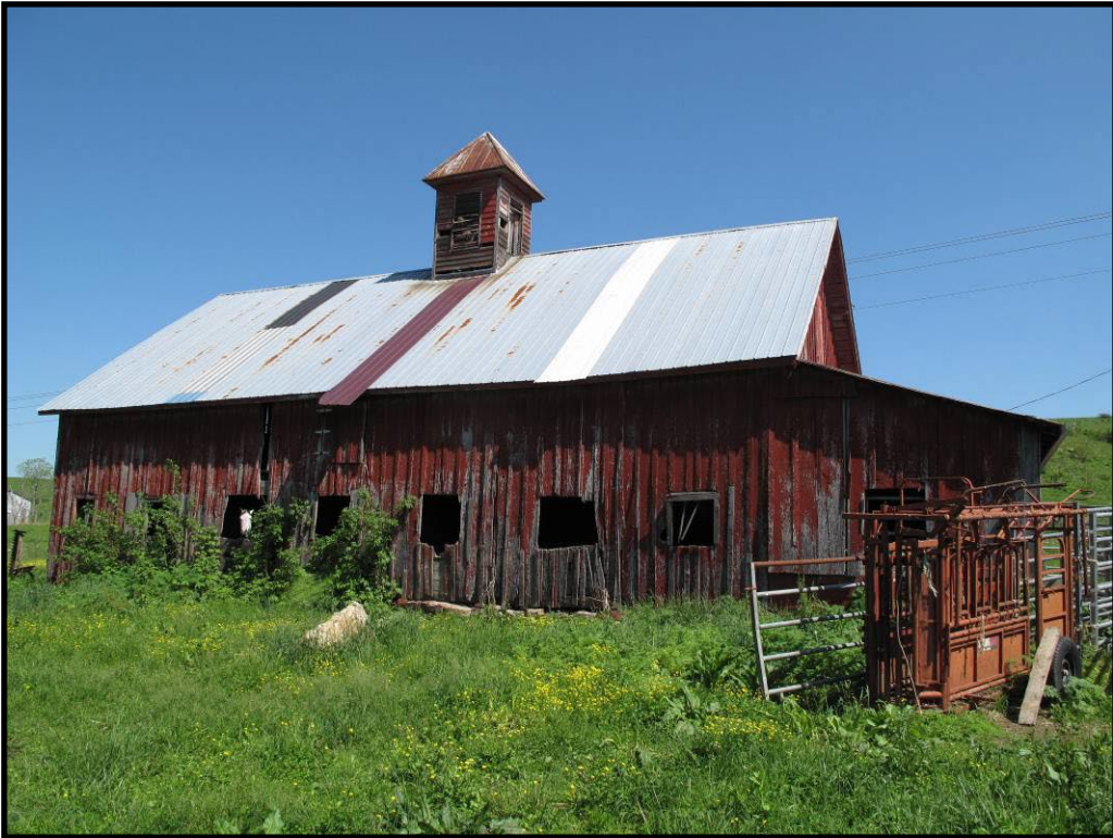
Figure 165 South and east elevations of barn, showing shed addition at east gable end.
