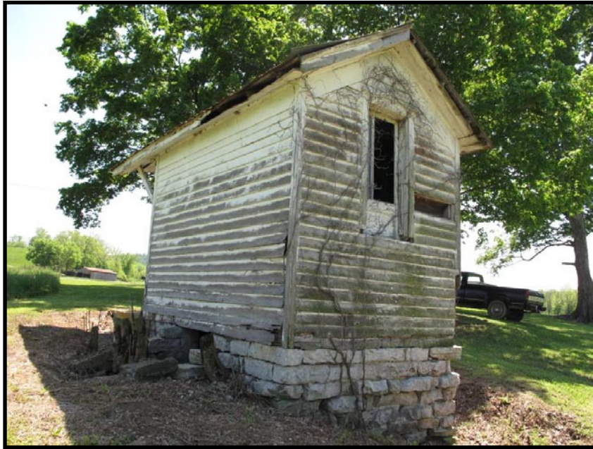
Figure 144 Side entrance to below grade springhouse and rear elevation, CS-10.
