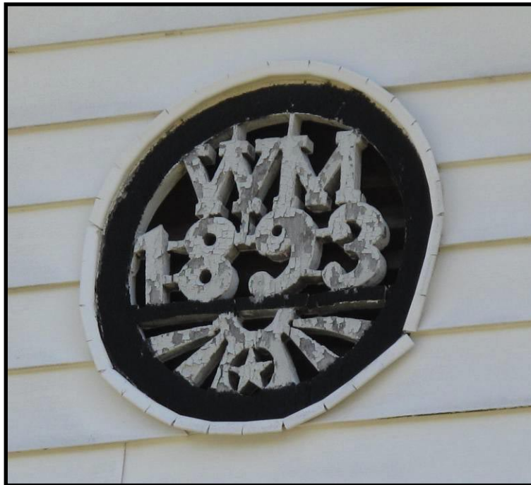
Figure 100 Detail of attic vent on façade.
