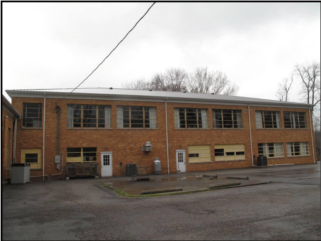
Figure 35 South elevation of St. Bernard's School.
