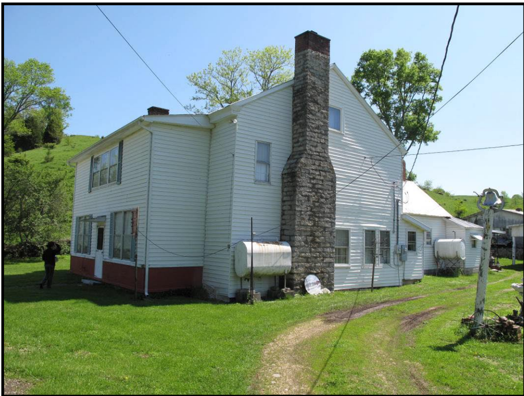
Figure 130 CS-89, facing northeast.
