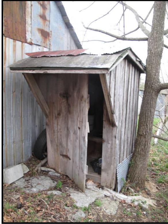
Figure 159 Privy at the Maxey Valley School, CS-57, Hustonville quad.
