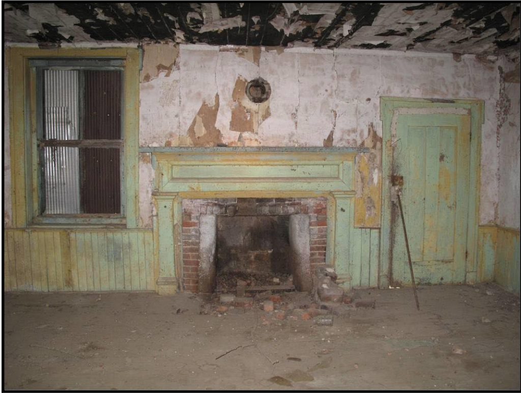
Figure 136 Interior of CS-158.
