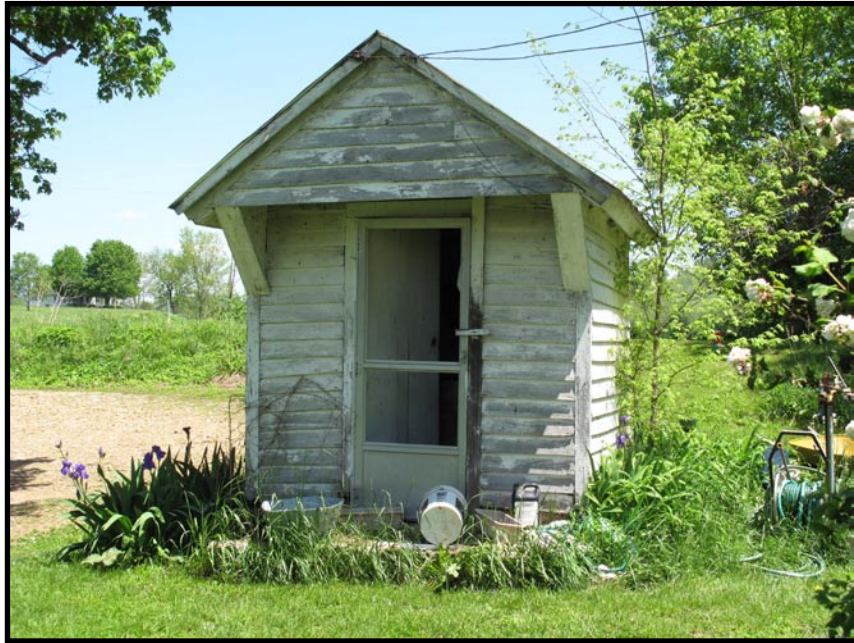
Figure 145 The well-house at CS-82 in the Ellisburg quad.
