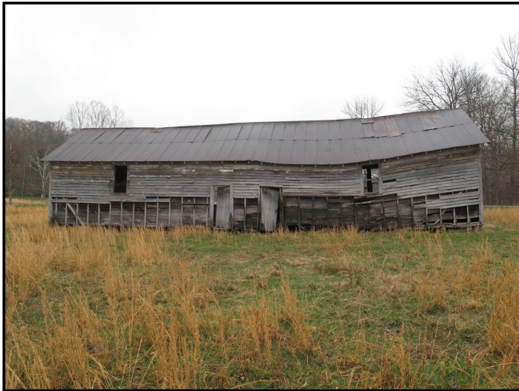
Figure 17 South elevation of the Atterson School.
