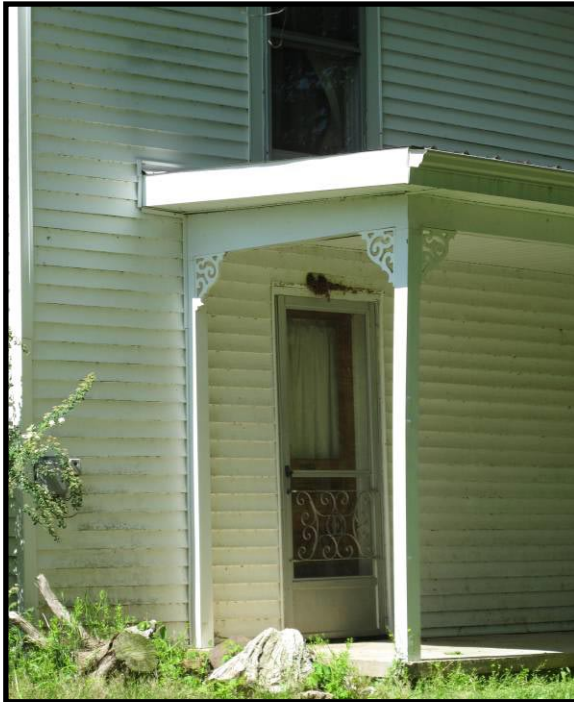
Figure 128 Detail of second door on façade of CS-90.
