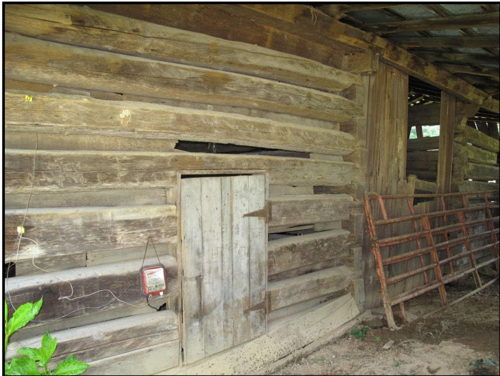
Figure 176 Log crib barn, CS-101, Mintonville quad.
