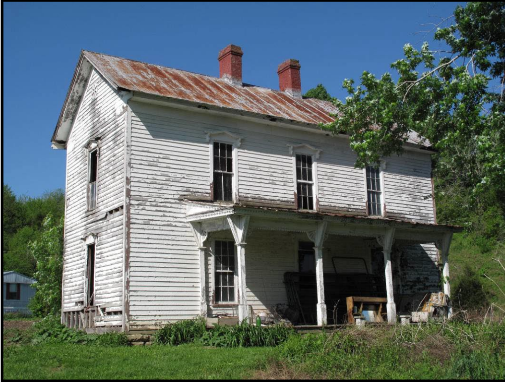
Figure 94 CS-79, a central passage house in the Ellisburg quad.
