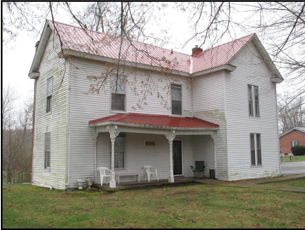
Figure 44 The original rectory at St. Bernard's Church and School, CS-61, in Clementsville.
