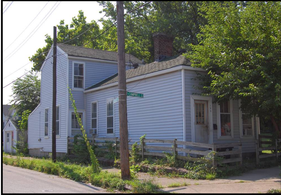
Figure 4. 20 South elevation and façade of 165 Campbell Street (JFCB-113).
