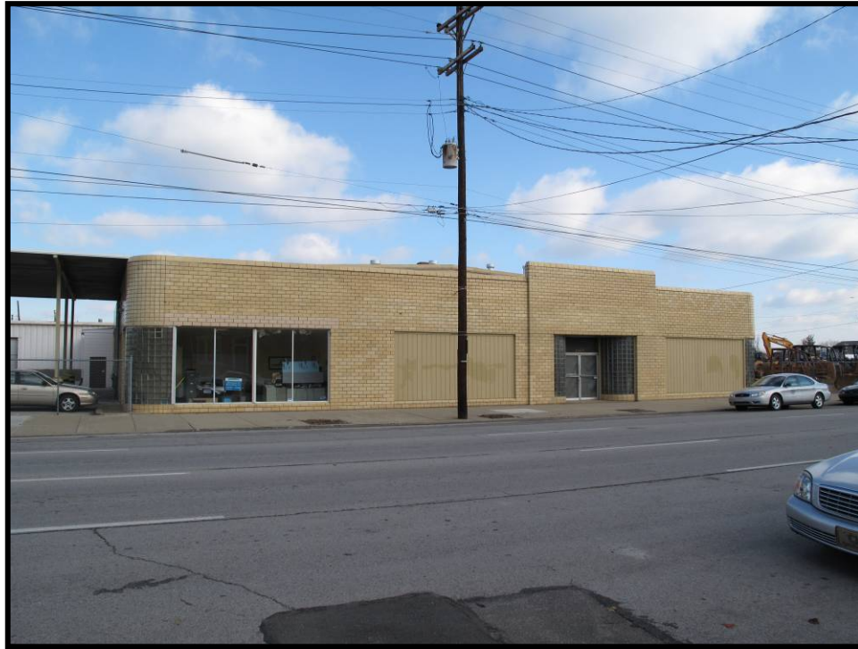
Figure 4. 240 South elevation of 1007 East Jefferson Street (JFCH-1272).
