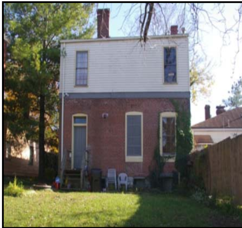
Figure 4. 25 Rear elevation of 1411 Quincy Street, showing frame camelback portion (JFCB-315).
