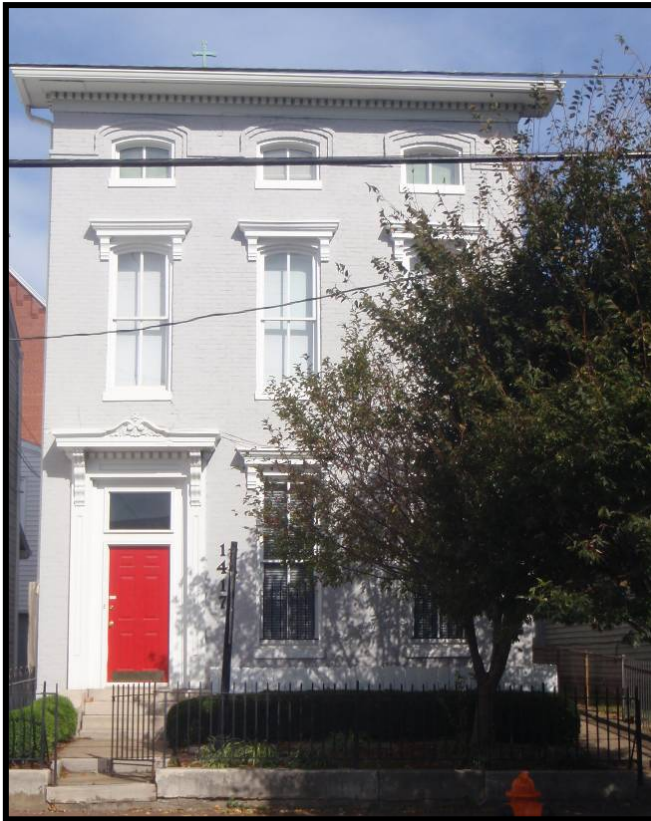
Figure 4. 8 Façade of 1417 Story Avenue (JFCB-352).
