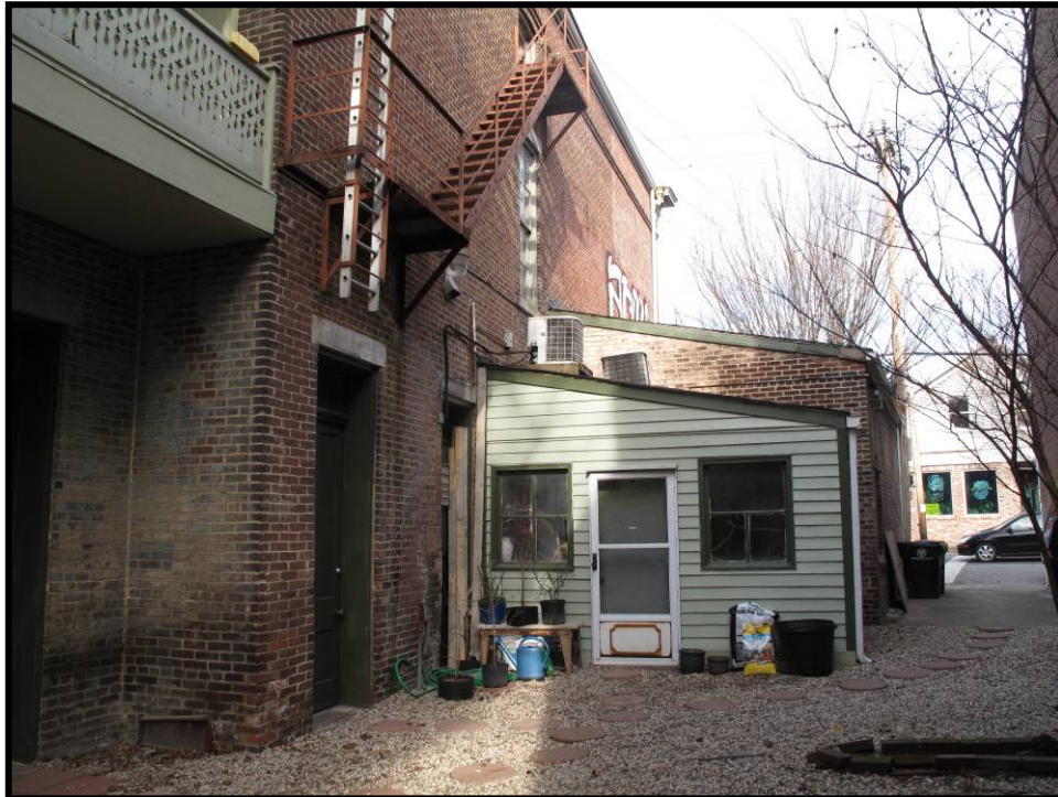
Figure 4. 79 Rear of the Zutt grocery workroom (JFCB-438).
