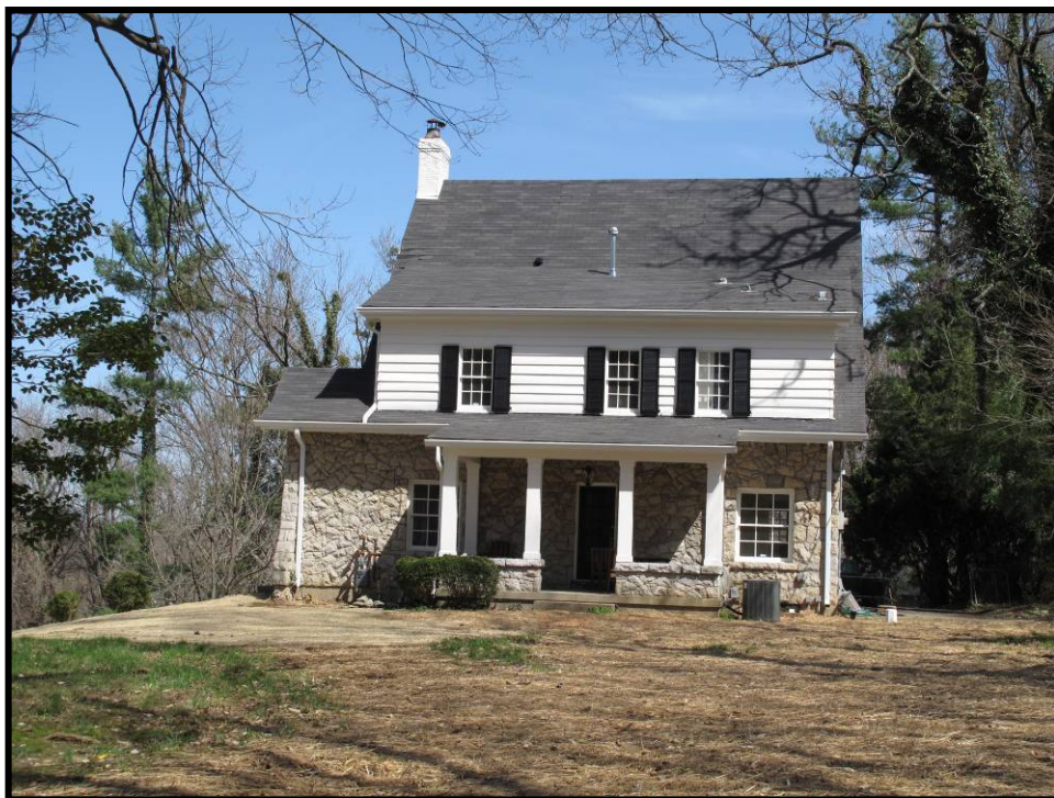
Figure 4. 126 Façade of James T. Taylor House (JF-784).
