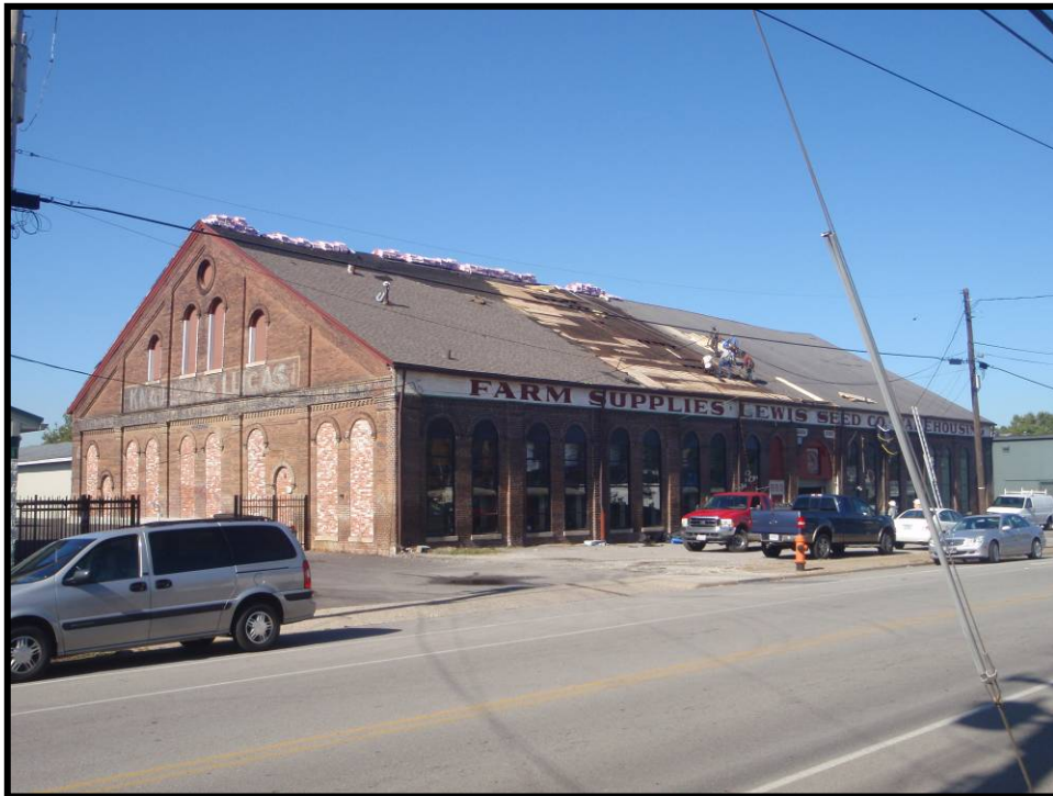
Figure 4. 215 L&N Building, 130 North Spring Street (JFEI-76).
