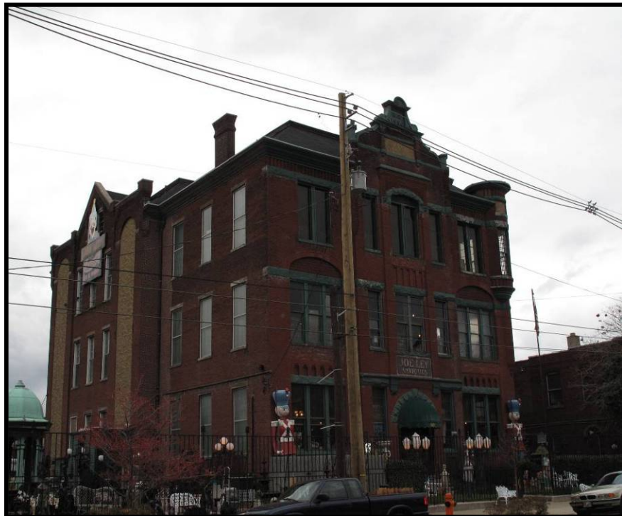
Figure 4. 89 West elevation and façade of Hiram Robert's Normal School (JFCH-19.)
