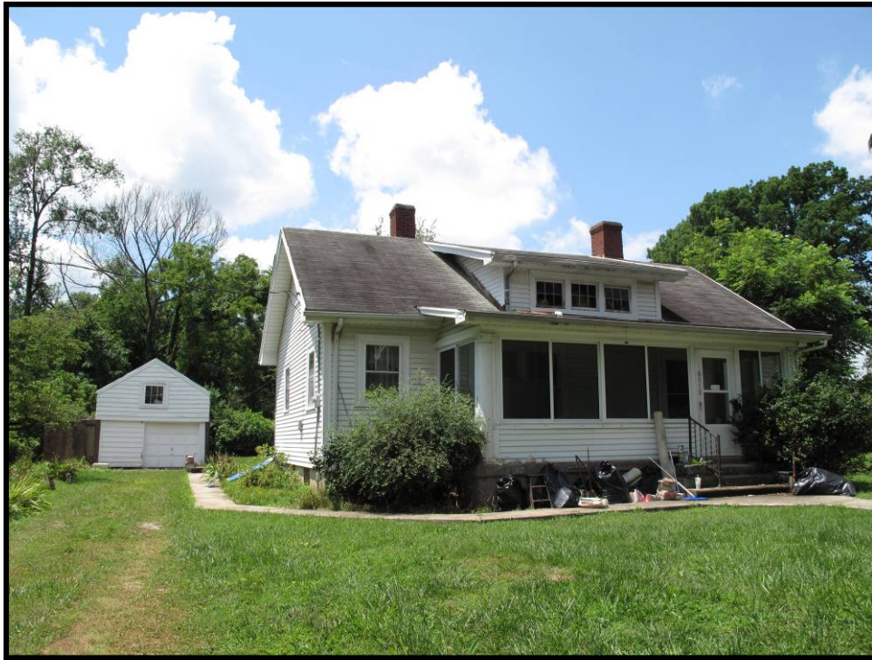
Figure 4. 39 Façade of 6810 Beech Avenue (JF-1865).
