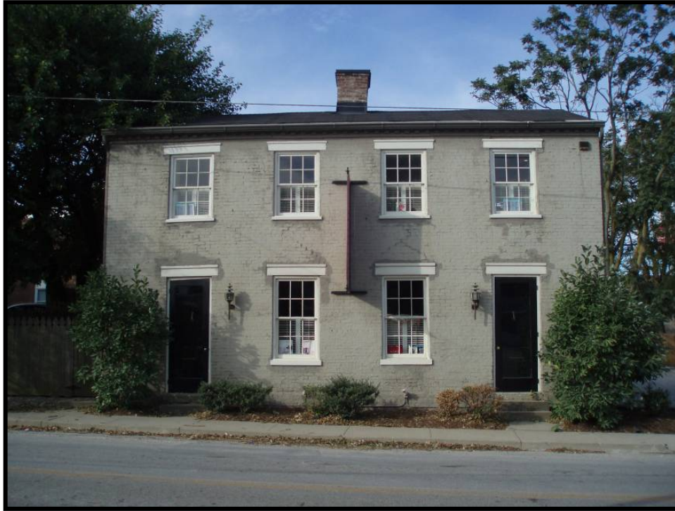
Figure 5. 3 Façade of 1556 Frankfort Avenue (JFCB-395).
