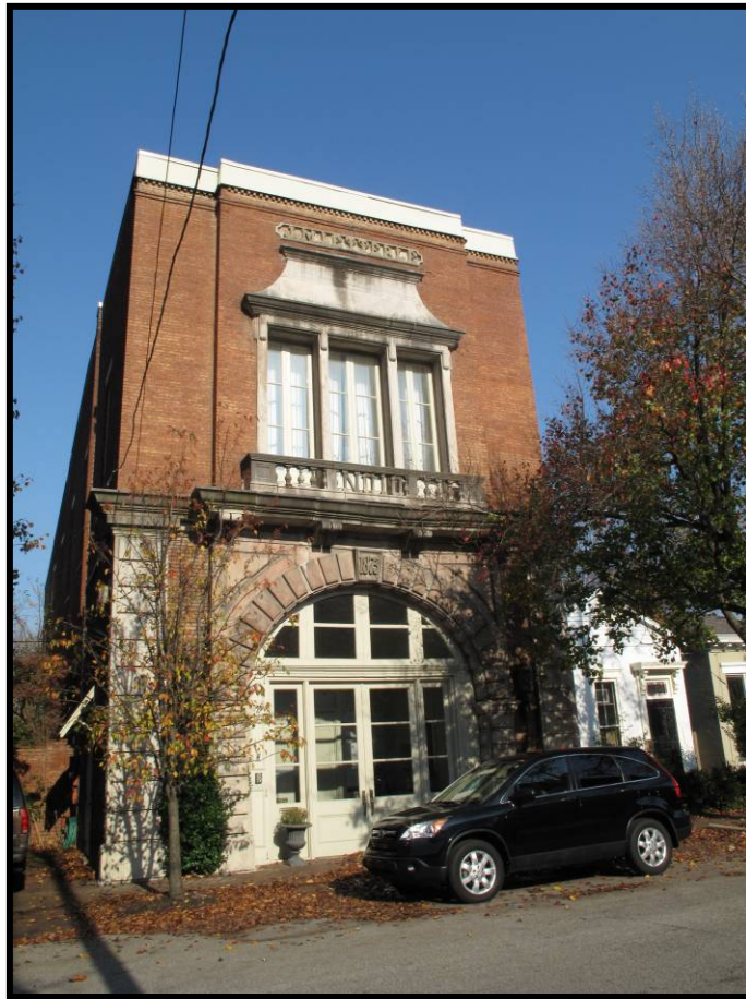
Figure 4. 105 Façade of 1419 East Washington Street (JFCB-336).
