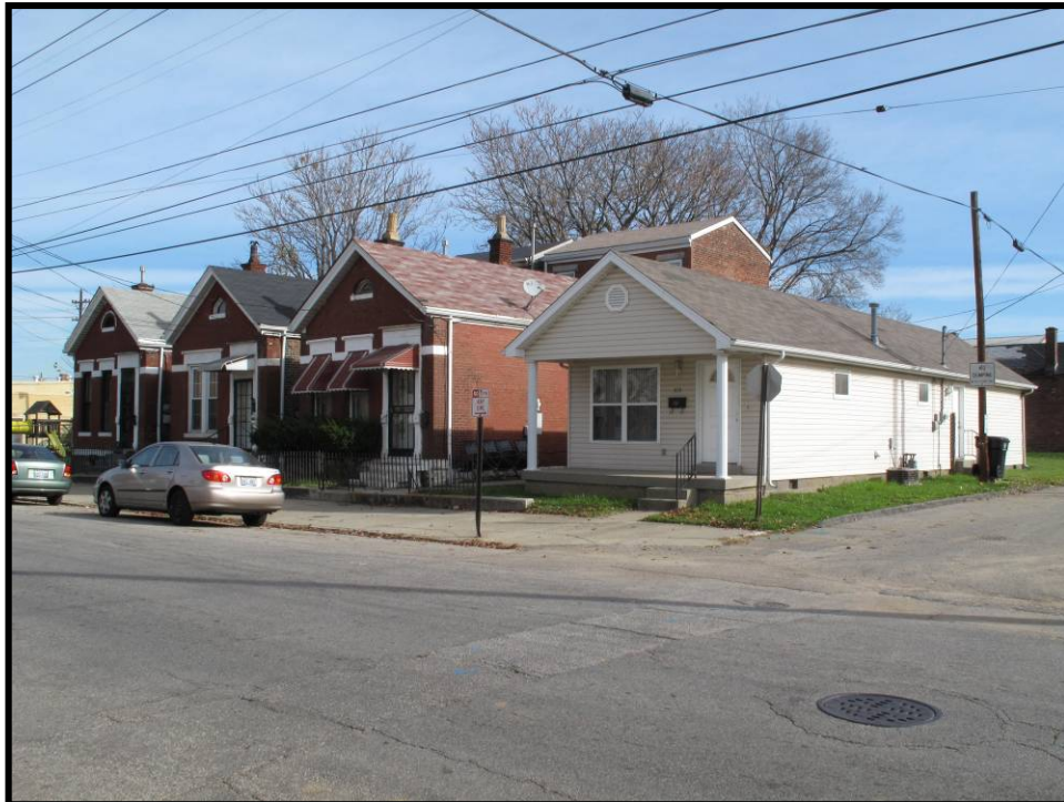
Figure 4. 14 View of shotguns on South Wenzel Street in Phoenix Hill.
