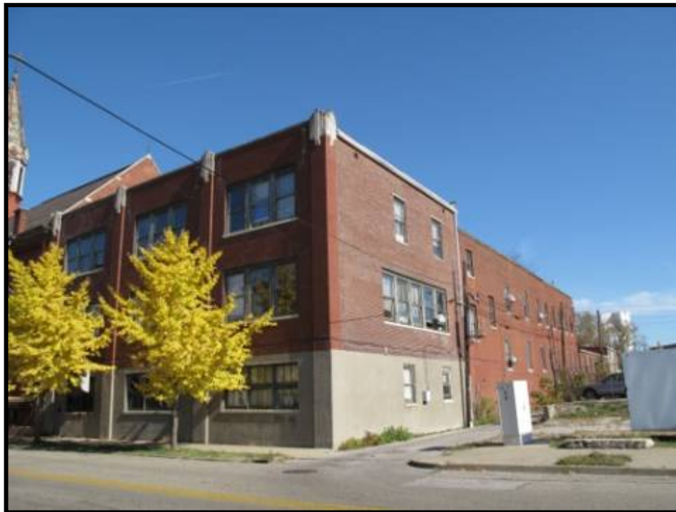
Figure 4. 104 Southwest elevation showing 601 South Shelby at the rear of the Chapel and the 806 E. Chestnut dormitory (later classroom) structures located along Springer Alley.
