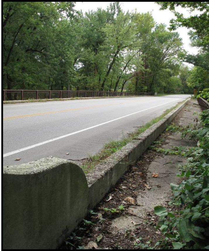
Figure 4. 221 Upper River Road Bridge, looking west down River Road (JF-787).
