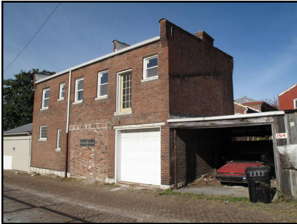
Figure 4. 202 Carriage House at rear of 1312 East Washington, on Bowles Alley.
