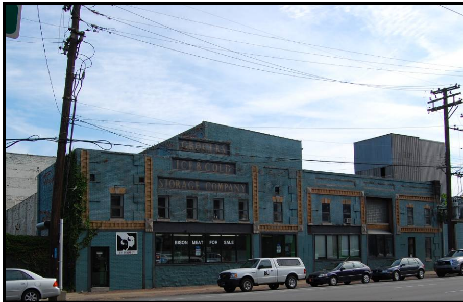
Figure 4. 194 Grocers Ice and Cold Storage, facing northeast (JFCB-634).
