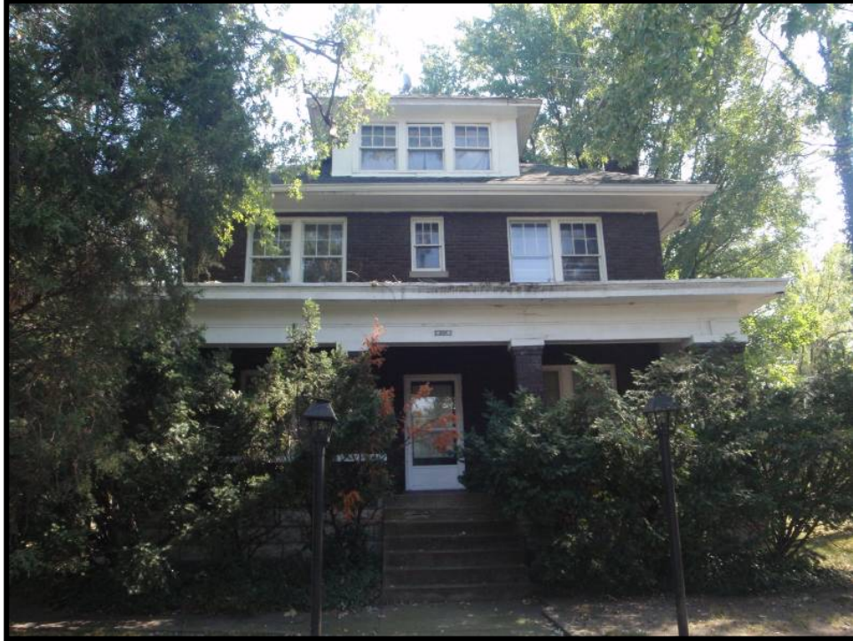
Figure 4. 43 Façade of 1632 Story Avenue (JFCB-446).
