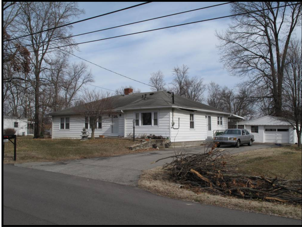
Figure 4. 47 Façade of 6403-6405 Shirley Road (JF-2083).
