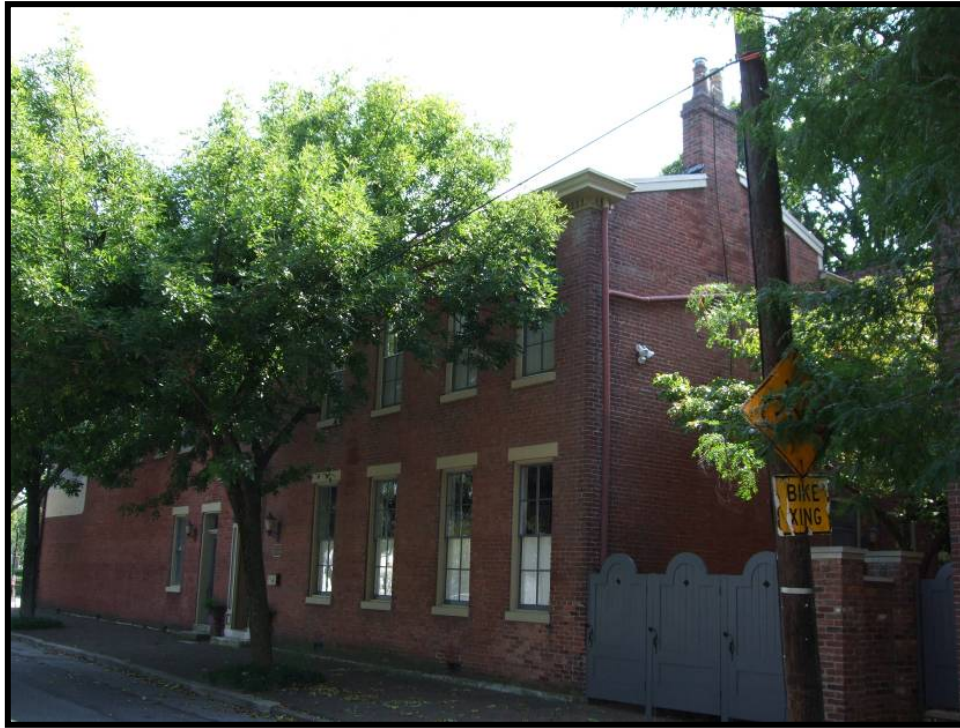
Figure 4. 75 North elevation (Washington Street side) of the Gnau dwelling (JFCB-345).
