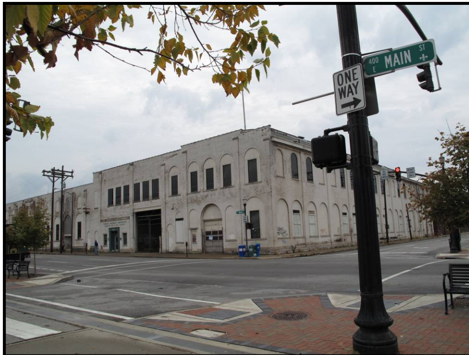
Figure 4. 160 American Machine Company, looking southeast at Main Street and Jackson Street elevations (JFCH-3).
