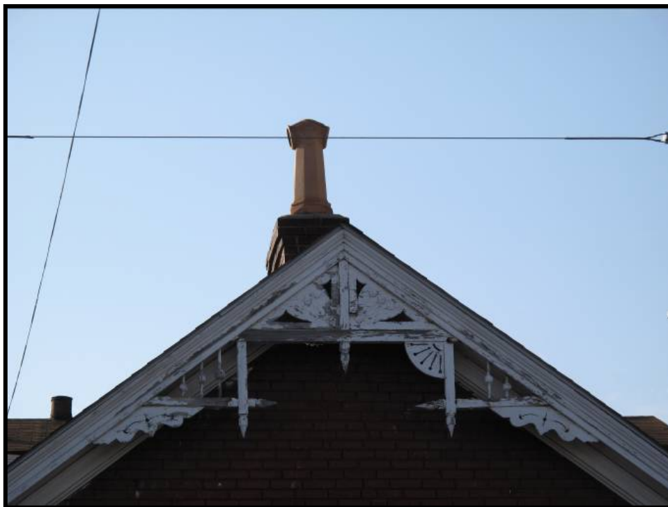
Figure 5. 10 Detail of the bargeboard at 802-804 East Liberty Street (JFCH-195).
