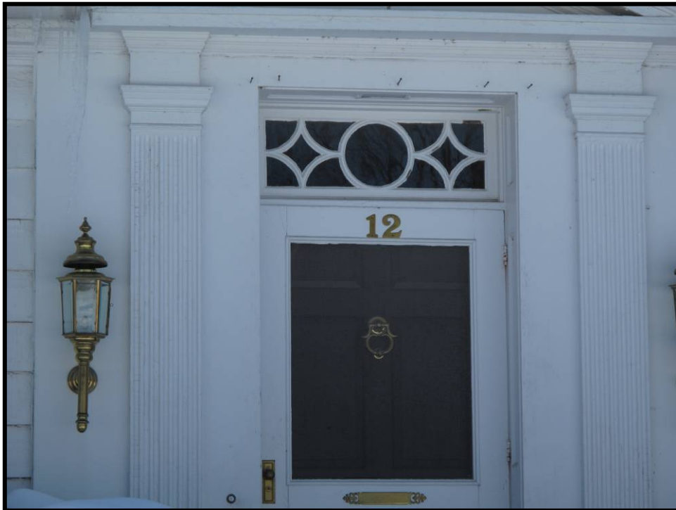
Figure 5. 18 Detail of entryway at 12 River Hill Road (JF-2105).
