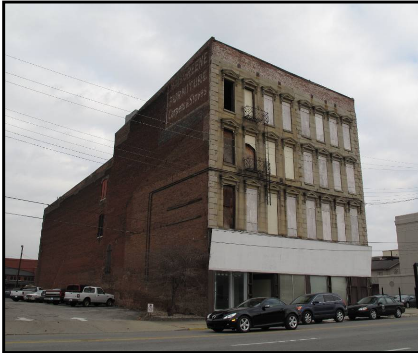
Figure 4. 70 West and south (façade) elevations of 405-415 East Market Street (JFCH-7).
