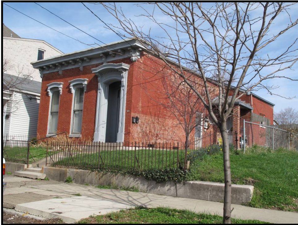
Figure 4. 17 Façade and east elevation of 823 Gray Street (JFCH-383).
