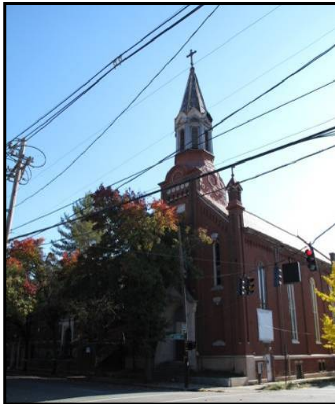
Figure 4. 103 Northwest elevation of Ursuline Convent Chapel (JFCH-352).
