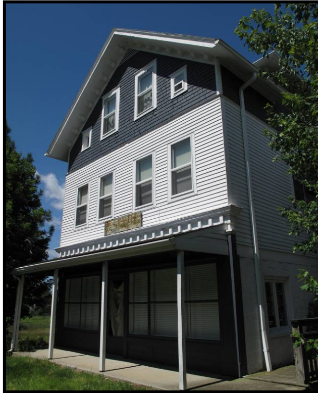
Figure 4. 83 Façade and east elevation of the Prospect Store (JF-444).
