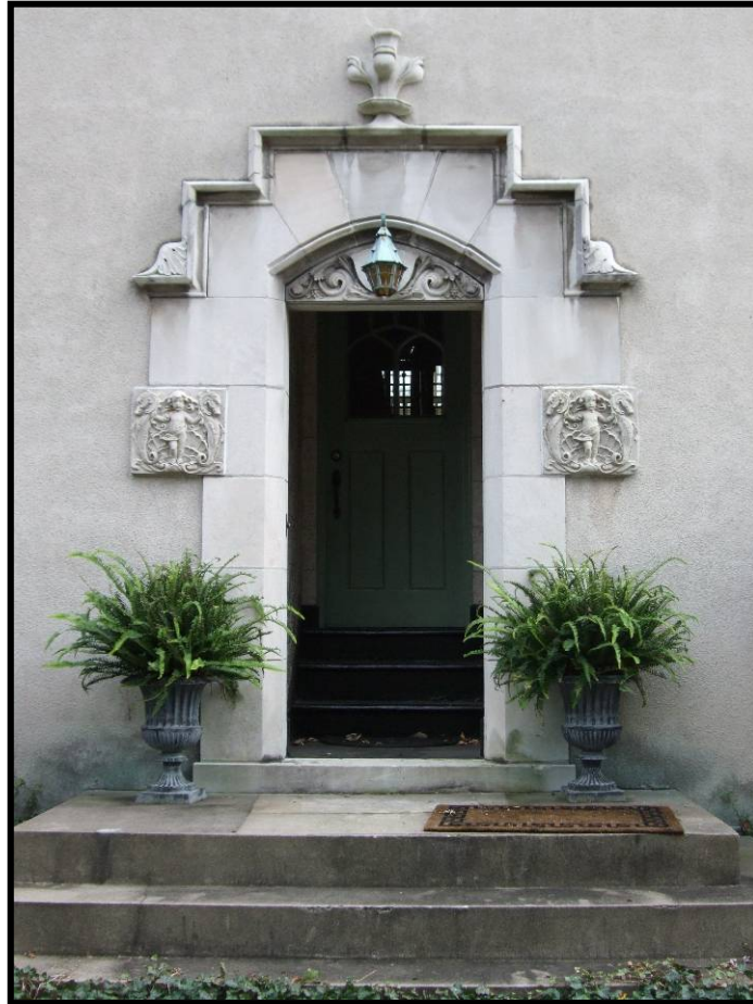
Figure 4. 56 Detail of entryway, 26 River Hill Road (JF-2111).
