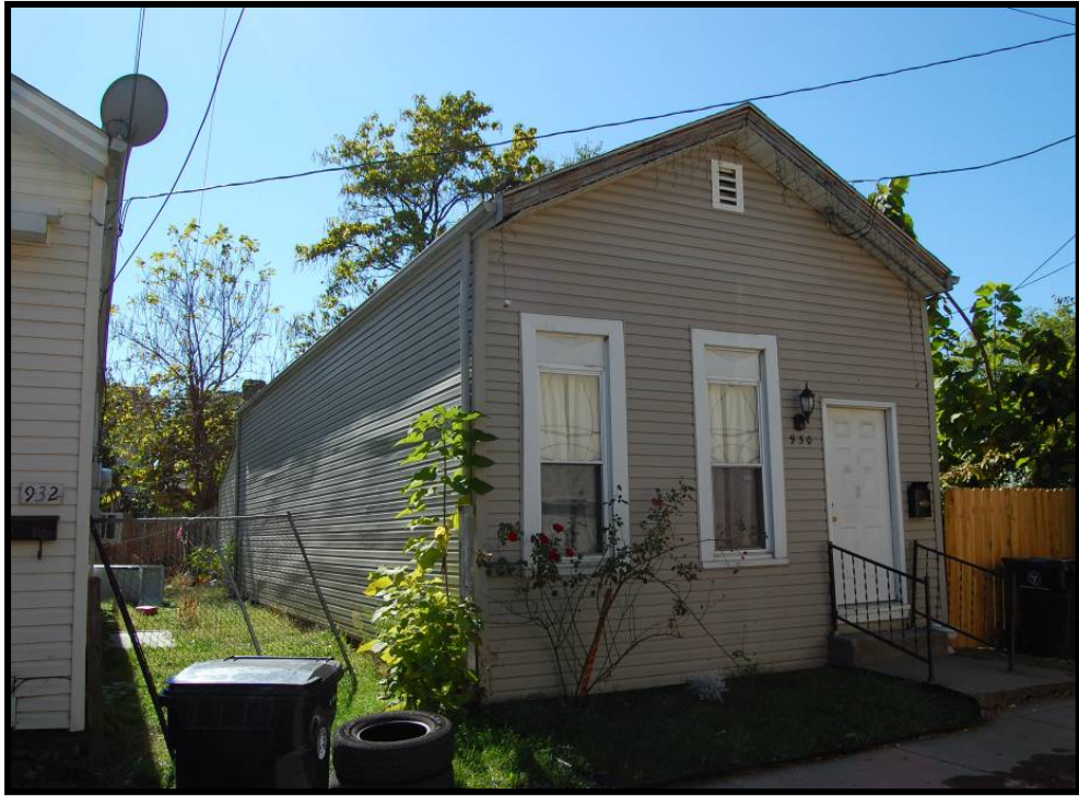
Figure 4. 204 930 Ballard Street (JFCH-1069), between Campbell and Wenzel.
