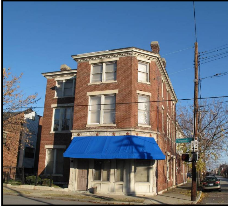
Figure 5. 31 Façade of 845-847 Muhammad Ali Boulevard (JFCH-469).
