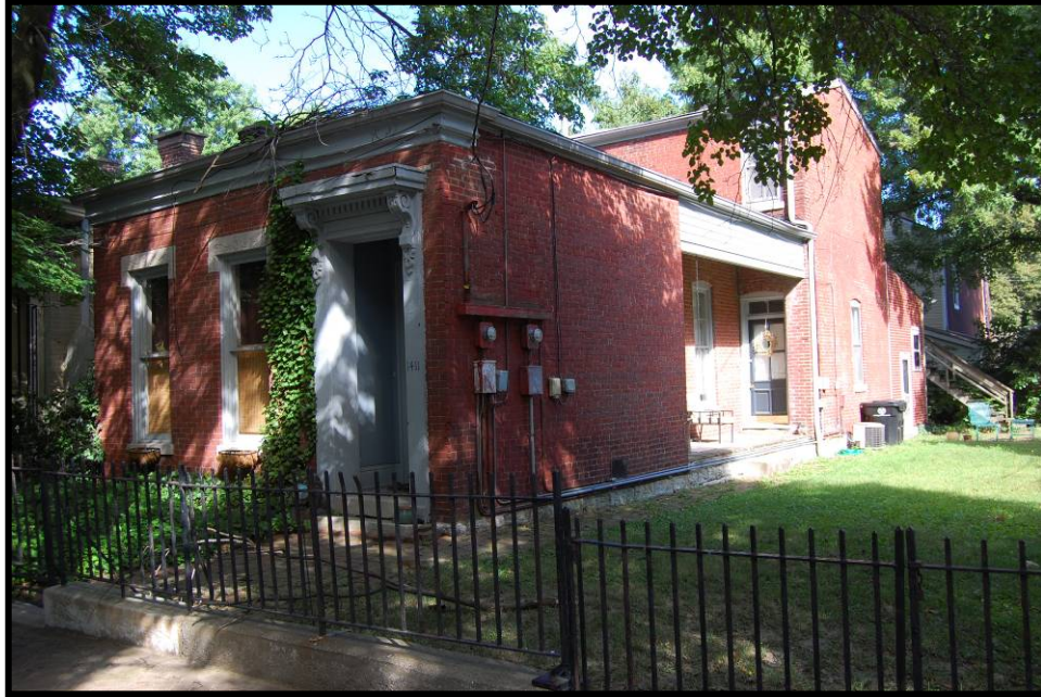
Figure 4. 27 Façade and east elevation (showing recessed side porch) of 1411 East Washington Street (JFCB-334).
