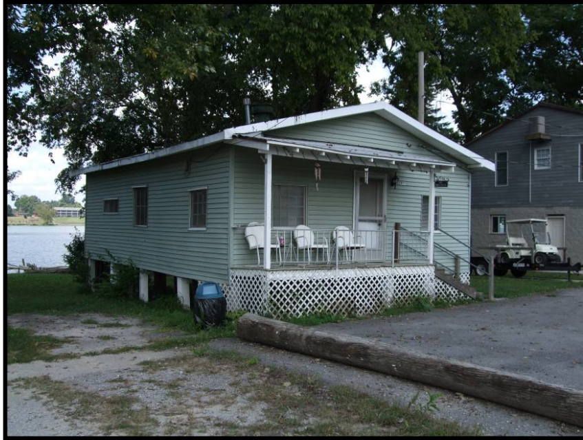
Figure 4. 139 West and south elevations of 2801 Waldoah Beach (JF-1927).
