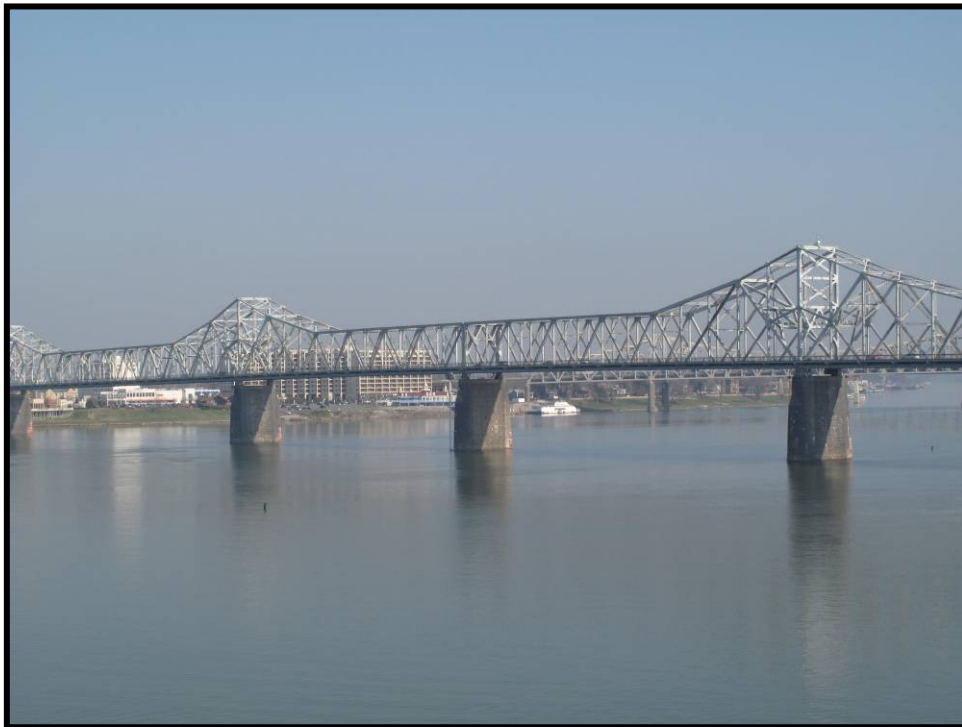
Figure 4. 227 George Rogers Clark Memorial Bridge, looking northeast (JFCB-217).
