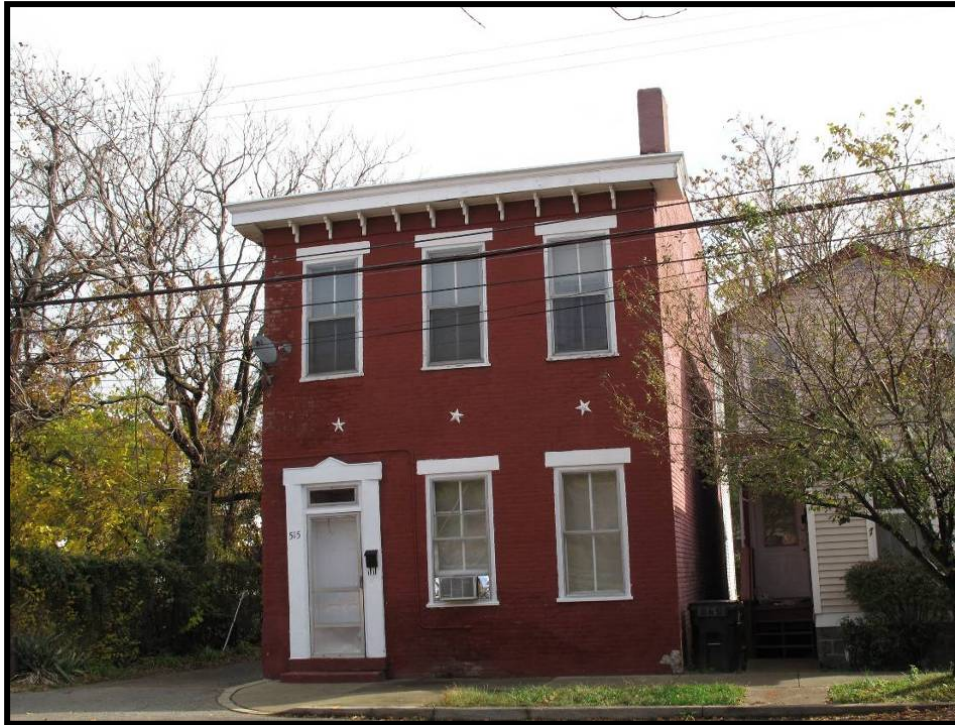
Figure 4. 11 Façade of 515 Campbell Street (JFCH-913).
