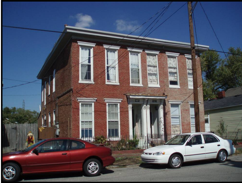
Figure 4. 36 West elevation and façade of 1025-1027 East Washington Street (JFCB-208 and 209).
