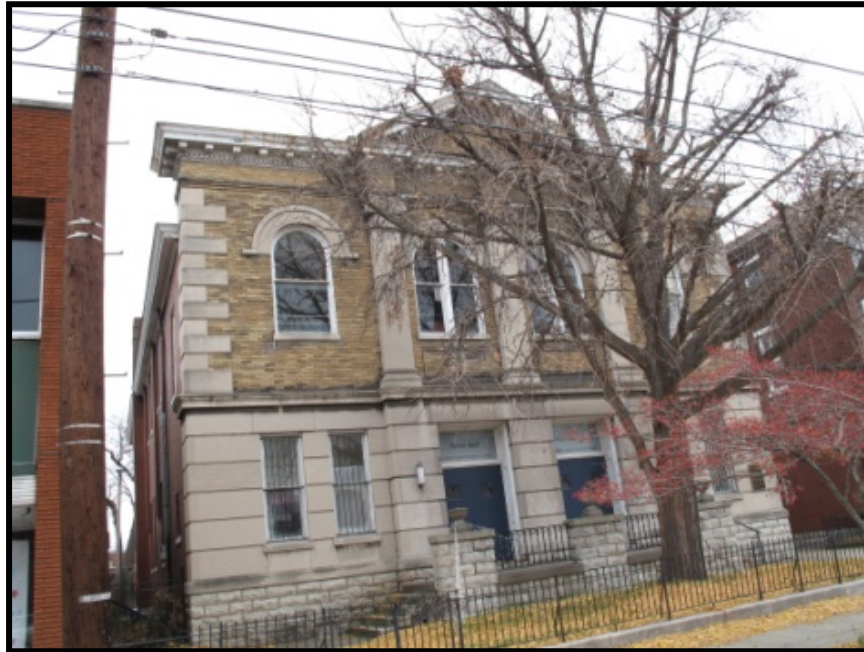
Figure 4. 114 Southwest elevation of St. John's Parish Hall and Renaissance Theater (JFCH-21).
