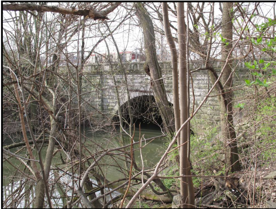
Figure 4. 223 Frankfort Avenue Bridge over Beargrass Creek (JFCB-718).
