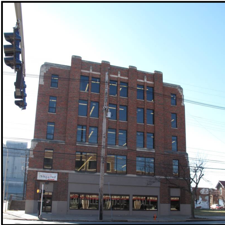
Figure 5. 34 Façade of 834 East Broadway (JFCH-1315).
