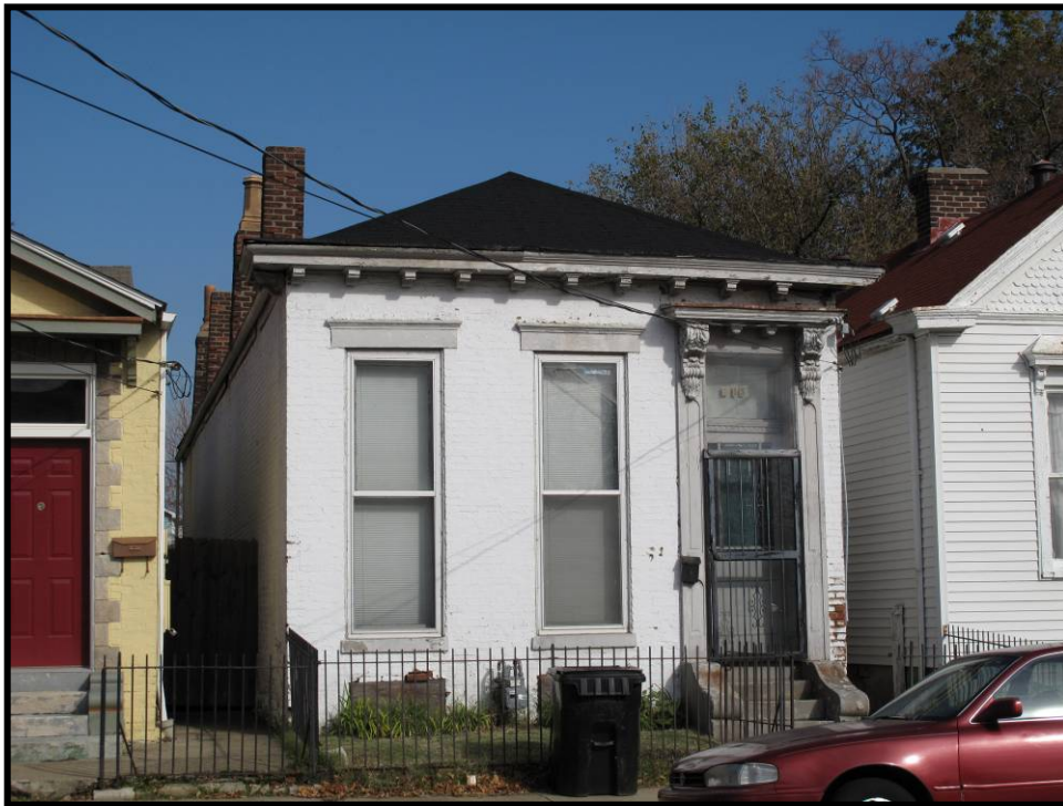
Figure 4. 16 Façade of 915 East Madison Street (JFCH-288).
