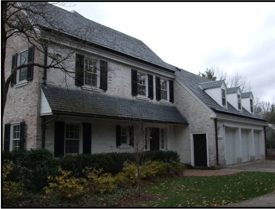
Figure 4. 54 Attached three-car garage and service wing, 6 River Hill Road (JF-2049).
