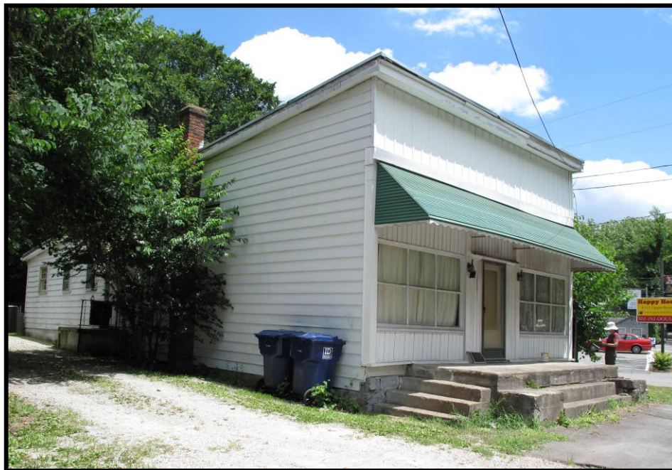
Figure 4. 85 West elevation and façade of Walter Bader’s Grocery Store (JF-937).
