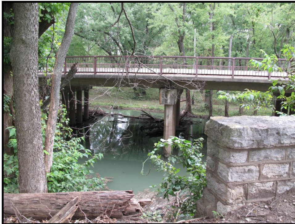
Figure 4. 222 Upper River Road Bridge (JF-787) as seen from old bridge (JF-786).
