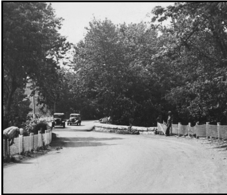
Figure 4. 219 Goose Creek Bridge on River Road, circa 1935. 215
