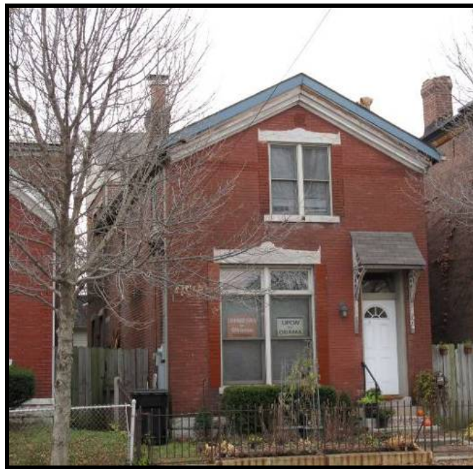
Figure 4. 22 Façade of 902 Liberty Street (JFCH-1016).
