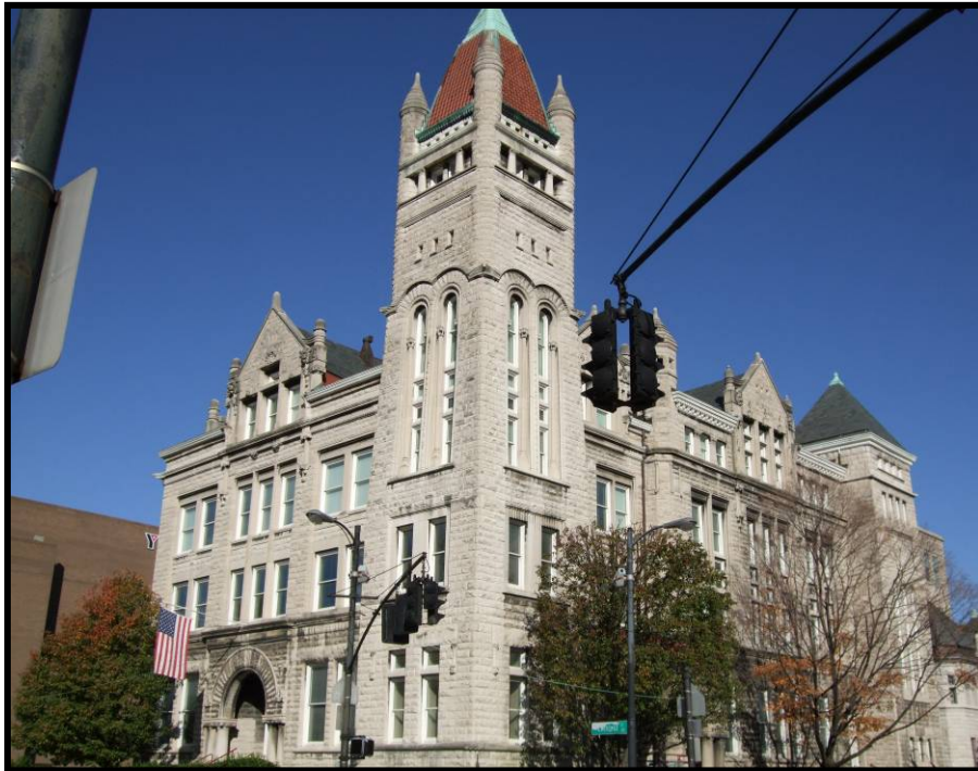
Figure 4. 155 South and east elevations of Louisville Medical College Building (JFCD-159).
