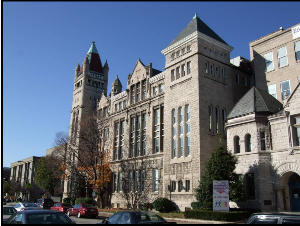
Figure 5. 33 Louisville Medical College, facing southwest (JFCD-159).
