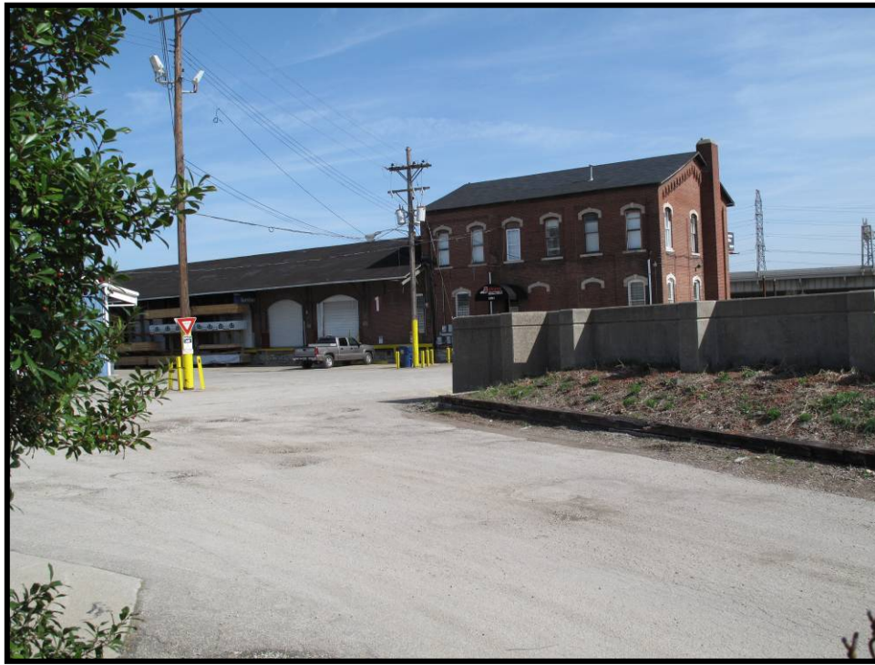
Figure 4. 210 Pennsylvania Lines Freight Depot, 1301 Portland Avenue (JFWP-164).
