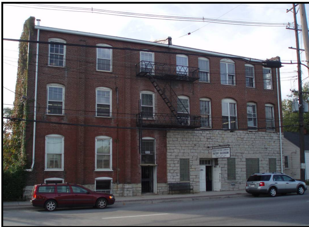
Figure 4. 179 Façade of Hadley Pottery Building, facing southwest (JFCB-401).
