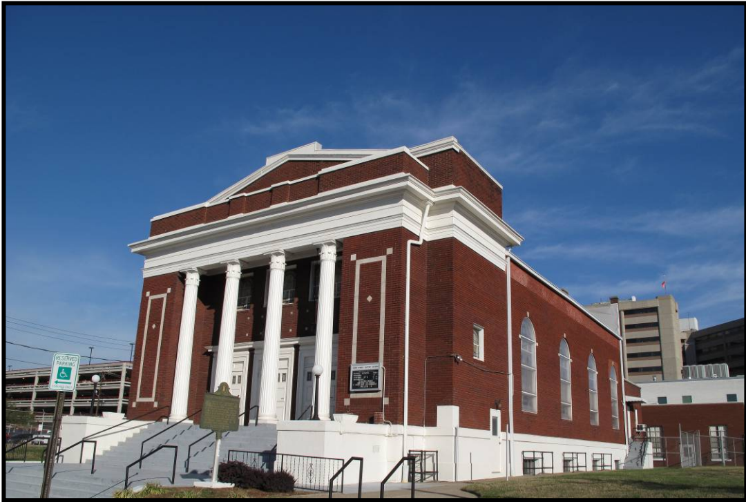
Figure 4. 124 Green Street Baptist Church, facing northwest (JFCH-421).
