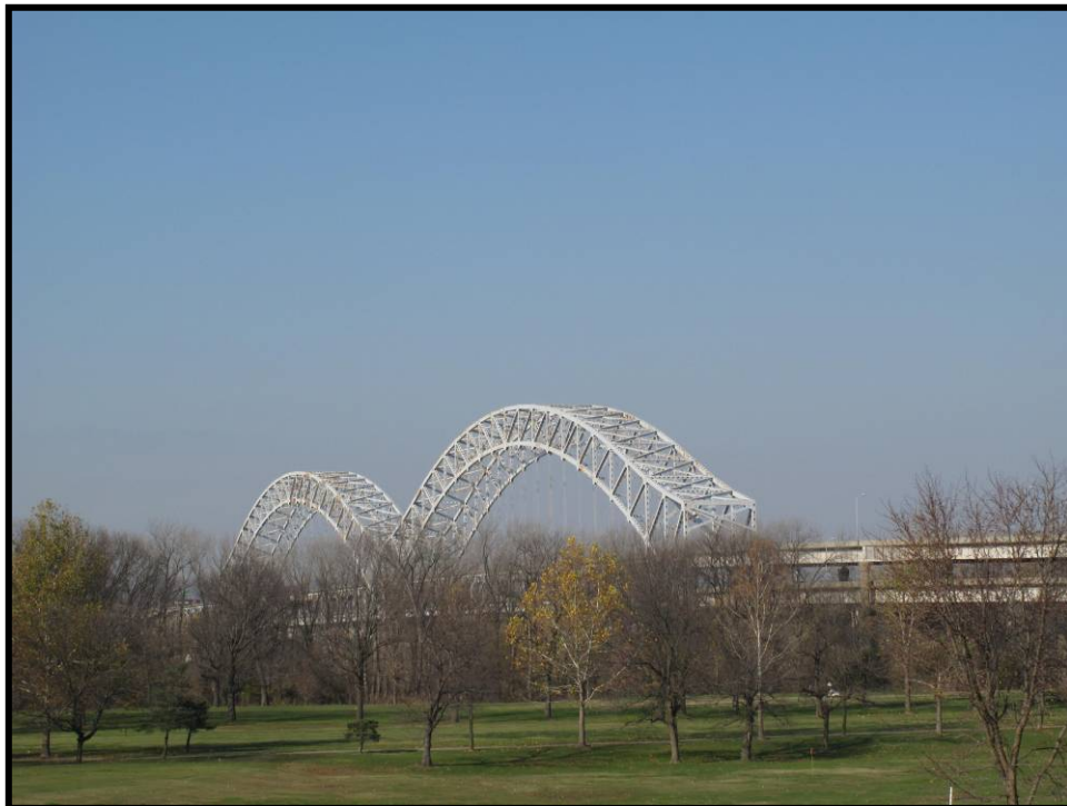
Figure 4. 228 Sherman Minton Bridge, looking northeast (JFWP-589).
