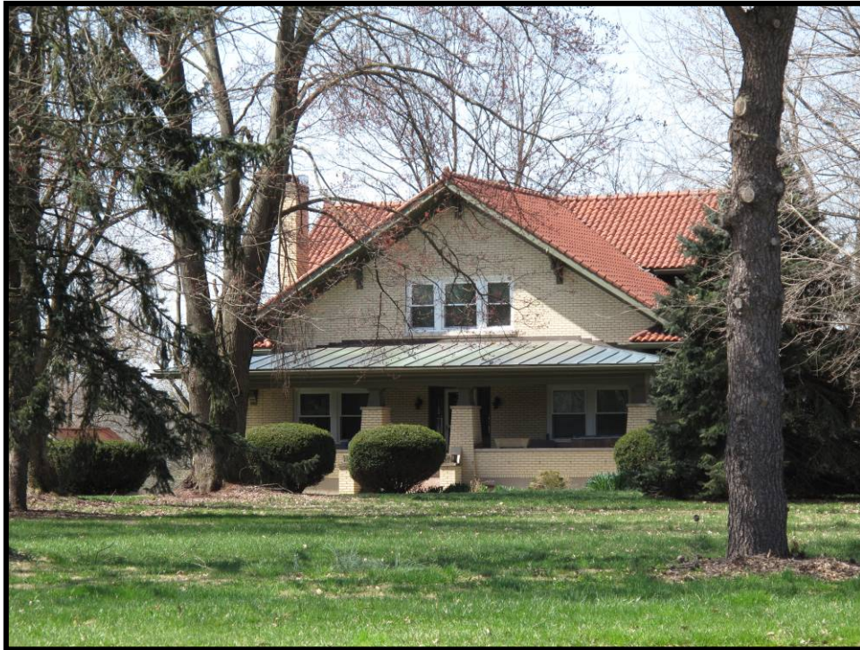
Figure 5. 15 Façade of the William C. Baass House (JF-839).
