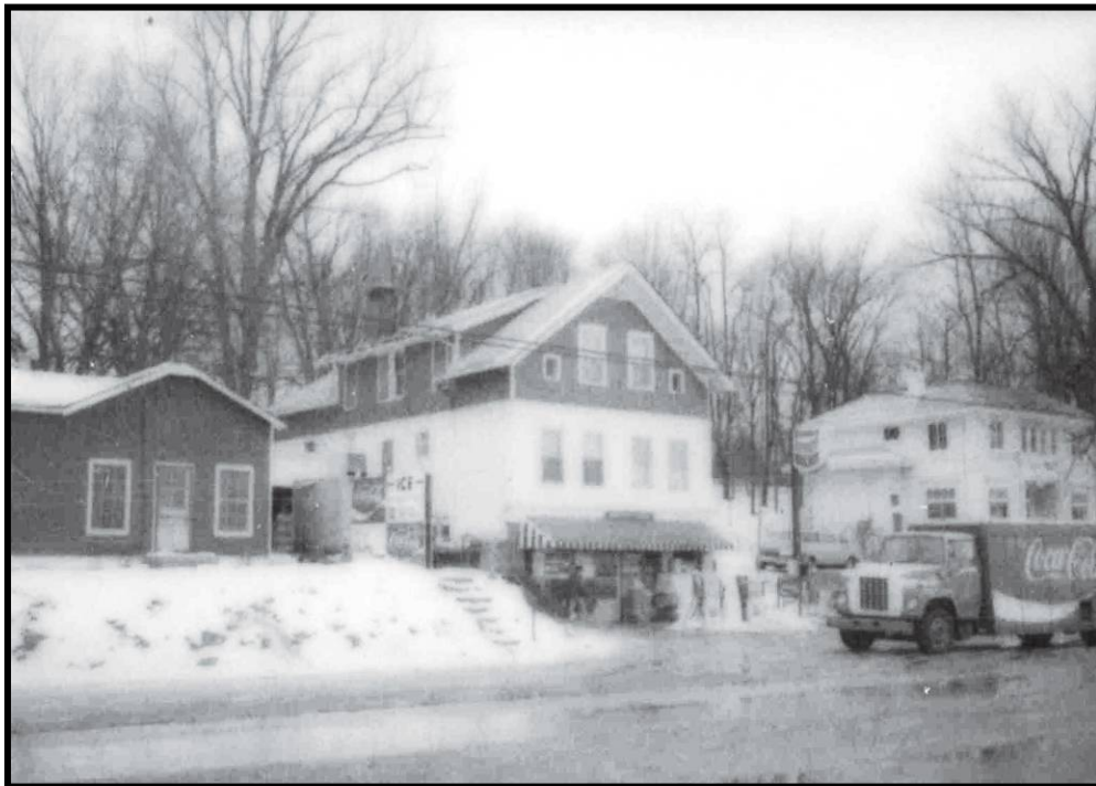
Figure 4. 84 Prospect Store before it was moved across US 42. Photo courtesy Kentucky Heritage Council.
