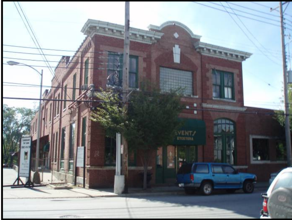
Figure 4. 181 Façade of 1332 Story Avenue, Oertel's Bottling Plant (JFCB-310).
