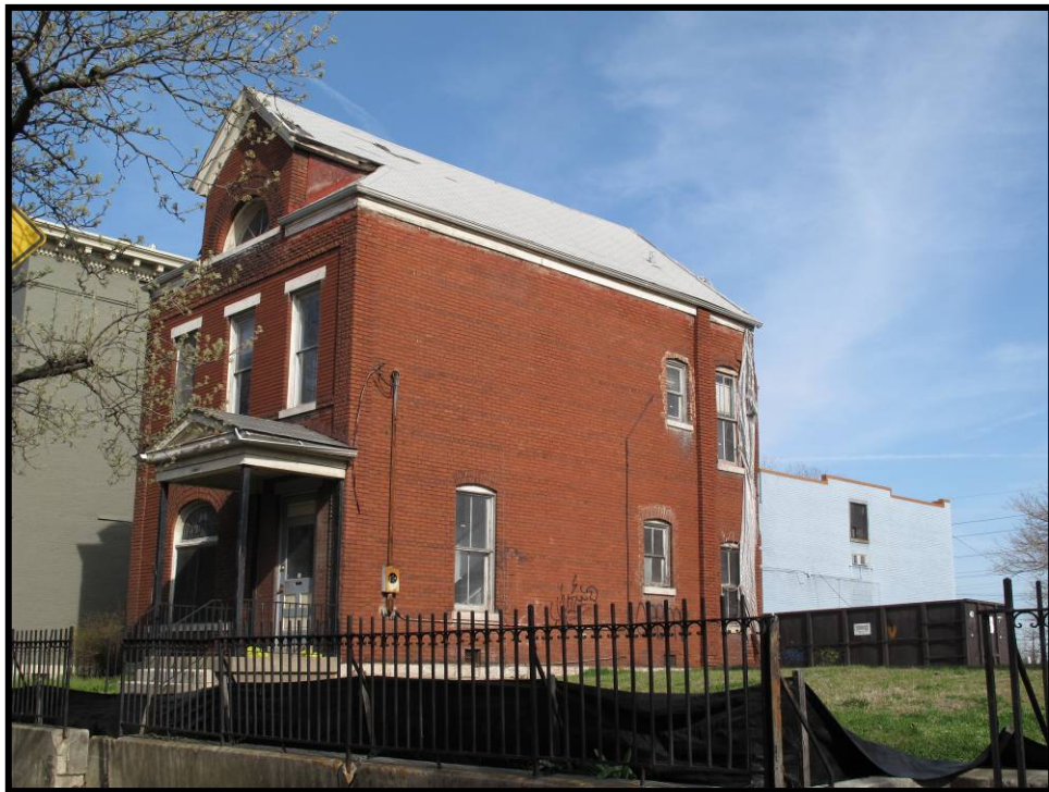
Figure 4. 132 809 East Washington Street, looking northwest (JFCB-72). The rear of the Wesley House gymnasium is visible to the right of 809 East Washington Street.
