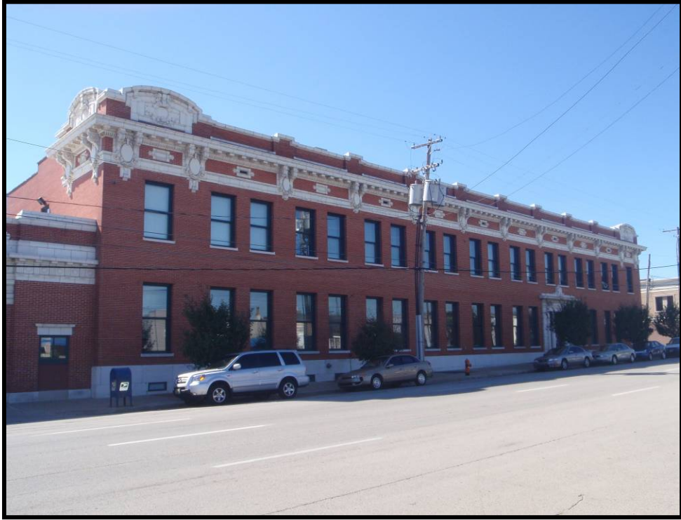
Figure 4. 172 Main Street elevation of the Bourbon Stockyards Exchange Building (JFCB-621).
