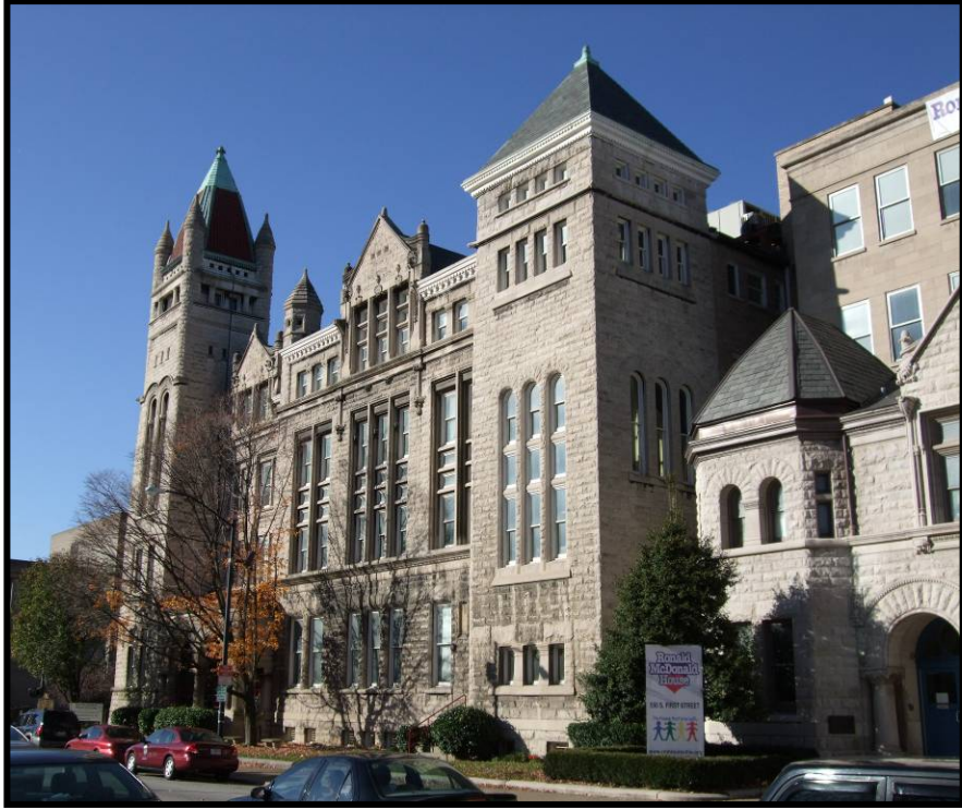
Figure 4. 156 Louisville Medical College, façade, looking southwest (JFCD-159).
