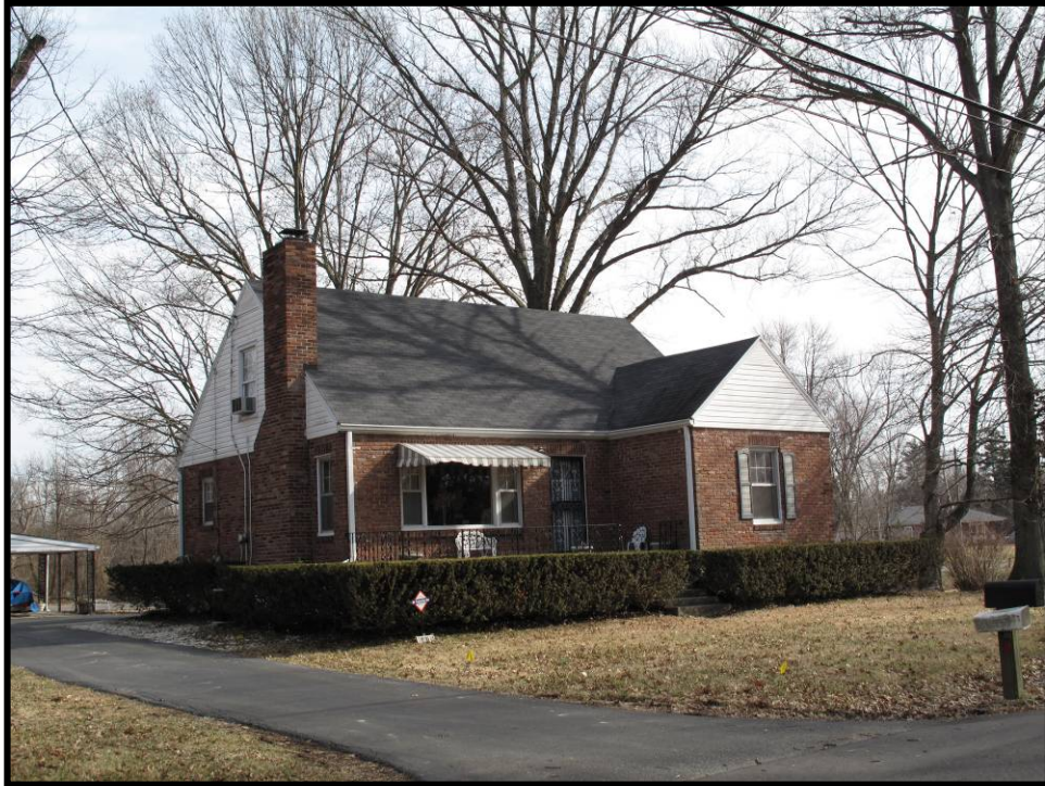
Figure 5. 24 Façade of 6415 Shirley Avenue (JF-1884).
