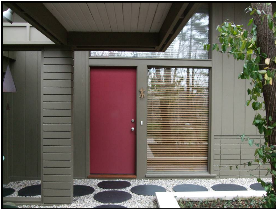
Figure 5. 26 Central entry of 7425 Woodhill Valley Road (JF-1004).
