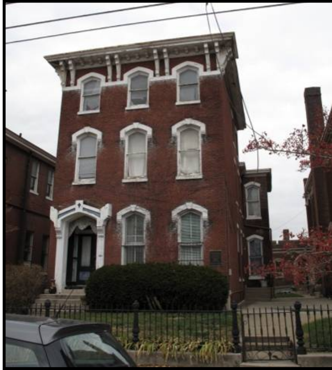
Figure 4. 113 Southeast elevation of St. John's Parish House (JFCH-22).
