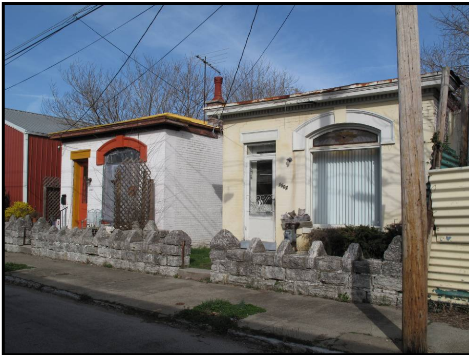
Figure 4. 18 Façades of 1505 and 1507 Quincy Street (JFCB-678 and 679).
