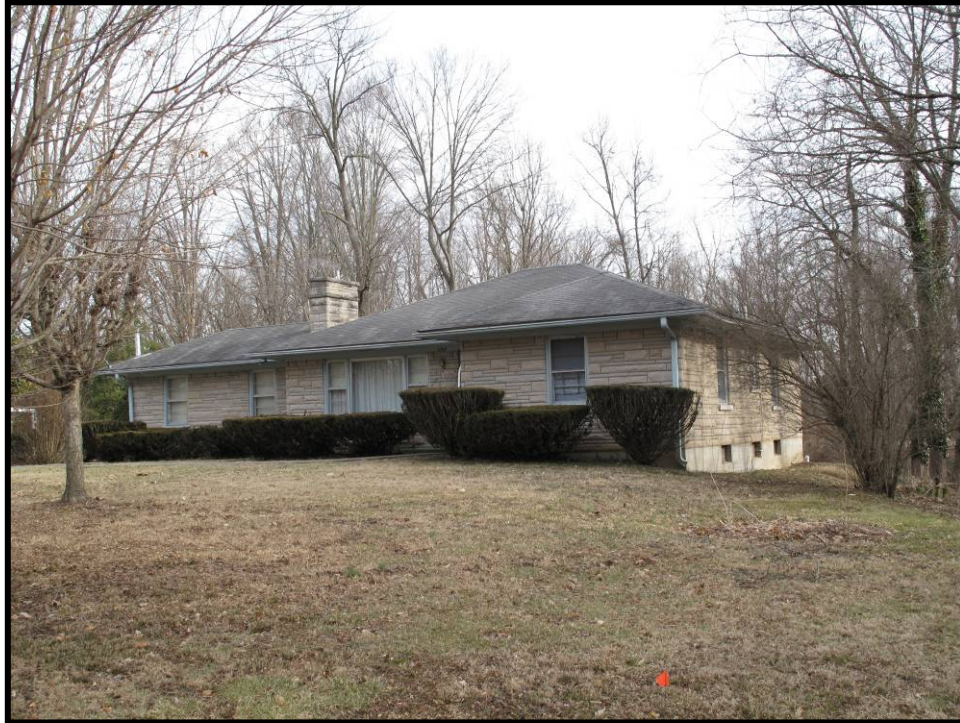
Figure 4. 46 Façade of 6707 Shirley Avenue (JF-1893).
