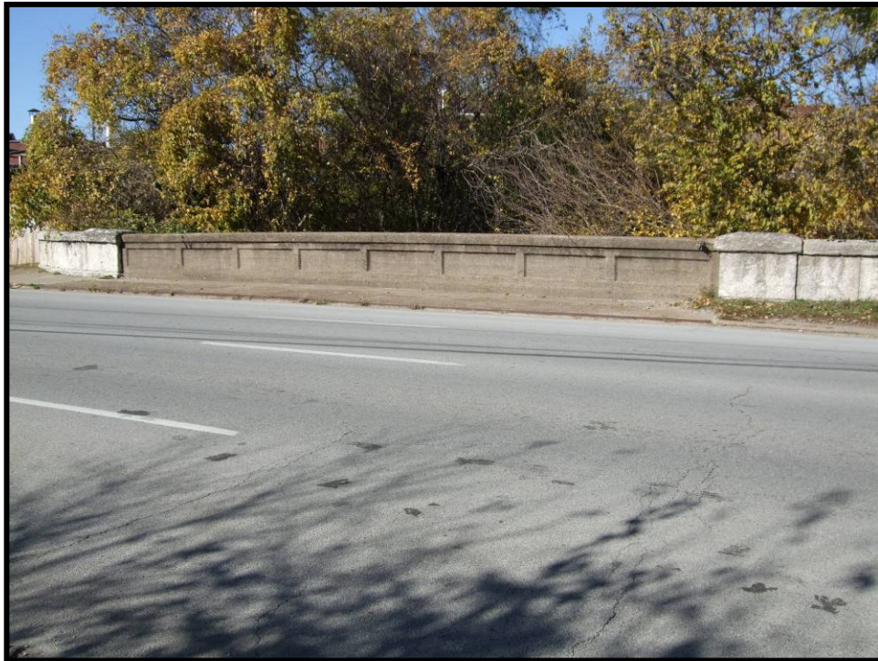
Figure 4.224 Main/Mellwood Bridge over Beargrass Creek (JFCB-719).
