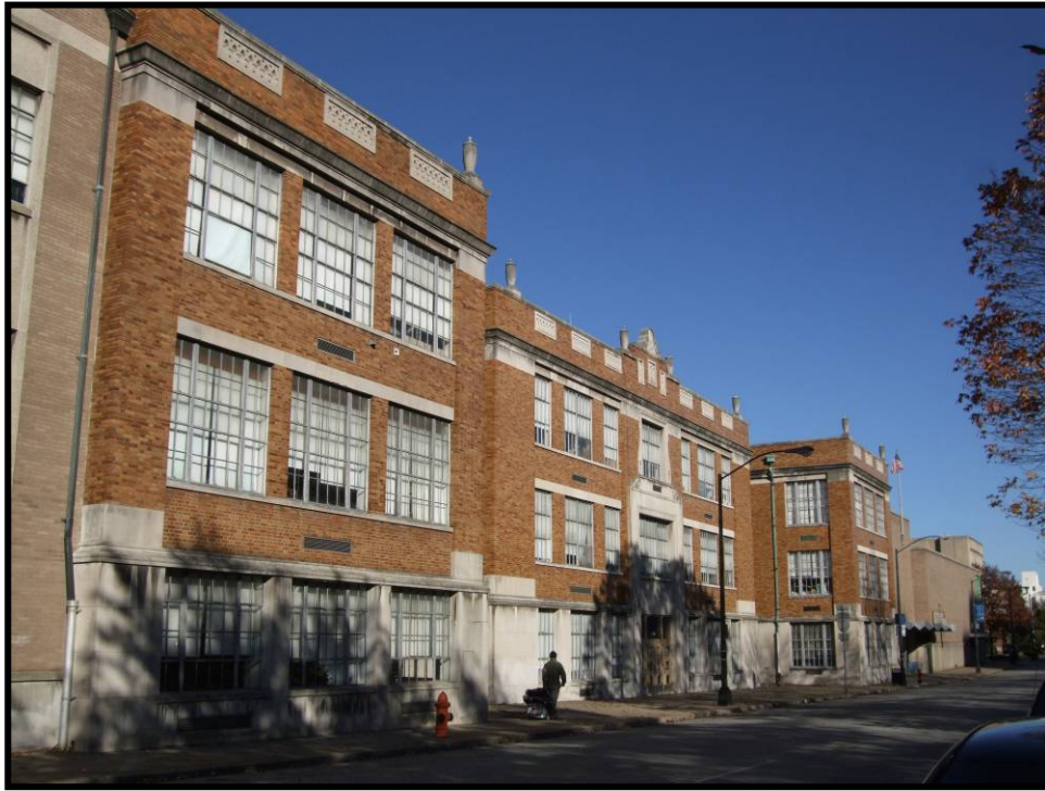
Figure 4. 94 Ahrens Trade School, looking northwest (JFCD-314).
