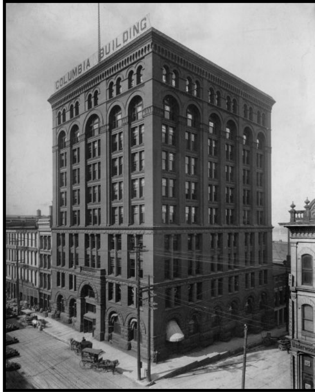
Figure 3. 17 Columbia Building at Fourth and Main Streets (no longer extant), circa 1920. 346
