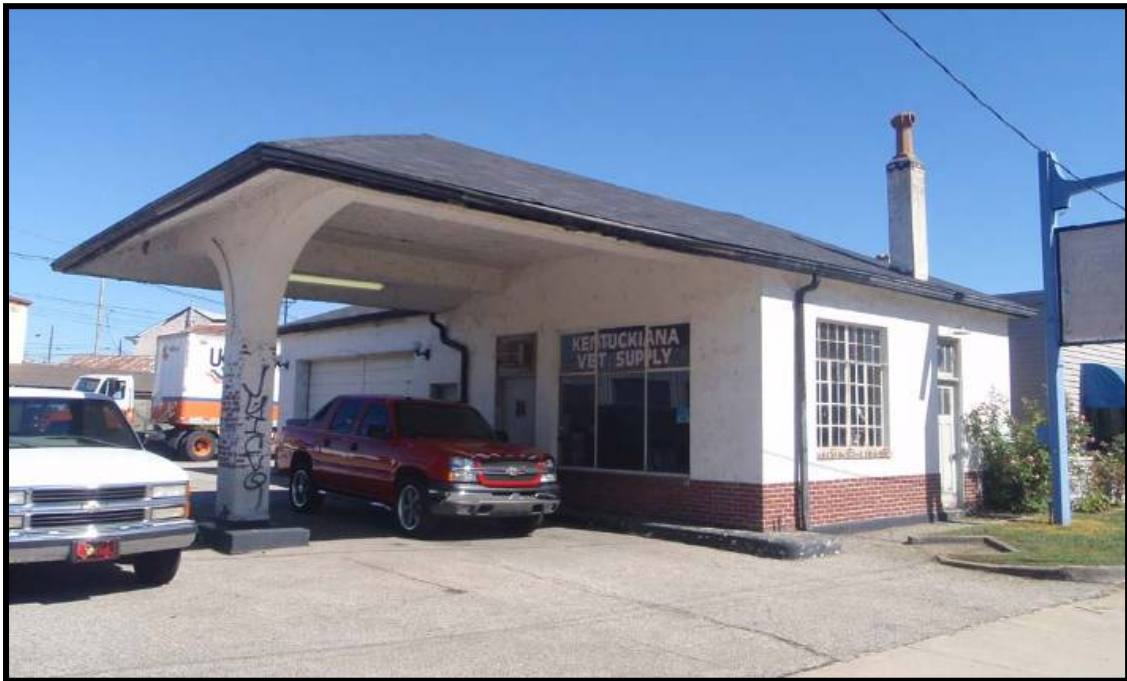
Figure 4. 234 Southwest elevation of 101 North Johnson Street (JFCB-618).
