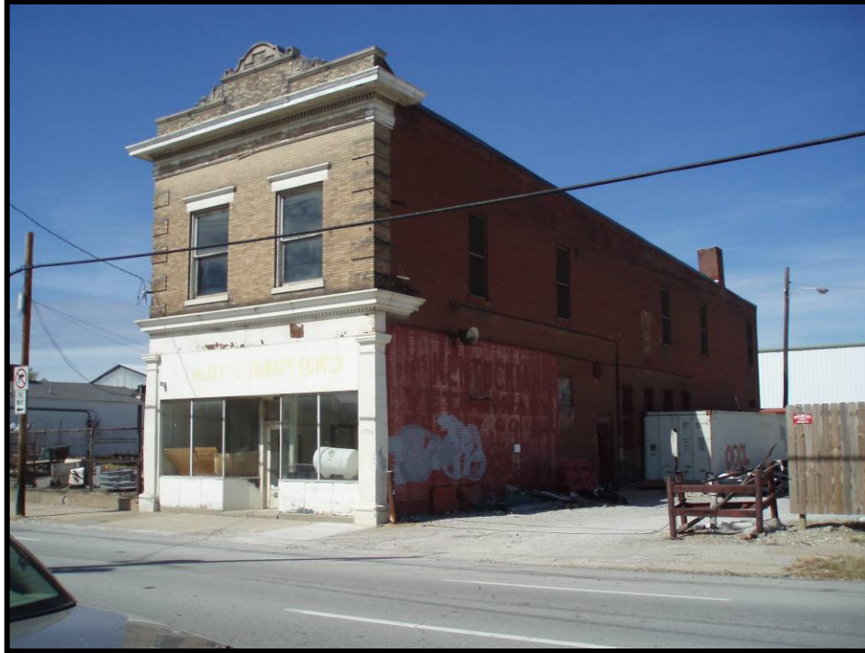
Figure 4. 67 1033 Story Avenue (JFCB-244).
