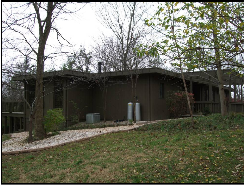
Figure 4. 62 Circa 1959 Norman Sweet-designed house at 7425 Woodhill Valley Road (JF-1004).
