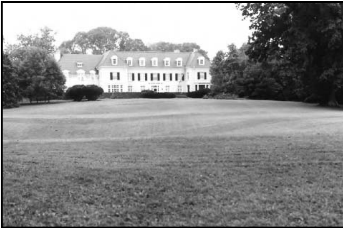
Figure 4. 50 Façade and front lawn of Lincliff (JF-531). 37
