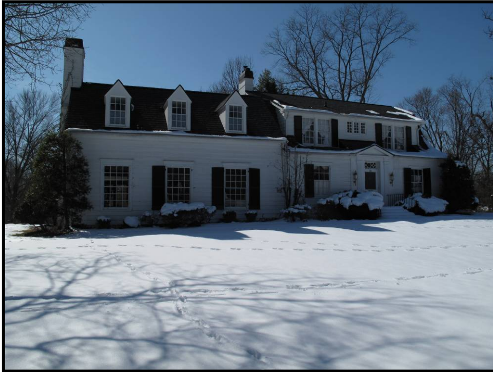
Figure 5. 17 Façade of 12 River Hill Road (JF-2105).
