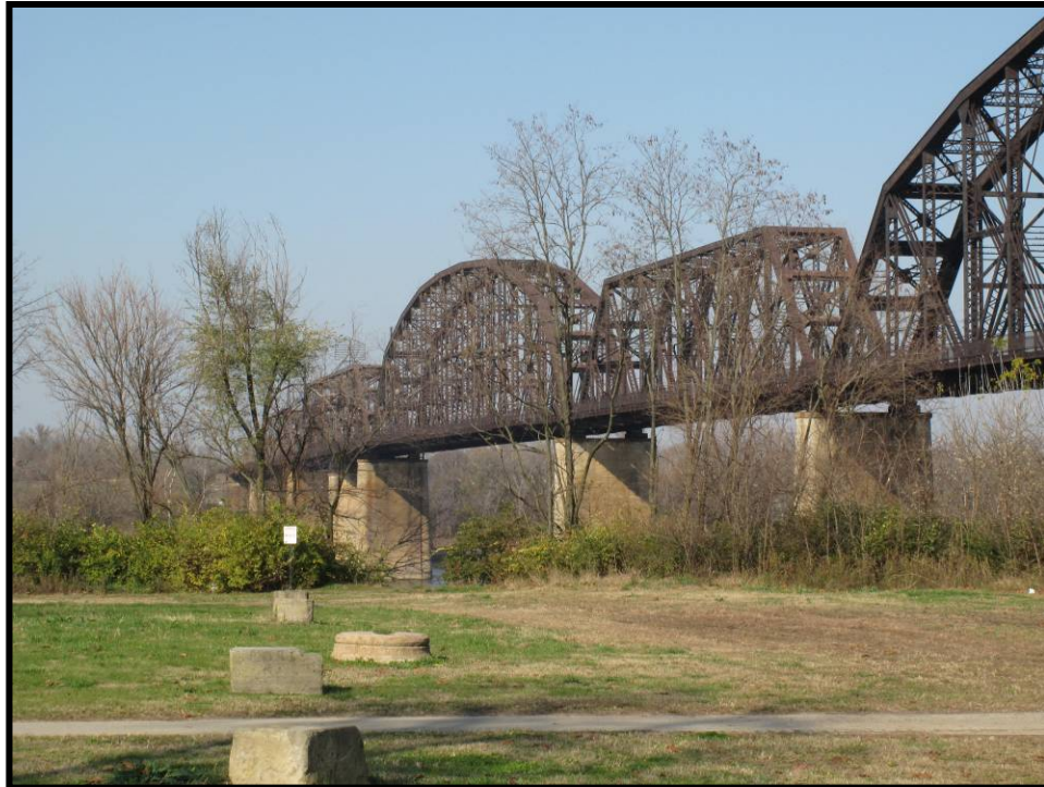
Figure 4. 208 K&I Bridge (JFWP-332).
