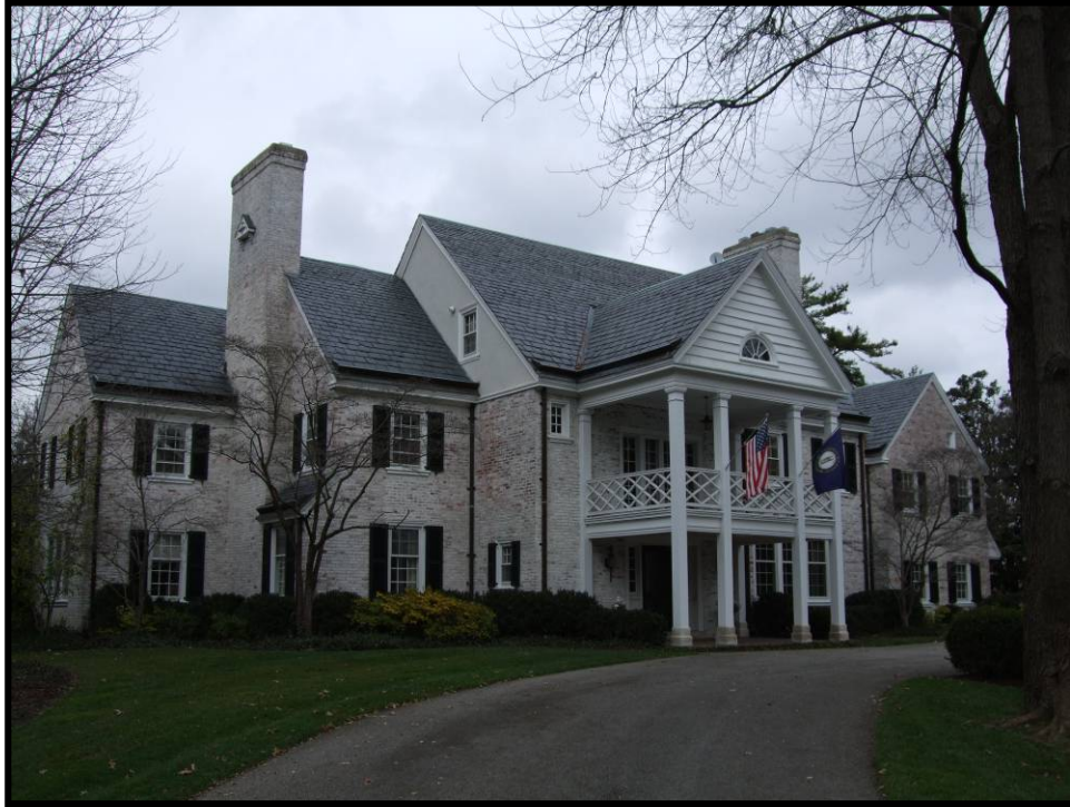
Figure 4. 53 Façade of 6 River Hill Road (JF-2049).
