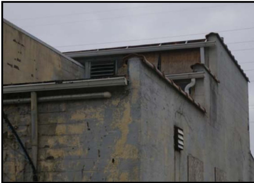
Figure 4. 170 This two-story section of the structure (note terra cotta coping) appears to be an older portion of the complex.
