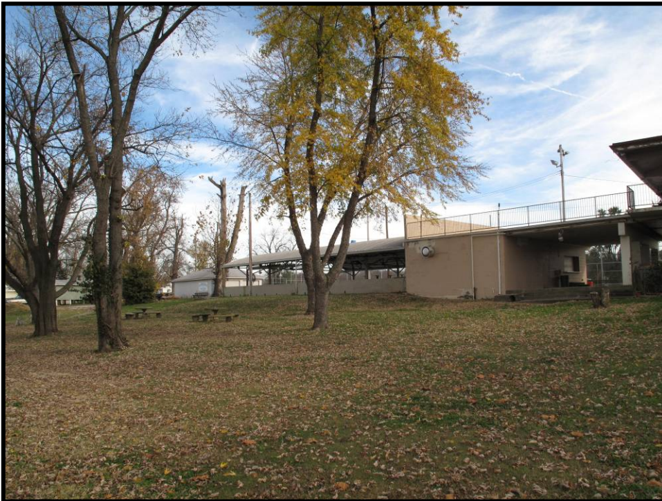
Figure 4. 152 Looking southeast from the river toward the concession stand and public areas of American Turners.
