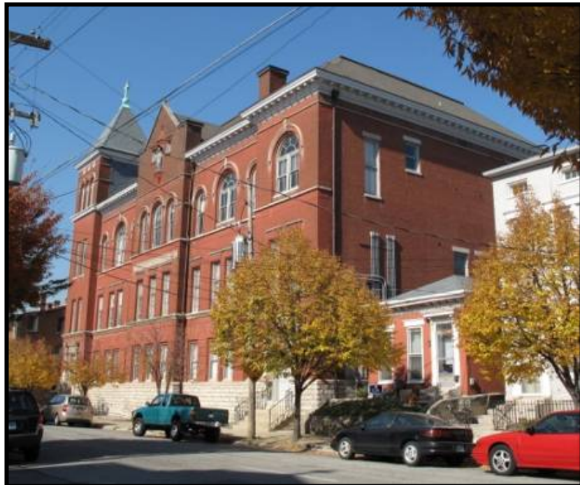
Figure 4. 99 Southeast elevation of St. Martin's Girl's School (Pfarrschule, JFCH-388).
