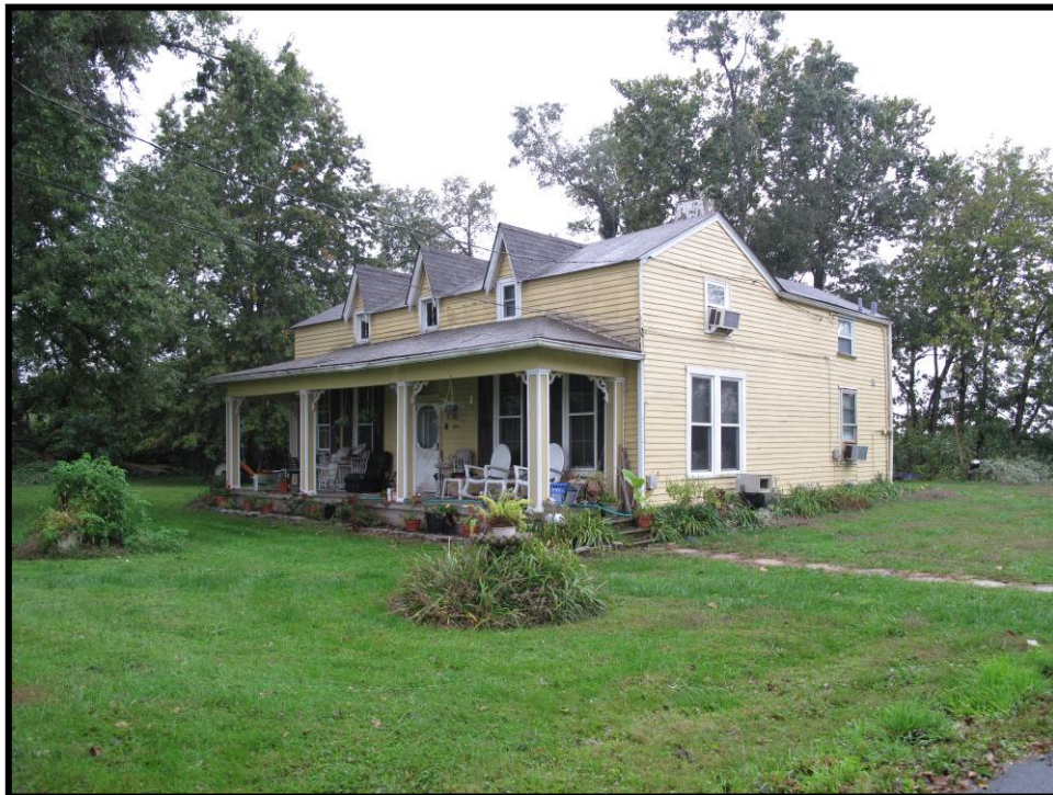
Figure 5. 4 Façade and east elevation of the Dr. J.C. Metcalfe House (JF-455).
