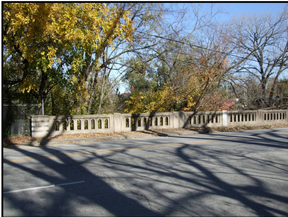
Figure 4.225 Spring Street Bridge over Beargrass Creek (JFCB-717).
