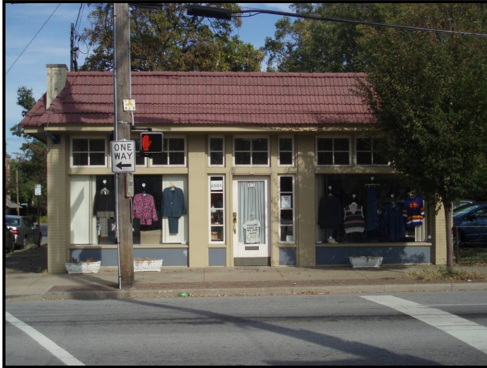
Figure 4. 68 Façade of 1501 Story Avenue (JFCB-382).
