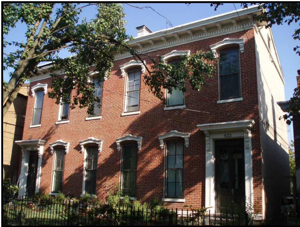
Figure 4.35 Façade of 831-833 East Washington Street (JFCB-79).
