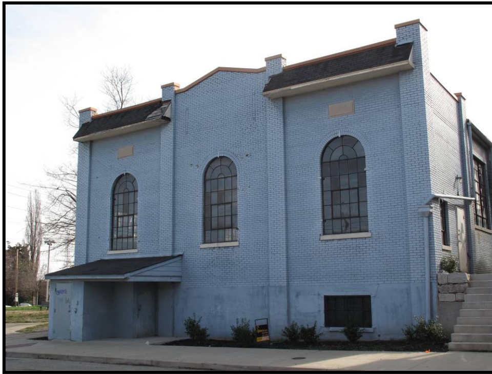
Figure 4. 133 121 North Shelby Street, Wesley House gymnasium (JFCB-623).
