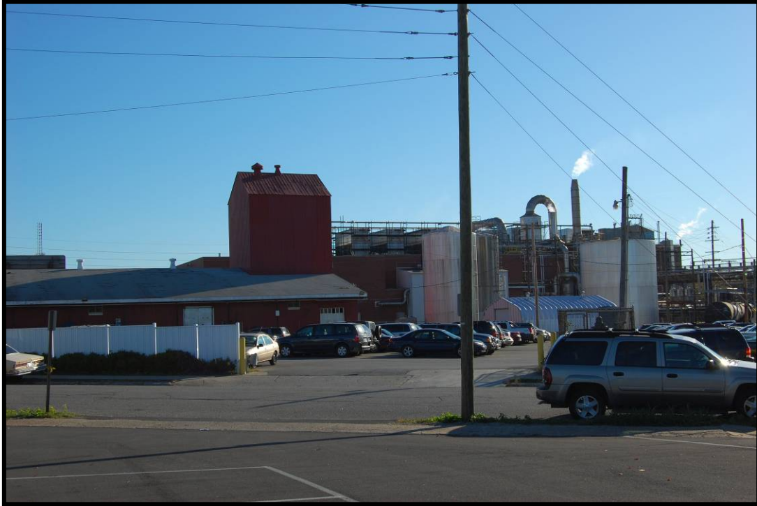
Figure 4. 174 JBS Swift Plant, looking southeast (JFCB-692).
