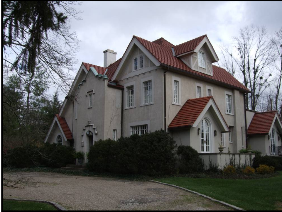
Figure 4. 57 Façade and west elevation of 26 River Hill Road (JF-2111).
