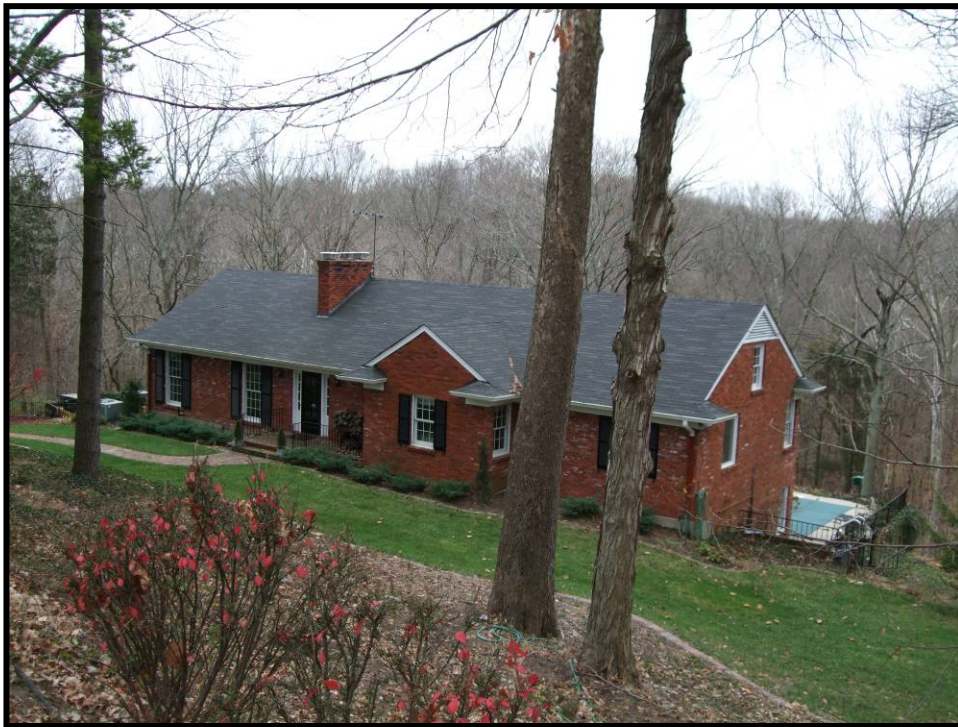
Figure 4. 63 Ranch house at 7428 Woodhill Valley Road (JF-2068).
