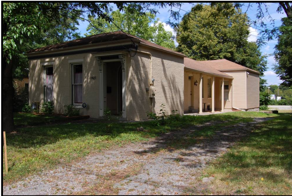
Figure 4. 28 Façade and east elevation (showing recessed side porch) of 1421 Quincy Street (JFCB-318).
