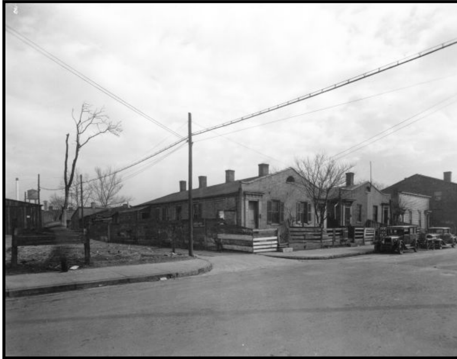
Figure 3.34 Photograph labeled “Housing in Phoenix Hill 1934.” The location is between Jefferson and Chestnut Streets and Jackson and Clay Streets. 492
