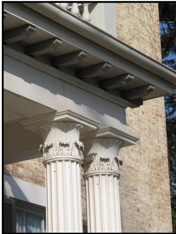
Figure 4. 5 Detail of the portico at Rosewell(JF-452).
