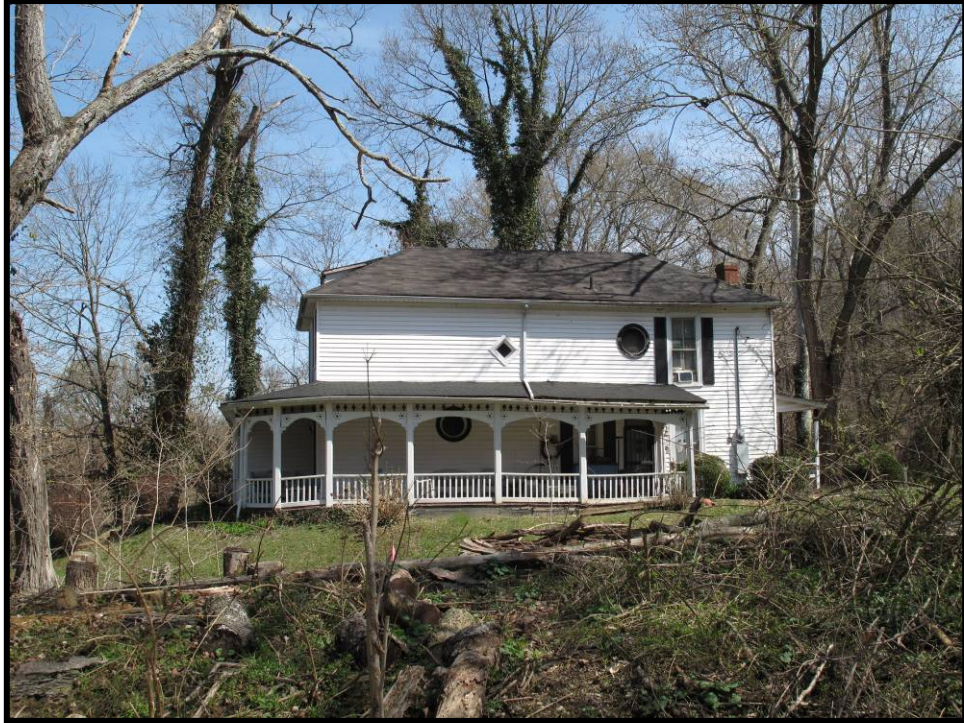
Figure 4. 122 Southwest elevation of Merriwether House, facing northeast (JF-690).
