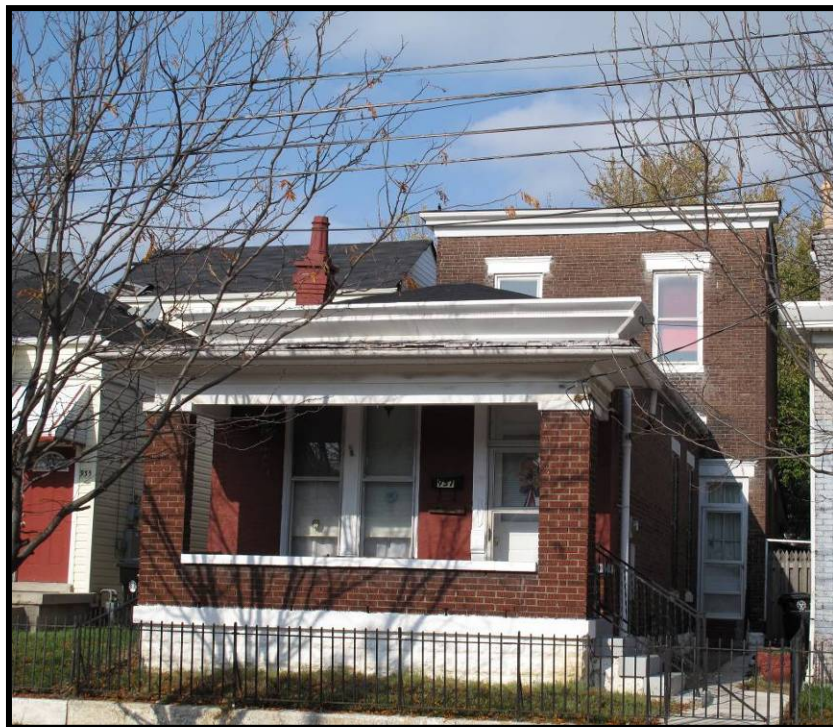
Figure 5. 14 Façade of 937 East Liberty Street (JFCH-1041), showing remodeled Craftsman porch.
