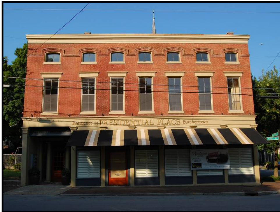
Figure 4. 74 Façade (Adams Street side) of the Gnau Store (JFCB-345).
