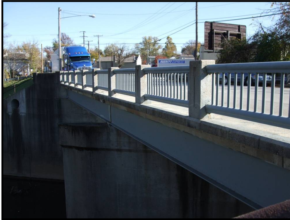
Figure 4. 226 Brownsboro Road Bridge over Beargrass Creek (JFCB-716).
