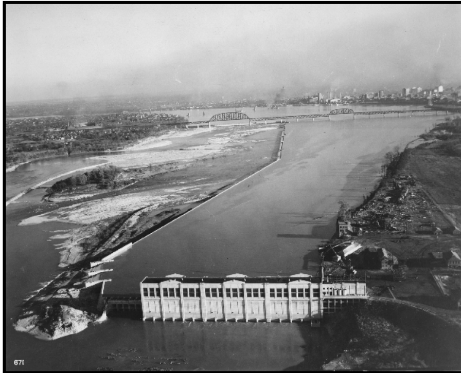
Figure 3. 30 Louisville Hydroelectric Power Plant, circa 1930. 459
