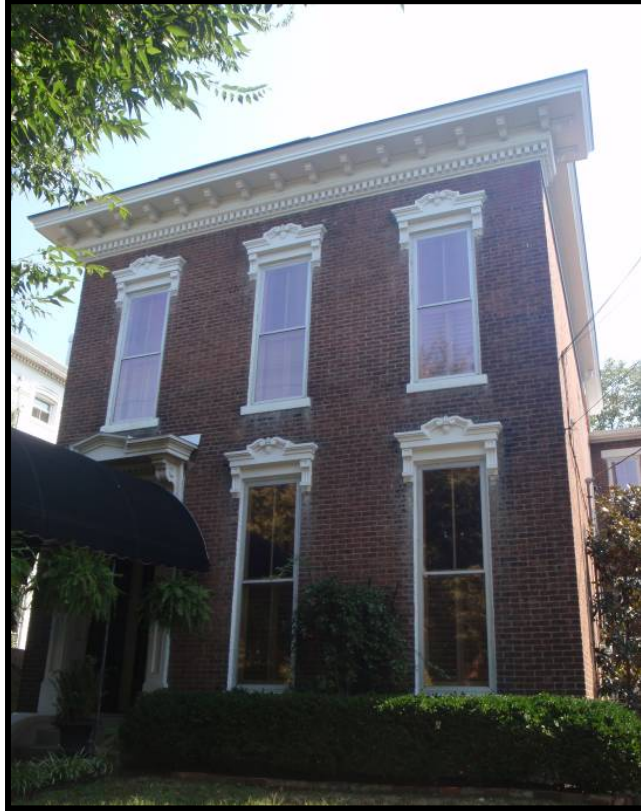
Figure 5. 7 Façade of 1618 Story Avenue (JFCB-443).
