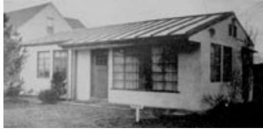
Above: A Steelcraft prefab house. All framing materials were either steel or aluminum. Interestingly, stucco was added as the exterior sheathing material. (Source: Prefabs on Parade ).
