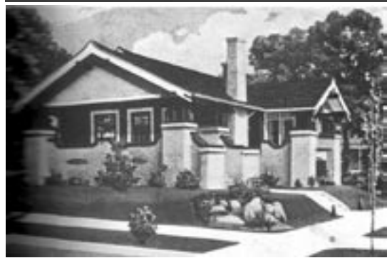
Above: Located at Madison and 16th Street, resource (MCNP-946) is located near the ICR railroad shops and may have been built to serve as worker housing. It closely resembles the Sears “ Osborn ” pictured below. The main difference is that the building appears to be reversed in its orientation. Further research and access to the house would confirm whether it is a precut house. (Source: Houses by Mail ).
