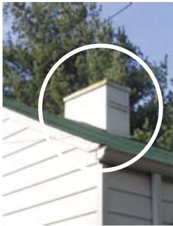
Above: Exterior details like porch railings and door hoods with wrought iron detailing are hallmarks of a Gunnison house. An other tell tale detail of a Gunnison house is the sheet metal chimney with horizontal vents.
