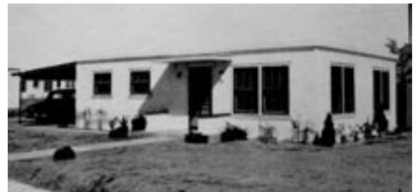
Above: A Le Tourneau prefab house that was produced at the site in a single pour of concrete cast in the “Tournalayer” machine. (Source: Prefabs on Parade ).
