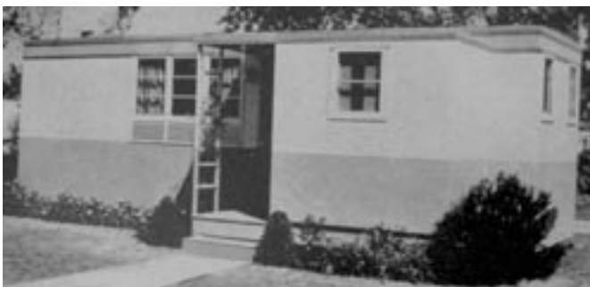
Above: A completely preassembled Wingfoot house ready for occupancy. (Source: Prefabs on Parade ).
