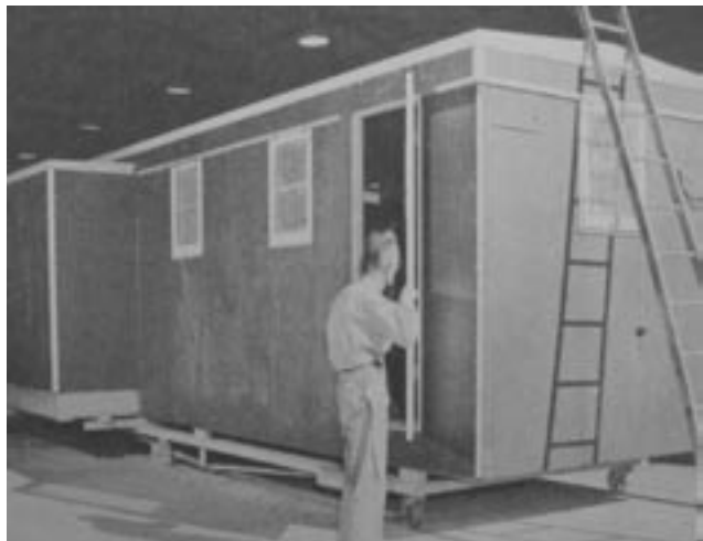
Sectional and preassembled prefab houses often came complete with wiring, plumbing, and appliances. By completely preparing the house before it arrived at the site, the prefab was ready for immediate occupation. (Source: The Prefabrication of Houses ).
