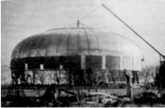
Above: Buckminster Fuller's Dymaxion House made of aluminum. Despite public interest in the innovative project, Fuller's prefab never was mass-produced. (Source: The Prefabrication of Houses ).
