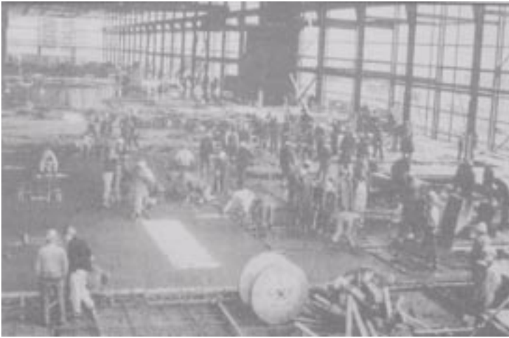
Inside the PDGP plant. The massive influx of workers for this plant and allied industries created a population boom in Paducah. (Source: "Cultural Resource Survey and National Register Assessment C140 Complex Paducah Gaseous Diffusion Plant McCracken County, Kentucky").
