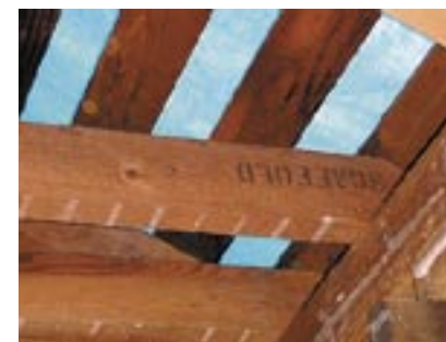
Left: A shipping label for a Sears house in Anderson County was found on the inside of a door frame. Right: Examples of stamped lumber. The top picture is from a Sears house which used numbers. The bottom picture is from a Gordon-Van Tine House, which has words stamped on the lumber identifying where it should be placed in the framing system. (Source: www.desertweyr.com).
