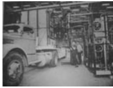
Above: Loading the Lustron materials onto a truck specially designed for the company. Materials were loaded to coordinate unloading with the assembly process on the site. (Source: The Prefabrication of Houses ).
