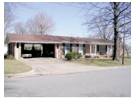
The original owners of this prefab house at 1353 Rudy Avenue, (MCNP-964) added the carport and brick veneer after its initial construction.
