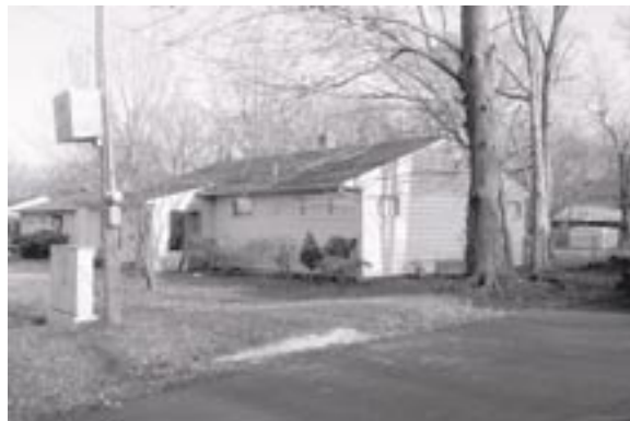
Above left: 108 14th Street (MLB-34). Above right: 200 14th Street (MLB-35). These houses may be panelized prefabs. They are small in form and have sheet metal chimneys.
