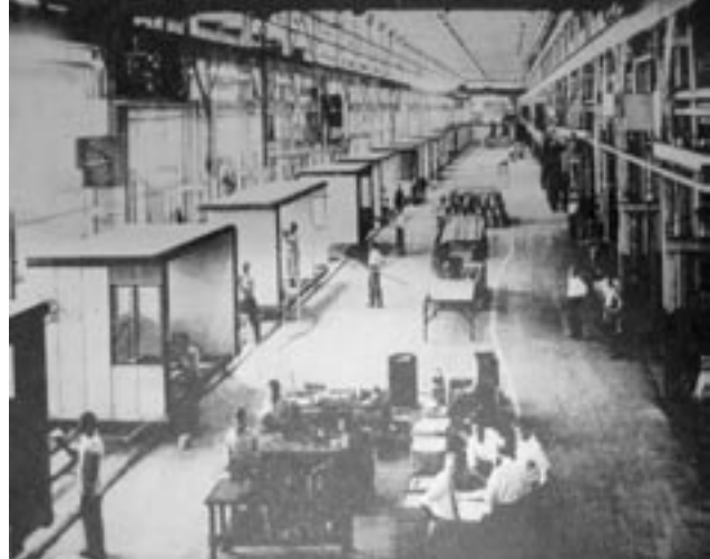
Assembling sectional prefab housing at the Reliance Factory. (Source: The Prefabrication of Houses ).
