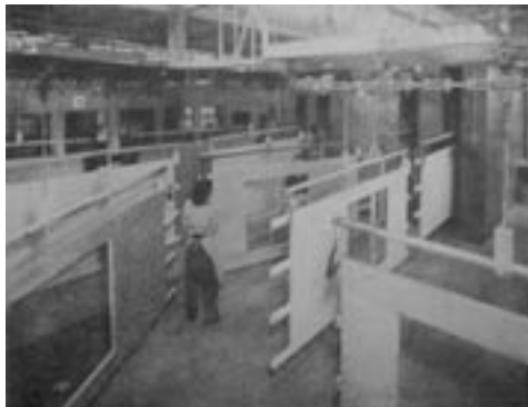
Above: Gunnison stressed skin panels fitted with window openings. By including windows and doors in panels, construction time at the site was reduced. (Source: The Prefabrication of Houses ).
