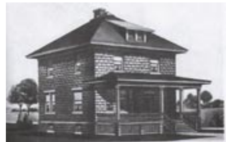
Sears House model no. 52 featured concrete block as its principal construction material. (Source: Houses by Mail ).
