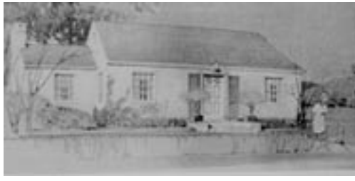
Above: A Cape Cod prefab house offered by the General Plywood Company. (Source: Prefabs on Parade ).
