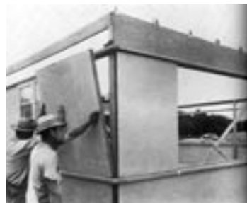
Right: Assembling a Cemsto House using solid panels in 4' by 4' modules. These panels served as both the interior and exterior wall surfaces. (Source: The Prefabricated of House ).
