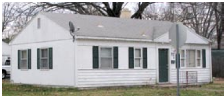
Above: A National house with exposed panels on the side elevation leaving a smooth surface.
