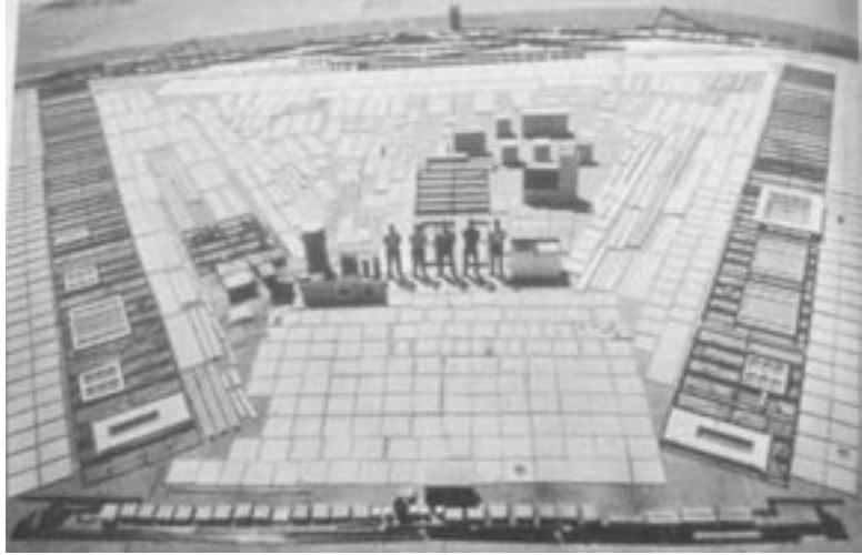
All of the parts needed to assemble a Lustron house are shown above. The porcelain-enameled steel panels and steel frame fit together to make the building envelope. (Source: The Lustron Home: The History of a Postwar Prefabricated Housing Experiment ).
