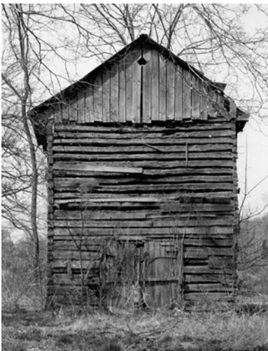
Flue-Cured Tobacco Barn, Log, Trigg County, Circa 1880. Although this barn was built in the late nineteenth century, its form and massing is much like earlier flue-cured tobacco barns.
