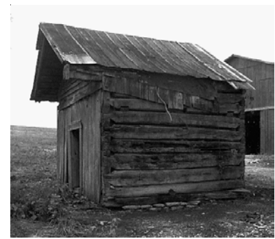
Log Meat- or Smokehouse, Jessamine County, Circa 1815-25. The overhanging gable is a common form for log outbuildings.
