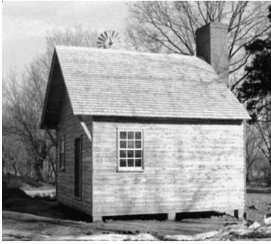
Kitchen: Riverside, The Farnsley-Moreman Landing, Jefferson County, 1999 reconstruction of circa 1835 building. The reconstruction is based upon archaeological evidence. Although it is sited behind a brick house, the kitchen was impermanent, resting on a foundation of posts set in the ground, which quickly began to rot. The original building fell into disuse after about 1865, and had been demolished by the late 1870's
