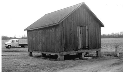
Granary, circa 1840-60, Oldham County. The building is elevated well above ground on a stone pier foundation.
