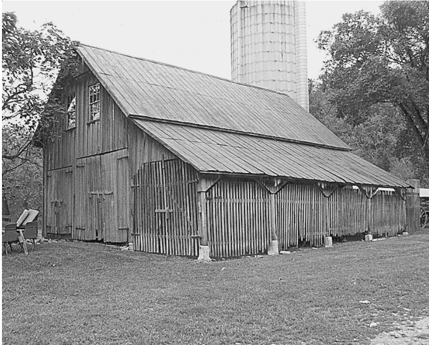
Carriage House and Granary, Hamilton Farm, Washington County, 1877. Constructed by Joseph Tong, who signed and dated the building on a wooden beam. The original barn, to the left, has two long aisles. The aisle to the right was used for carriages; the aisle to the left is divided into storage areas for tack and tools. The second floor loft was used for hay and grain storage. The shed to the right is a later addition for further carriage and machine storage.
