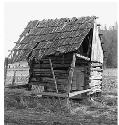
Corn Crib, Circa 1880-1900, Metcalfe County. Note the similarity of the form, single pen with covered side drive, to the crib at the Darius Downing Farm, above.
