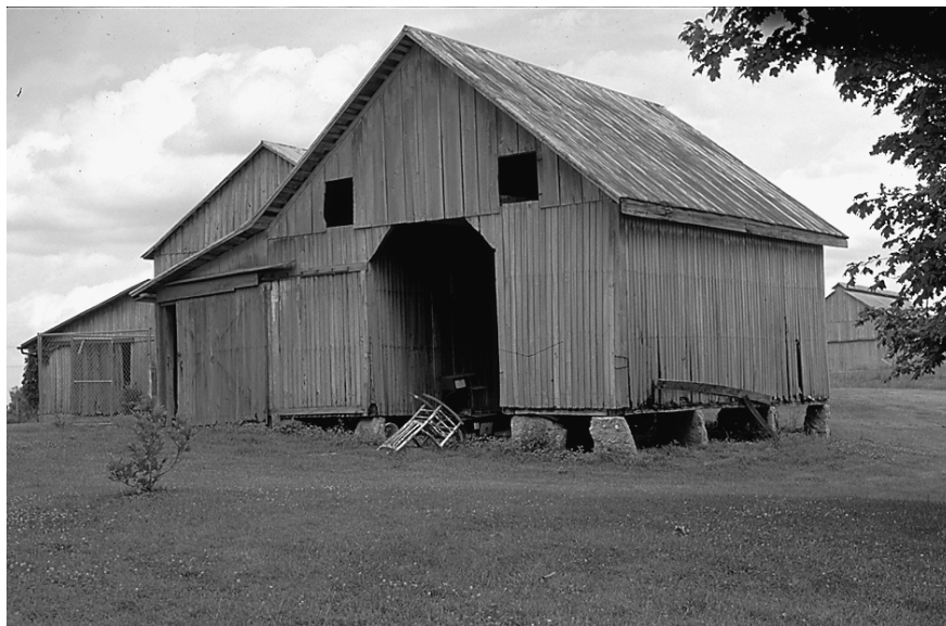
Corn Crib, Circa 1880-1900, Metcalfe County. Note the similarity of the form, single pen with covered side drive, to the crib at the Darius Downing Farm, above.
