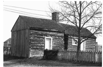
Saddlebag Slave House, Circa 1810 and 1840, Homeplace Farm, Woodford County. This structure began as a single pen log house on the left. It was probably the original dwelling of the farmer who later built a fashionable brick house. The log house was then expanded by adding a second pen - larger, but not as well finished - on the other side of the chimney.
