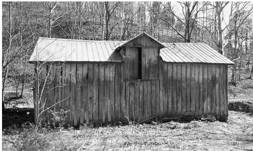
Sheep Barn, Hamilton Farm, Washington County, Circa 1900-10. This sheep barn looks much like a stable for larger cattle, except it is scaled for sheep.
