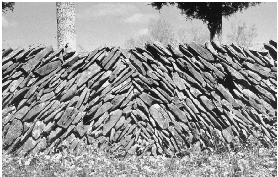
Edge Fence, Outer Bluegrass Region, 1850-75. Edge fences are most often found in the hilly areas of the Outer Bluegrass region.
