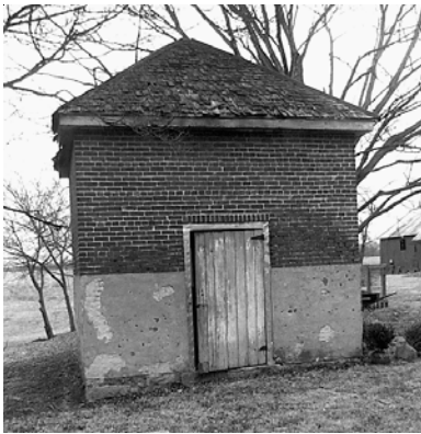
Smokehouse, circa 1830, Pine Grove Stock Farm, Oldham County. A substantial brick smokehouse with pyramidal roof, of a fairly typical size and shape. This smokehouse is on an upscale farm. Below, a rare example of a round smokehouse, Bardstown, circa 1820.
