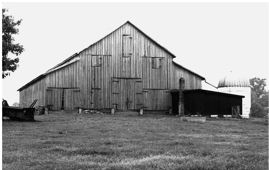
Air-cured Tobacco Barn, Frame, Bourbon County, 1860-1870. This aisled barn has attached sheds, probably for cart or machine storage.
