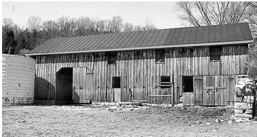
Stock Barn, Hamilton Farm, Washington County, Circa 1865. The Hamilton Farm Stock Barn is a modified English bank barn with a cross aisle accessed through double doors. The unique plan includes two drive-throughs, joined by a cross-aisle, which is flanked by stalls. The drive-throughs have hay racks on one wall (left). On the other side of the left drive are a couple of grain storage rooms. Hay is kept in the loft above. Given the barn's unusual design and Alexander Hamilton's interest in scientific agriculture, it is probable that he chose this barn's design from an agricultural improvement journals
