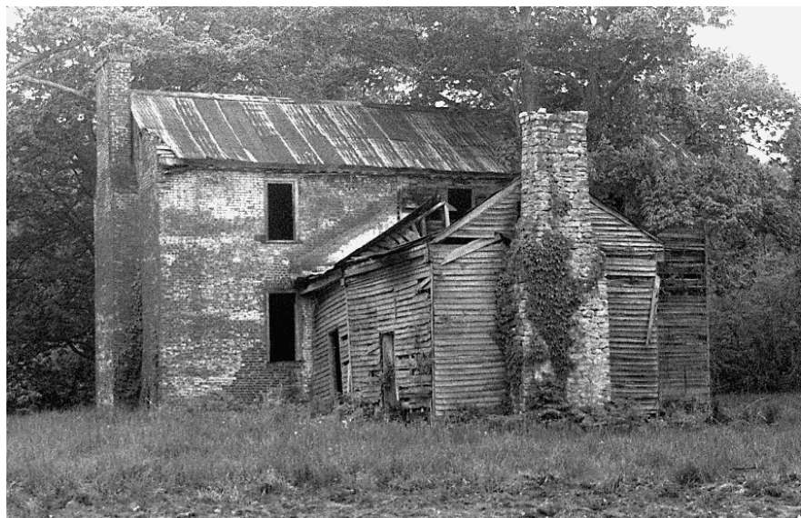
By the 1860's, detached kitchens began to be appended to the rear of the main house. Following the trend in new construction, in which the kitchen would be located in an ell at the back of the house, the builder would join the two structures through an open breezeway or enclosed passage. This occurred at the Hardin House in Owen County, above and right, when the 1830's log kitchen was attached to the house around 1870.
