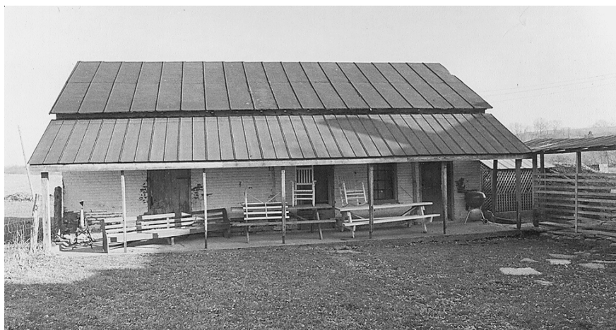
Backhouse, Hamilton Farm, Washington County, Circa 1810-30. This backhouse combines a smokehouse and an unheated room with good window light. This room may have been used for such tasks as spinning, weaving, and food processing. A loft overhead may have been used as for living space or storage.
