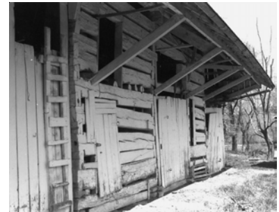
Log Stable, Shelby County, Circa 1820-30. More substantial than the simple rail pen, the hewn log barn was a common site in early Kentucky. These barns usually served many functions, including storage of crops and carriages.
