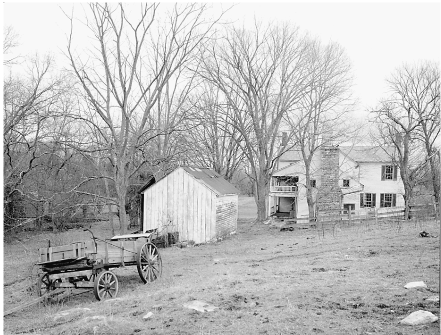
William Guyn House, Woodford County, Circa 1820-45. The oldest part of this house, the ell, dates from circa 1820. The kitchen, a single story section at the very back, was added to the end of this two-story log house around 1825-30. The front section, a fashionable frame house in the Greek Revival Style, was added about 1845, effectively converting the original house into an ell. The rooms in the original house, once living areas, were relegated to work space. Photograph by Jet Lowe, HABS.
