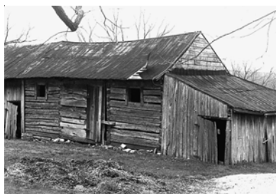
Double-pen Log Barn, Fayette County, Circa 1820. A variation on the English barn, the double-pen log barn, has a log crib located on each side of a central aisle in the manner of a dogtrot house. The form could serve a number of purposes, from hay storage to animal stableage. Frequently, its use changed as farming needs were altered.
