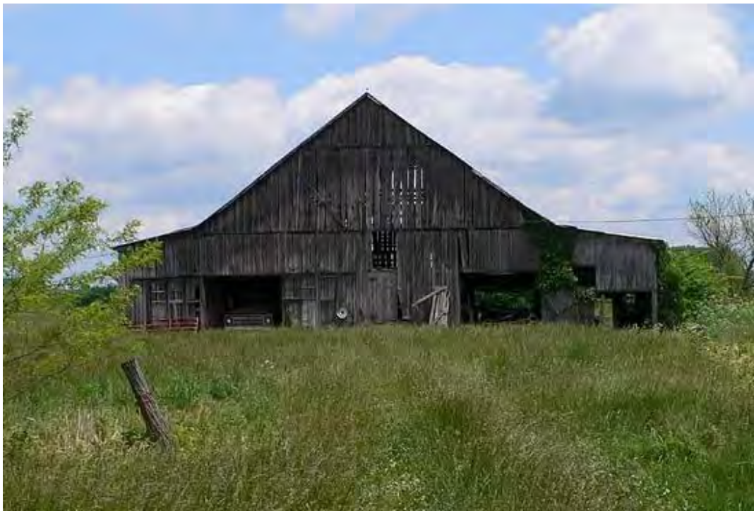
Figure 240: MN 685, Multi-purpose Barn, late nineteenth-early twentieth century, Gravel Switch vicinity. See also Figure 255.
