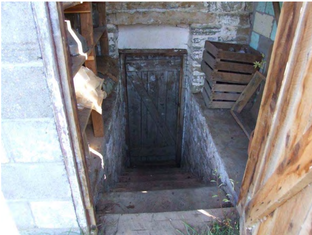
Figure 199: MN 205, view inside Entry Shed.
