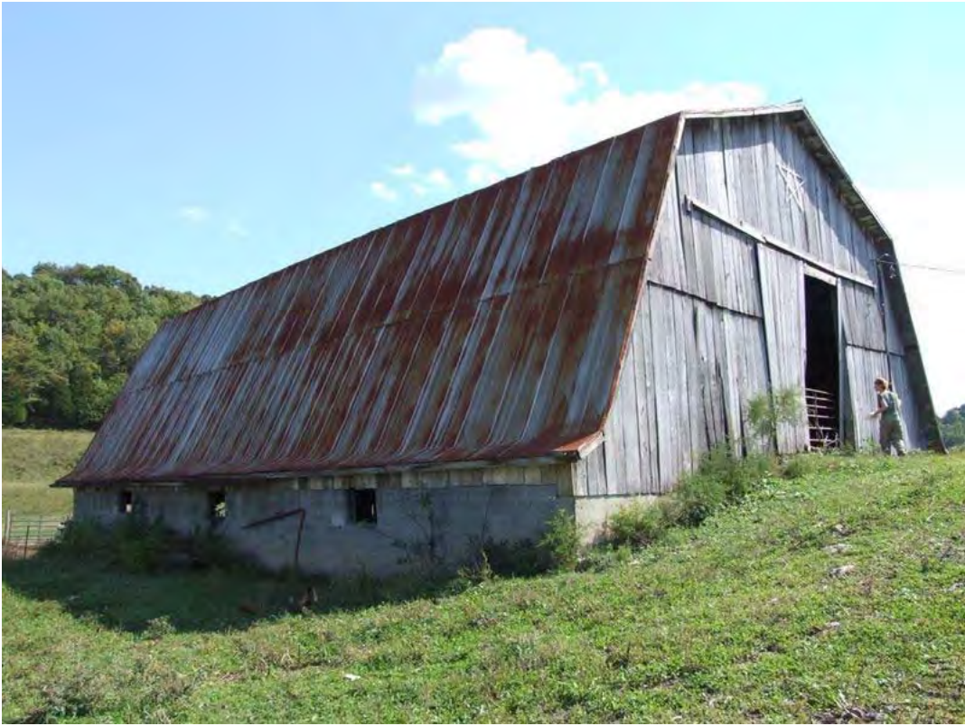
Figure 272: WS 98 Dairy Barn, 3/4 view. See also Figure 271 and Figure 273.
