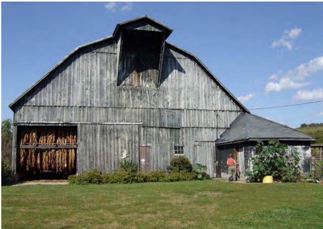
Figure 277: WS 317, Transverse Frame Gambrel Roof Dairy Barn, now used for tobacco; early twentieth century, Fredericktown vicinity. The interior has stalls, milking, and feeding areas with a concrete trough, with a hay loft overhead. The extension at front right is a concrete block milk room. The barn is connected, via a board and batten section, to a concrete stave silo not visible here.
