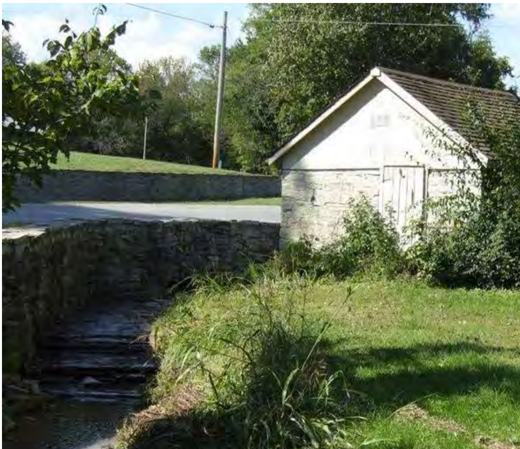
Figure 201: WS 317, Springhouse, early-mid- nineteenth century, Fredericktown vicinity.
