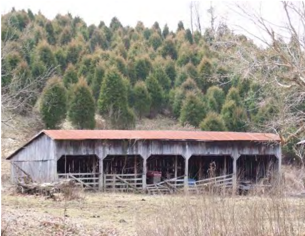
Figure 319: WS 579, Machine Shed, early-mid twentieth century, Texas Vicinity.
