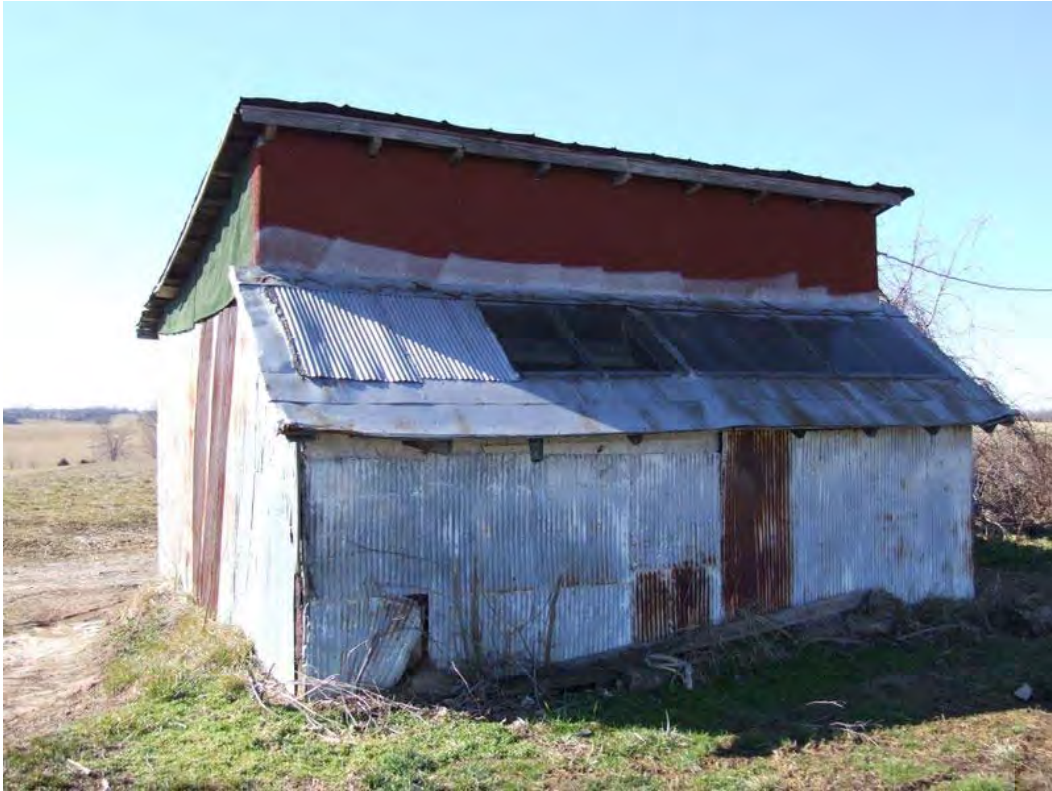
Figure 287: WS 590, Detached Stripping Shed, mid twentieth century, Jenkinsville vicinity.
