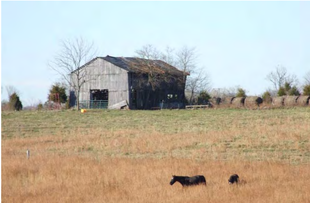
Figure 235: MN 217, Tobacco Barn, mid twentieth century, Holy Cross vicinity.
