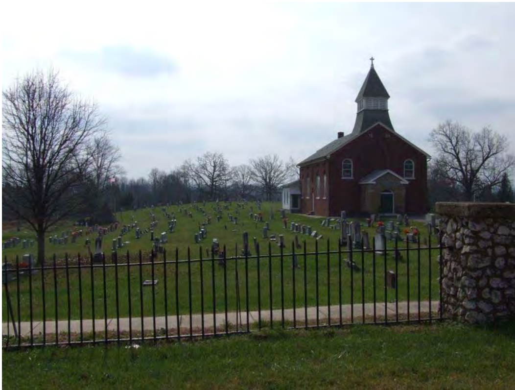
Figure 330: MN 13, Holy Cross Catholic Church, 1824.
