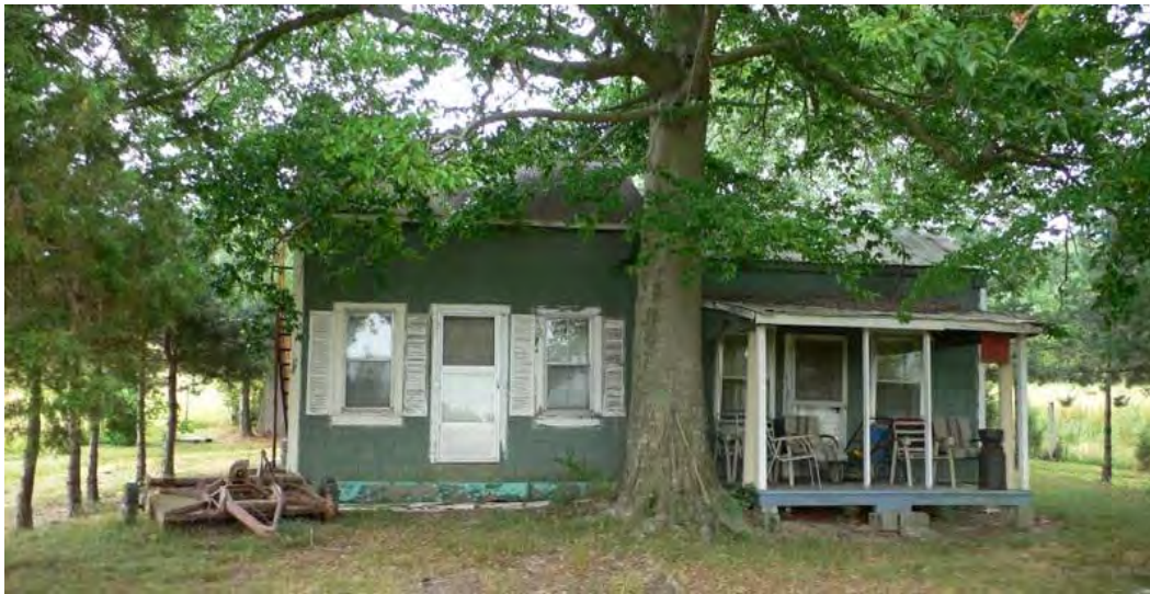
Figure 138: MN 925, saddlebag log and frame house, mid-late nineteenth century, Bradfordsville vicinity. The right side is log, the left side is later frame added to the chimney end of the log house.
