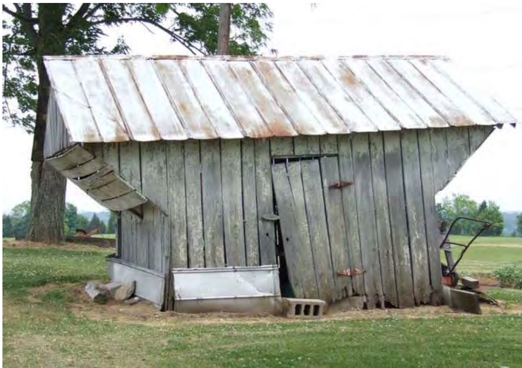
Figure 291: WS 931, Frame Chicken House , early twentieth century, Willisburg. This type of chicken house with cantilevered bays is a standard form in the twentieth century. The undersides of the bays are slatted to allow manure to sift through so that it could be collected underneath.
