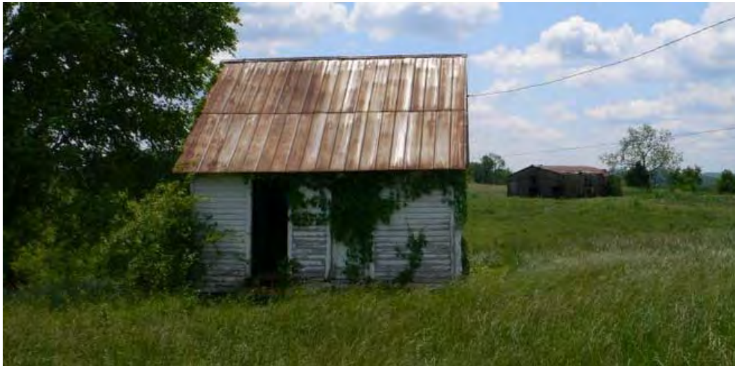
Figure 150: MN 685, Polly's house, a documented tenant house, has two doors with a single pen plan, but may have once been narrowly divided into two rooms on the ground floor. Ladder to the loft is near left hand door. Late nineteenth-early twentieth century, Gravel Switch vicinity. See also Figure 151.
