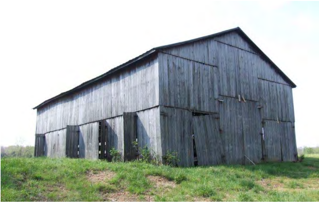
Figure 285: MN 515, Frame Tobacco Barn, mid-late twentieth century, Raywick vicinity.
