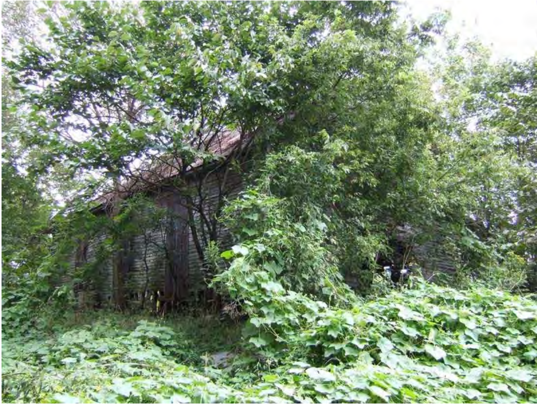
Figure 339: WS 263, Maud Methodist Church, late nineteenth-early twentieth century.
