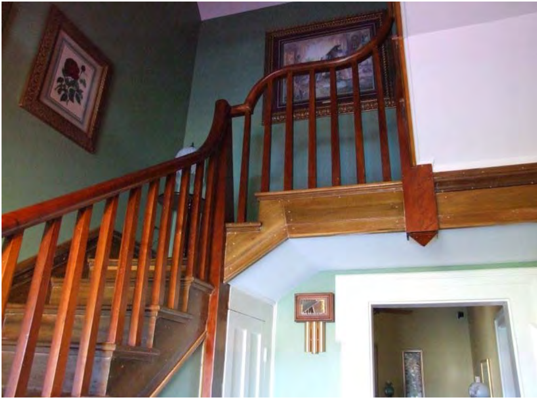
Figure 30: MN 336, “Old Loretto Farm” House, mid-nineteenth century, Loretto, stair detail. Stylistic details in this house have elements of Federal, Greek Revival, Gothic, and Italianate styles. See also Figure 31.
