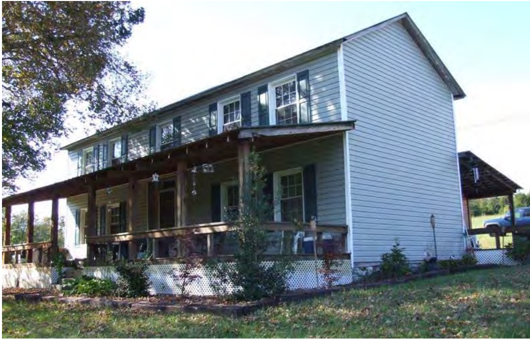
Figure 155: WS 301, early nineteenth century, Booker vicinity. This house is built in a dogtrot fashion with the space between the two pens serving as the entry hall.
