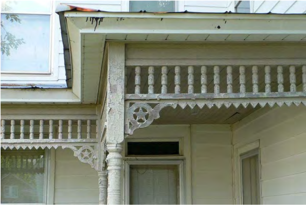
Figure 86: MN 930, Porch ornamented with sawn and turned elements, late nineteenth century, Bradfordsville.
