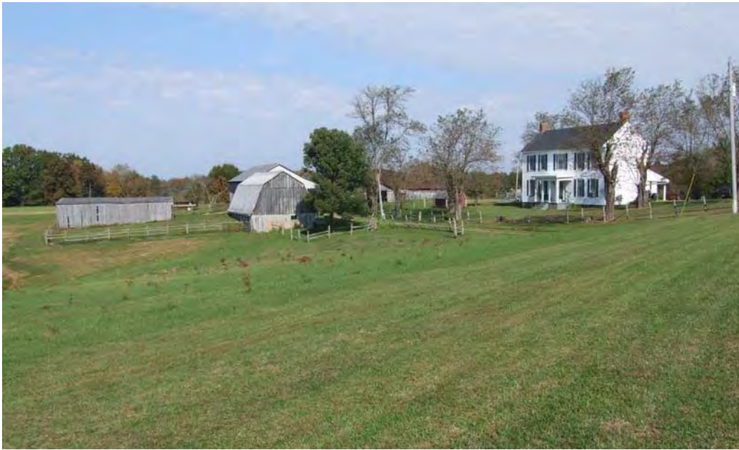
Figure 347: WS 85, James Grigsby farm, Mooresville vicinity. The oldest part of the house is an early nineteenth century log section located in the ell behind the frame front section seen here. The gambrel roof barn left center is a banked dairy barn with a milking parlor and milk room on the ground level and hay storage above. Other outbuildings include a tobacco/multi-purpose barn, corn crib, smokehouse, machine shed, and garage.
