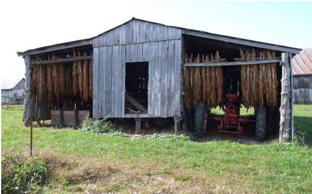
Figure 300: WS 85, Frame Corn Crib, early-mid twentieth century, with side sheds being used to hang tobacco and shelter farm machinery, Mooresville vicinity.
