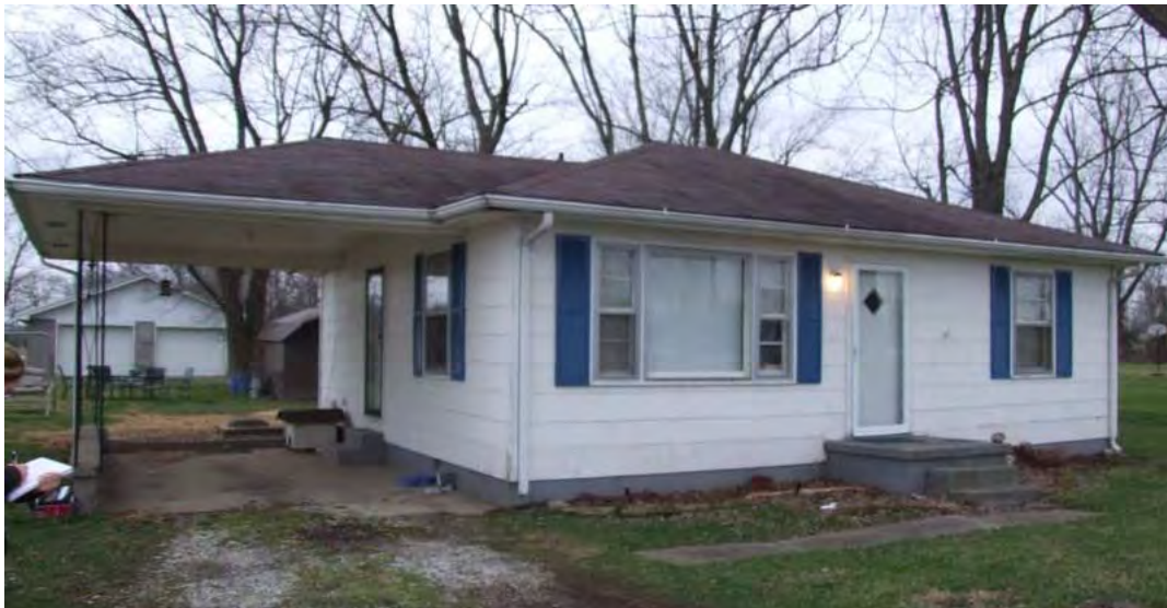
Figure 227: MN 432, Ranch style House with attached Carport, 1940s-50s, Loretto.
