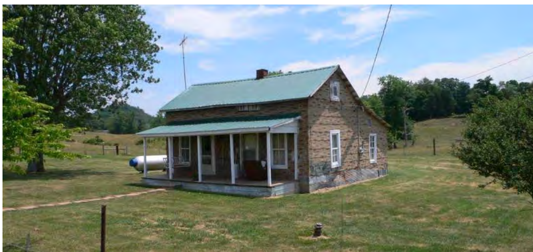
Figure 140: MN 963. Vertical Board frame double pen house with brick-patterned asphalt siding, late nineteenth-early twentieth century, Gravel Switch vicinity.
