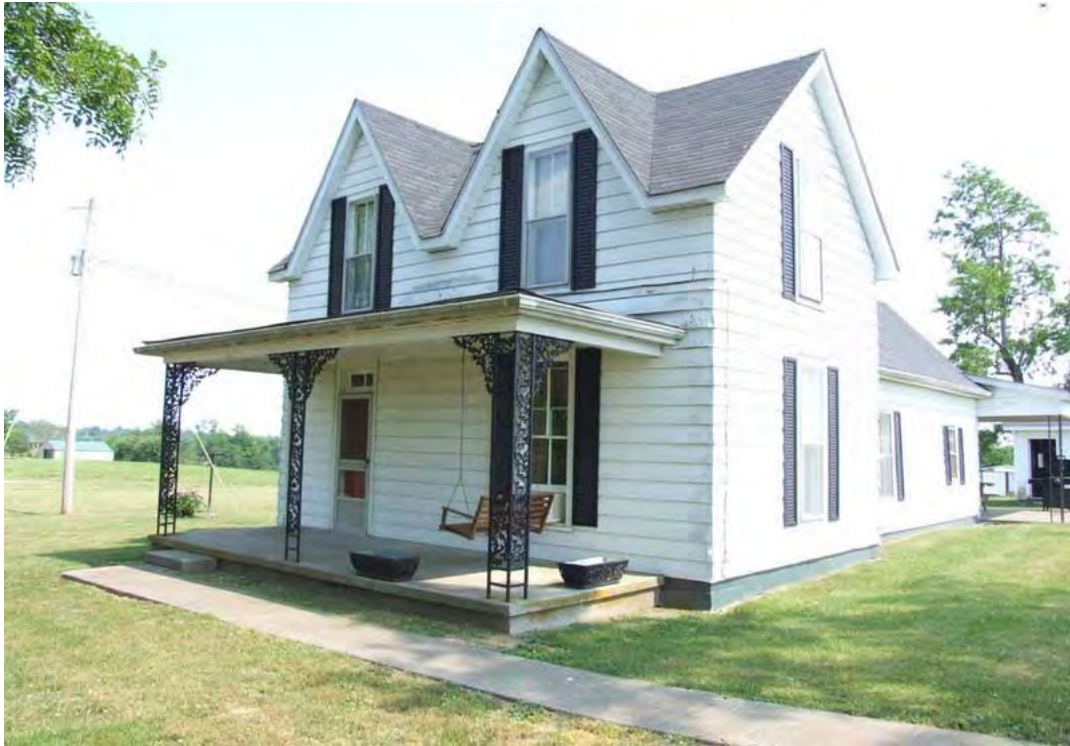
Figure 59: WS 869, late nineteenth-early twentieth century, Springfield vicinity.
