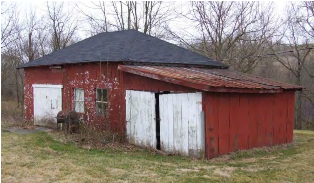
Figure 229: WS 556 Garage/Gas Station, mid twentieth century, Pottsville vicinity.
