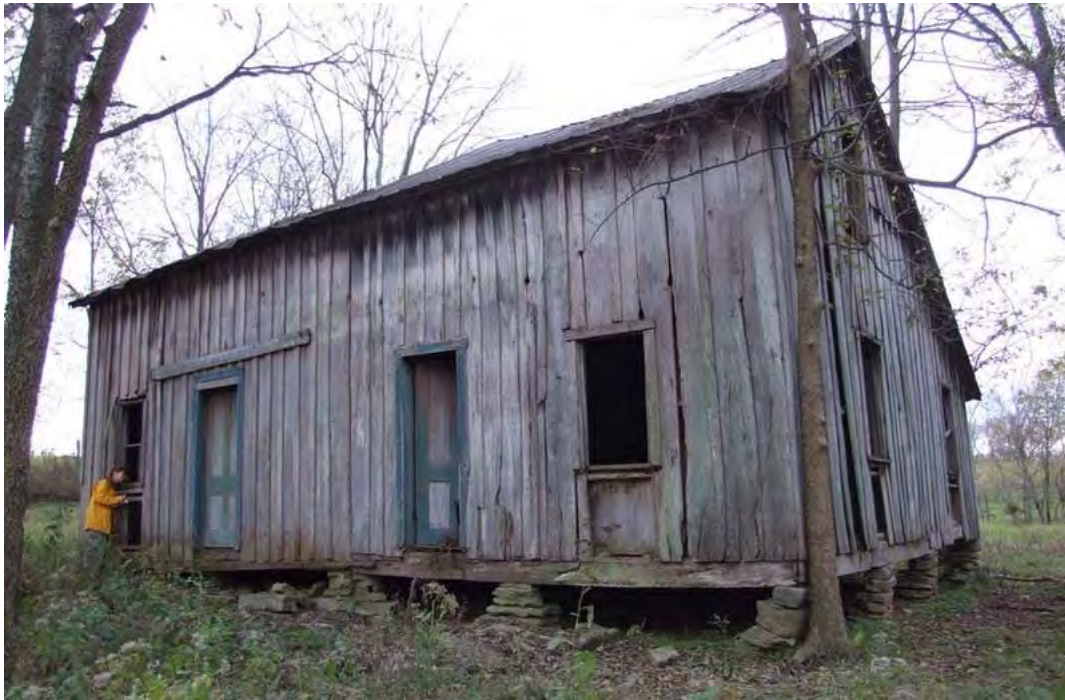
Figure 142: WS 431, Late nineteenth-early twentieth century, Valley Hill vicinity. House began as a single pen on the right but was later expanded into a double pen house.
