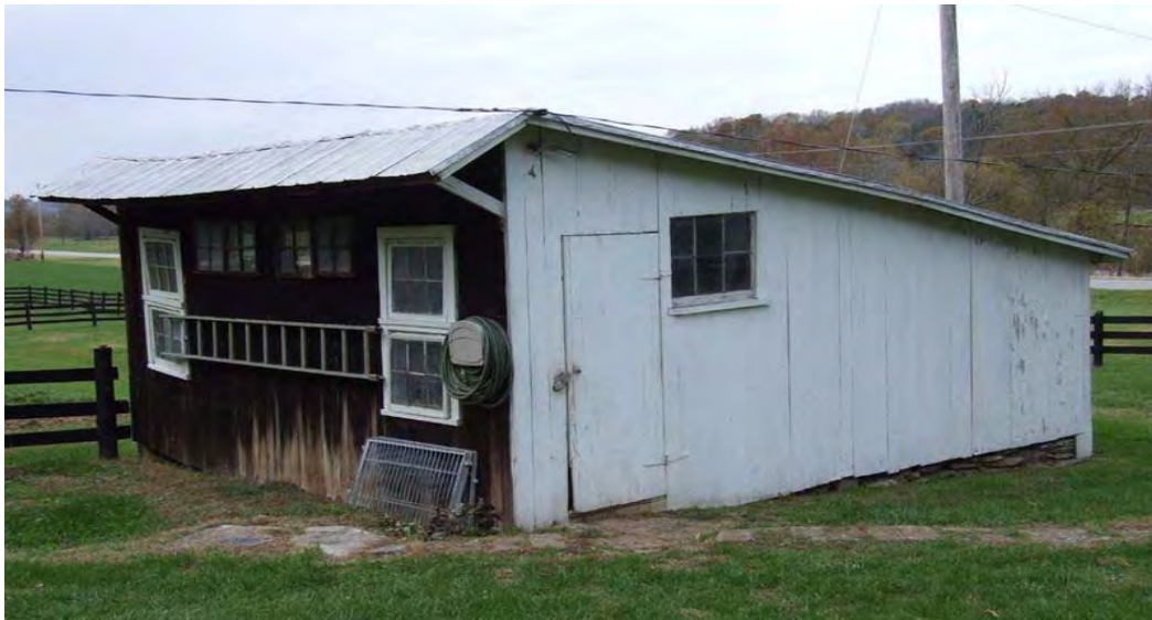
Figure 295: WS 416 Eugene Mudd's Chicken House, 1939, Fredericktown vicinity. According to the current owner, Mr. Mudd's son, Tom, the house was built from plans obtained from the Agricultural Extension Agency, compare to the "Laying House Plan" in Figure 294.
