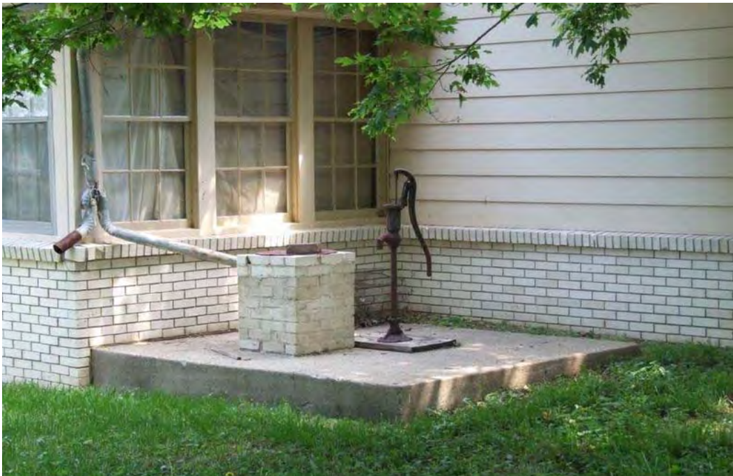
Figure 232: WS 877, Cistern with Pump, Ward House, 1930s, Springfield vicinity.
