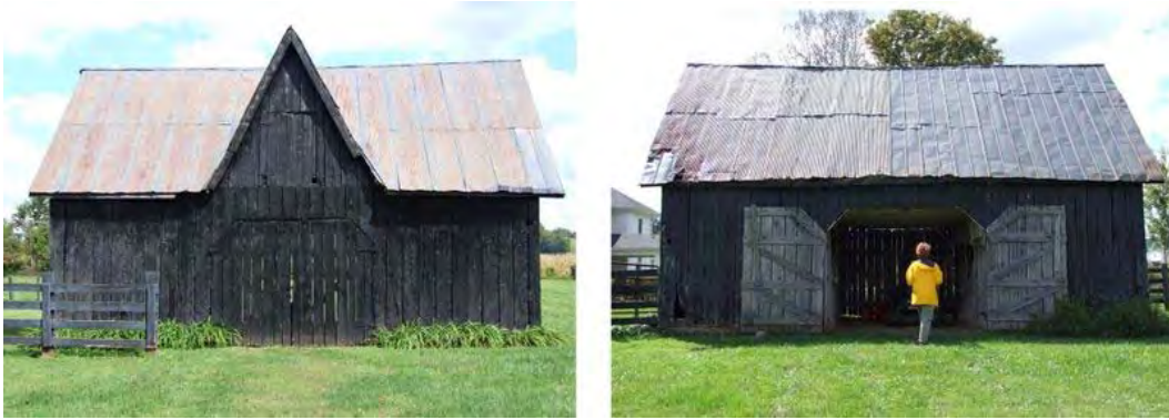
Figure 262: WS 33, Stock Barn, with stables, hay, and grain storage inside, late nineteenth century, Maud. Front of barn at left, back at right. An English barn type with a Gothic cross gable.
