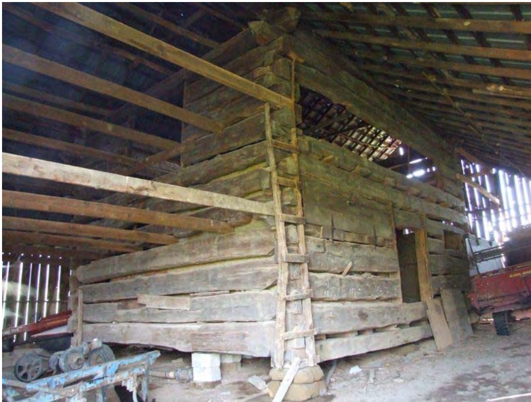
Figure 244: MN 514, Interior. See also Figure 243.
