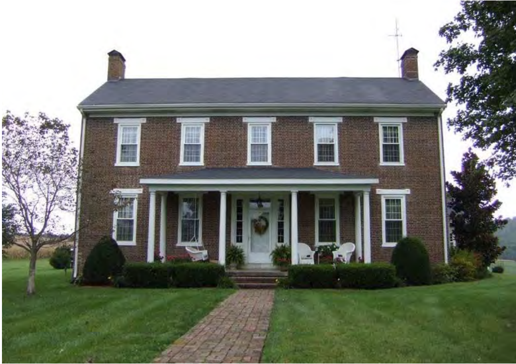
Figure 27: WS 27, Benjamin Pile House, Maud vicinity.
