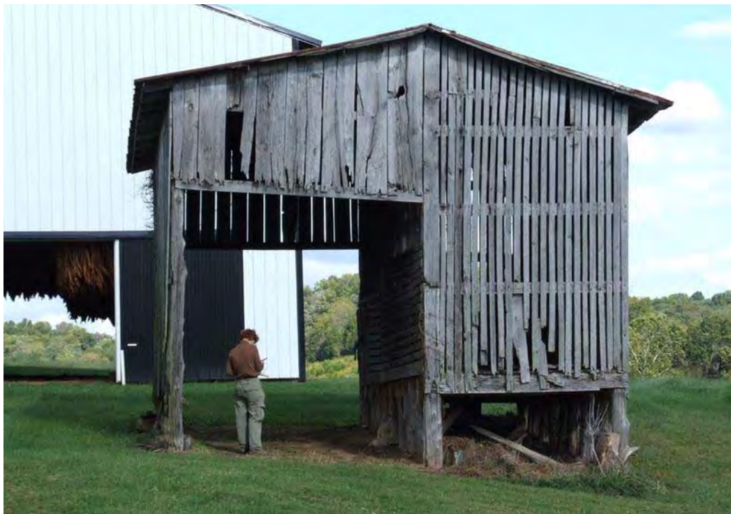
Figure 301: WS 278, Side Drive Corn Crib, early-mid twentieth century, Maud vicinity.
