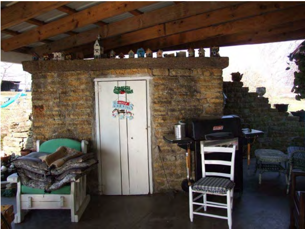
Figure 195: MN 273, Cellar, ca 1860-1900, Holy Cross. The roof overhead is a recent addition.
