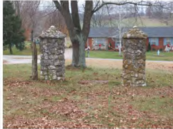
These are the entrance posts (made of coral heads) to Smock's Chapel. They are located to the front.
