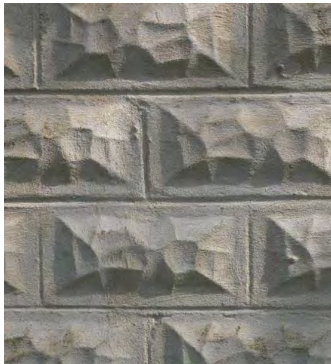
Figure 21: MN 672, Stone-faced Concrete Block House, mid 20 th century, Gravel Switch vicinity, detail.
