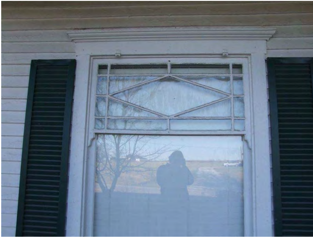
Figure 84: MN 384, detail of front window. See also Figure 83.
