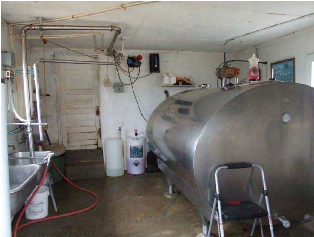
Figure 279: WS 407, Milkhouse, interior view, late twentieth century, Mooresville vicinity.
