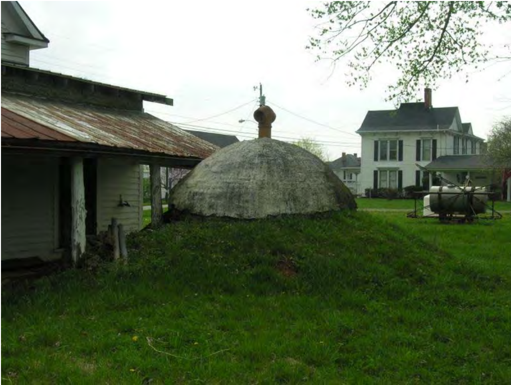
Figure 192: WS 171, Brick- domed Root Cellar, behind the John Harmon house, late nineteenth century, Mackville.
