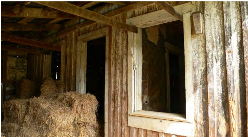
Figure 133: MN 920, Hall/Parlor house, nineteenth-early twentieth century, Gravel Switch vicinity: detail of front (covered by a later shed). The interior wall visible through the window divides the interior space of this house into two unequal size rooms. Dividing one of the two rooms with a wall results in a three-room plan.
