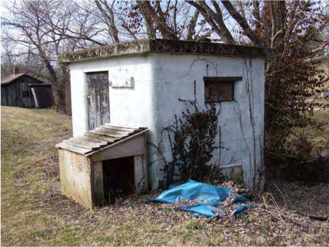
Figure 203: WS 579, Springhouse, early-mid twentieth century, Texas vicinity.
