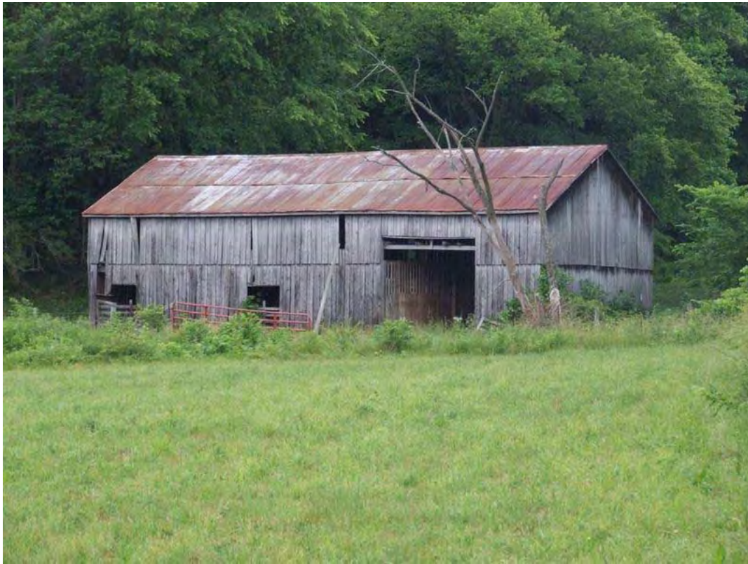
Figure 238: MN 715, Stock or Multi-purpose Barn, twentieth century, Jessietown vicinity.
