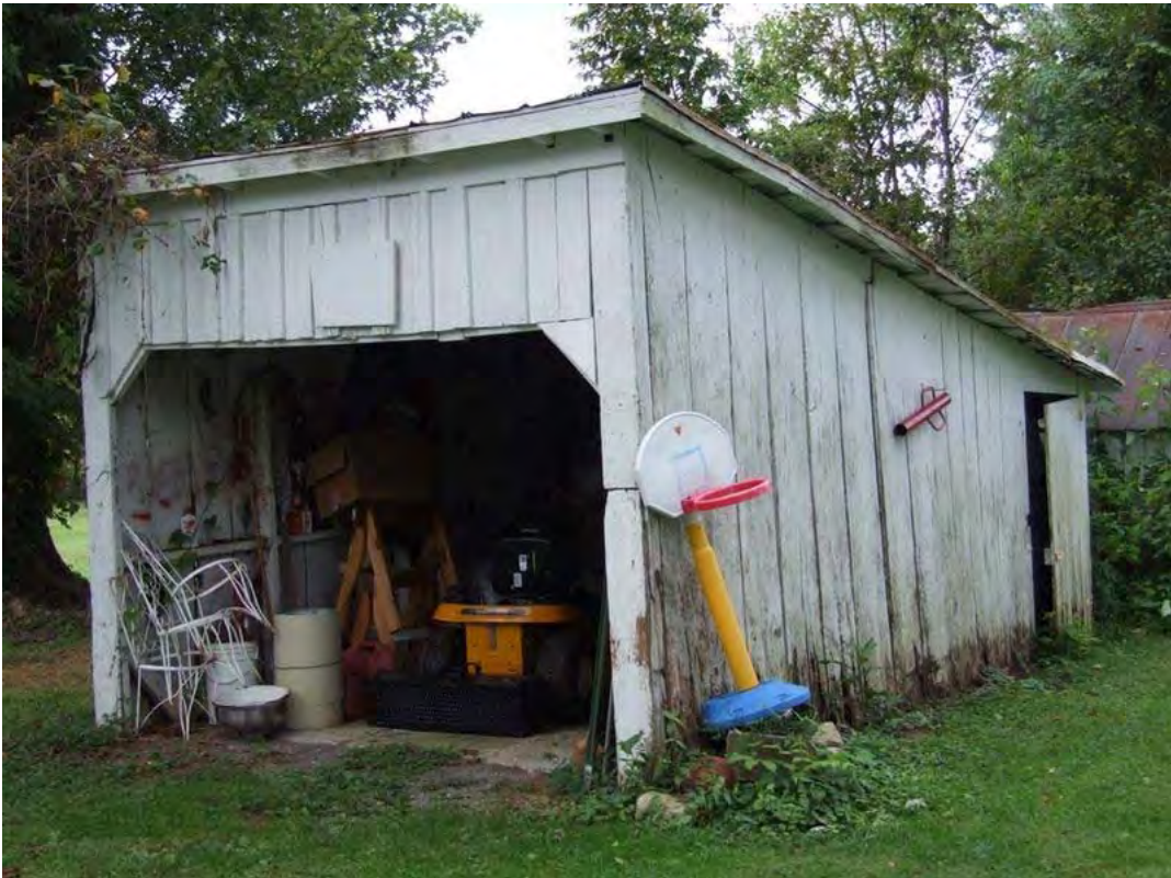
Figure 225: WS 270, Early-mid twentieth century frame Shed Garage, Maud.
