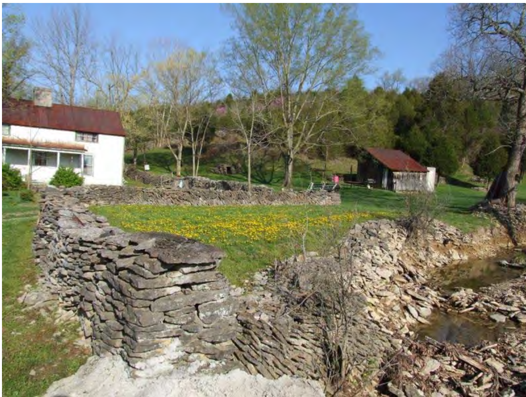
Figure 345: WS 720, Stone Fencing surrounding house. See also Figure 344 and Figure 346.
