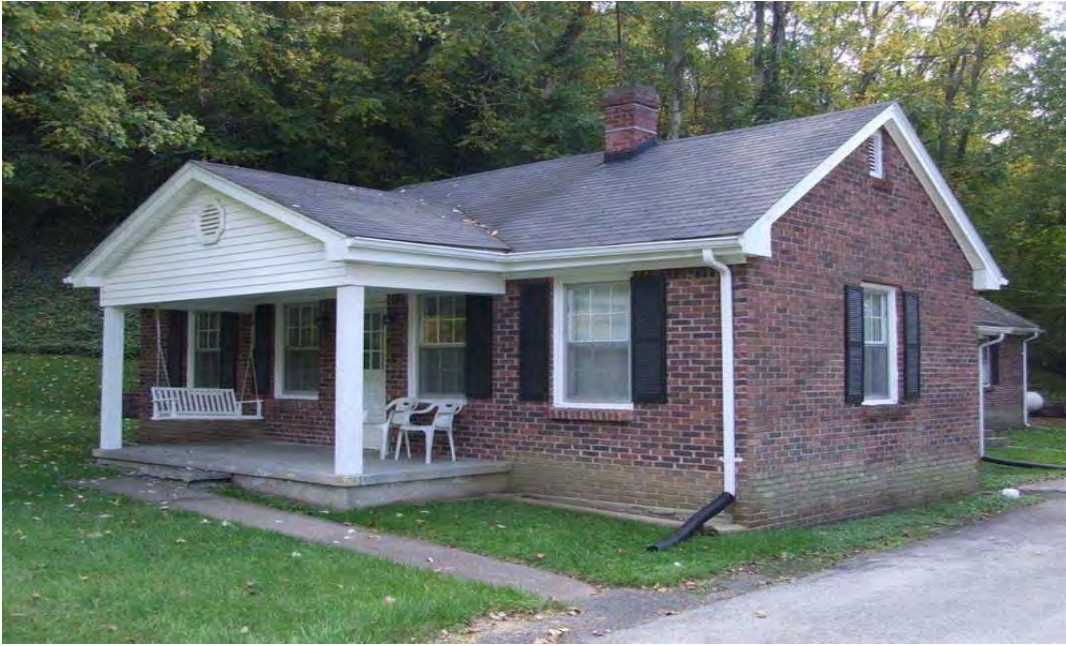
Figure 100: WS 350. At some later time after the move from Fort Knox, this house had a front porch added and was completely encased in brick, probably in the 1960s or 70s. This has had the effect of giving the structure over almost completely to Colonial Revival style, and giving it something of the appearance of a Ranch house, although it retains its basic center door, five bay form. The two houses share a common double garage, built in 1949 (Figure 101).
