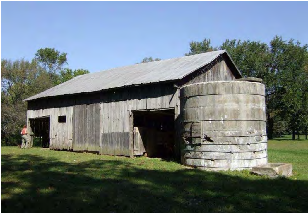
Figure 237: WS 315, Multi-purpose Barn, early-mid twentieth century, Fredericktown vicinity. A modified English barn with extended end sections for storage of farm machinery. The central section has stables, and hay was stored in the loft. The concrete structure in the foreground is a cistern.
