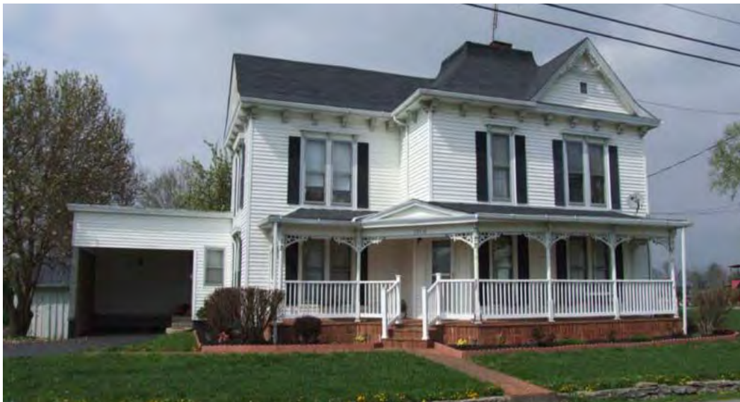
Figure 76: WS 172, John Harmon house, late nineteenth century, Mackville.
