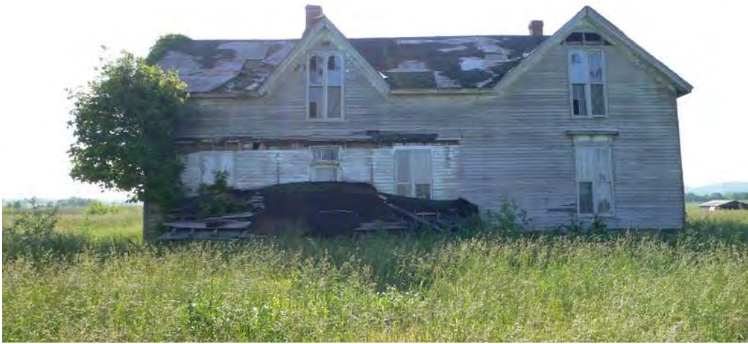
Figure 54: MN 688, side view. See also Figure 53, Figure 77, and Figure 80
