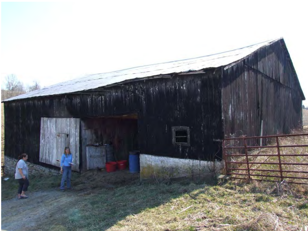
Figure 242: WS 633, Stock Barn, uphill side. See also Figure 241.
