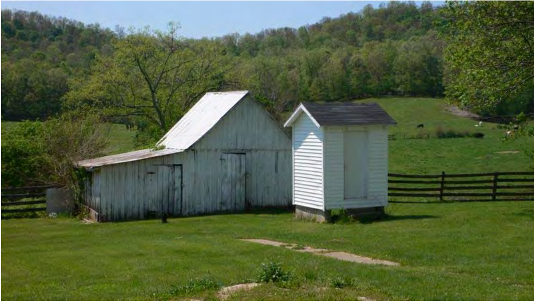
Figure 188, MN 681, Sweazy-Kirkland farm, Privy (front) and Gable-front Outbuilding, early twentieth century, Gravel Switch vicinity.
