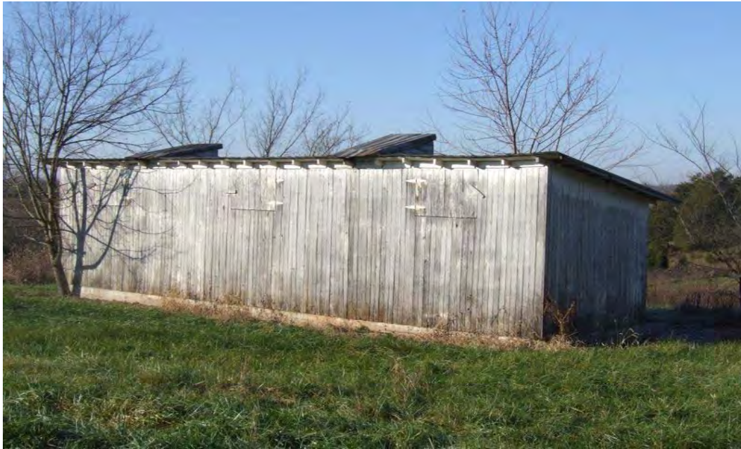
Figure 296: MN 193, Poultry House, 1930s-40s, near Terrapin Run. The roof has two dormer vents.
