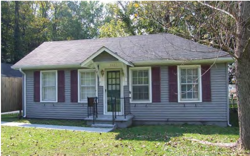
Figure 99: WS 349 & 350 (Figure 100), 1930s-1950s, Fredericktown. These two houses were both moved to this location from Fort Knox after World War II in the late 1940s by Colonel Everett Mudd. The structures were apparently built for housing for the War effort at Fort Knox, and then surplused after the war. WS 349 appears much as it did during its tenure at Fort Knox: a utilitarian structure with some elements of Colonial Revival and Arts and Crafts styling. Its neighbor, WS 350, below, is just barely recognizable as a related structure.
