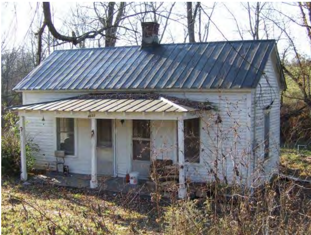
Figure 109: WS 453, Heel house, 1938-39. The house is said to have been built with lumber salvaged from a single room schoolhouse, which may account for its having the appearance of being older stylistically than its construction date would suggest. The 3/1 sash windows and the exposed porch rafter tails are consistent with the late 1930s.
