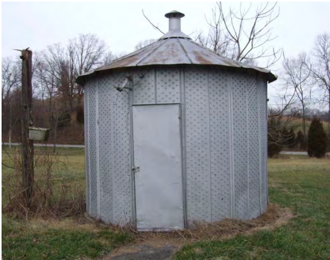
Figure 308: MN 320, Peterson Farm: mid twentieth century prefabricated metal Corn Crib, Dant vicinity.
