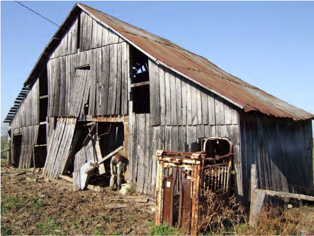
Figure 250: WS 451, exterior. See also Figure 248.
