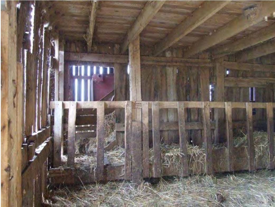
Figure 264: MN 749, Stables, Lebanon vicinity, interior. See also Figure 263.
