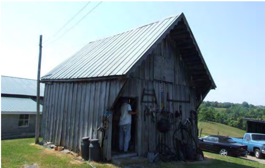
Figure 207: WS 849, Meathouse, late nineteenth century, Willisburg/Brush Grove vicinity. The steep, Gothic style gable and board and batten siding are notable features.
