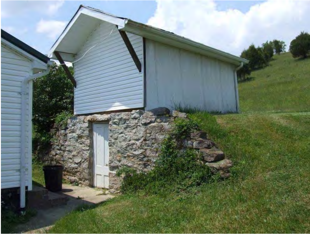
Figure 200: WS 812, Stone-lined Cellar with frame Dry Storage Structure above, late nineteenth-early twentieth century, Tathum Springs vicinity. The upper level is accessed by a door in back.
