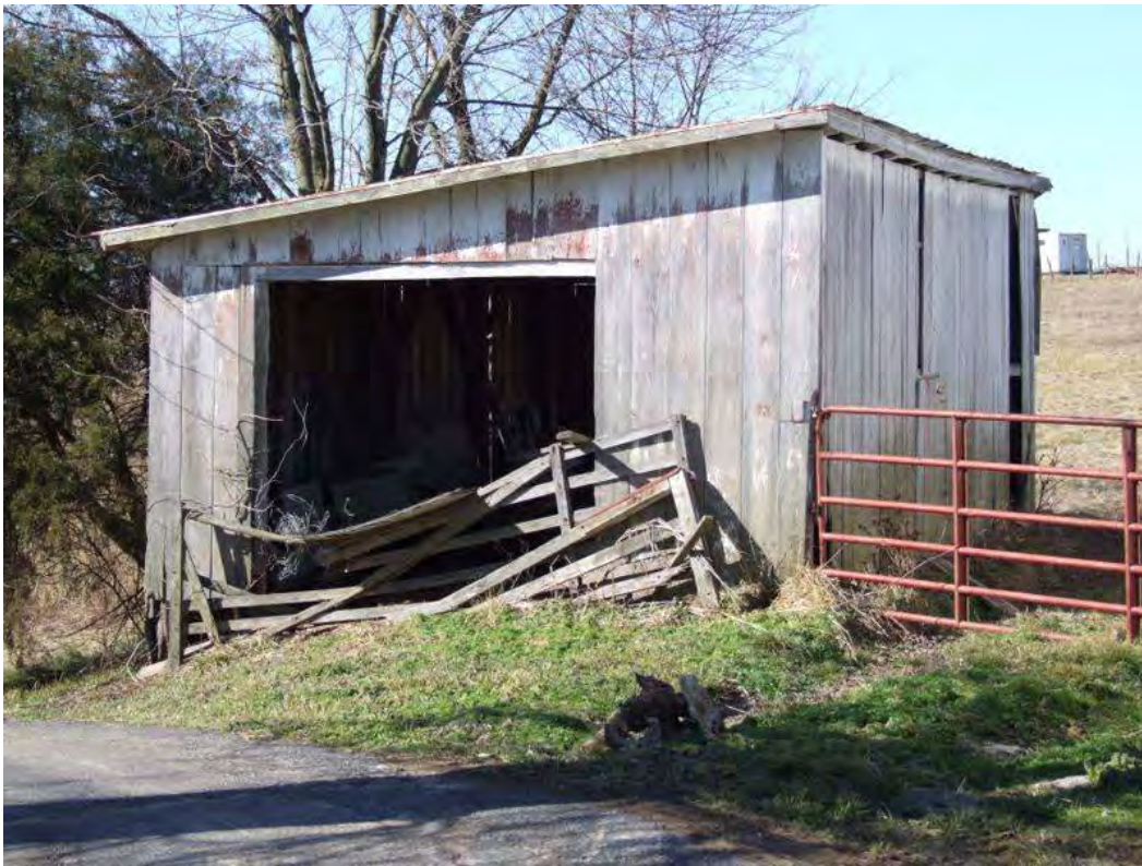
Figure 309: WS 590: Scale House, twentieth century, Mackville vicinity.
