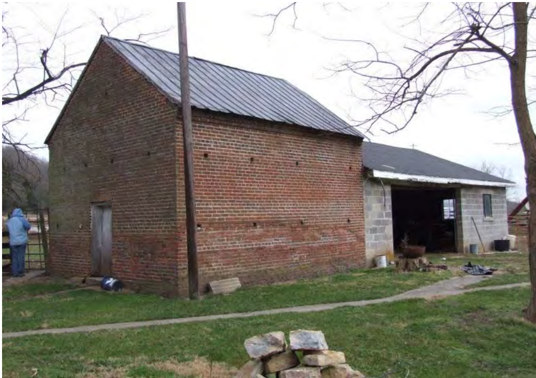
Figure 206: WS 187, Brick Smokehouse, Manton vicinity, early nineteenth century. A substantial and early brick example, with a corbelled cornice and a much later concrete block addition in back.
