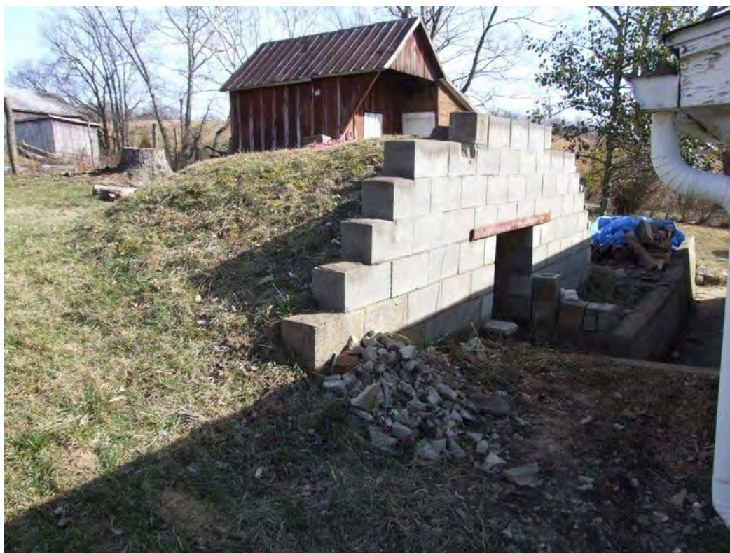
Figure 191: WS 476, Cellar, early twentieth century, Mackville vicinity.
