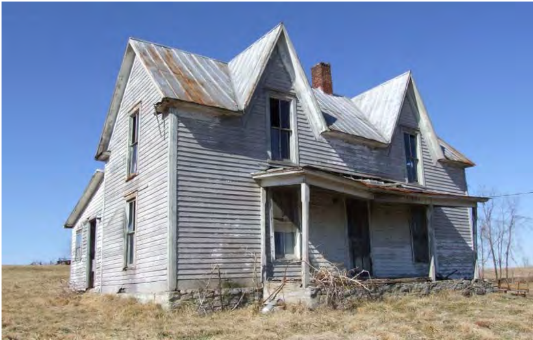
Figure 55: WS 523, frame two-gable Gothic house, center passage plan, late nineteenth century, Mackville vicinity.
