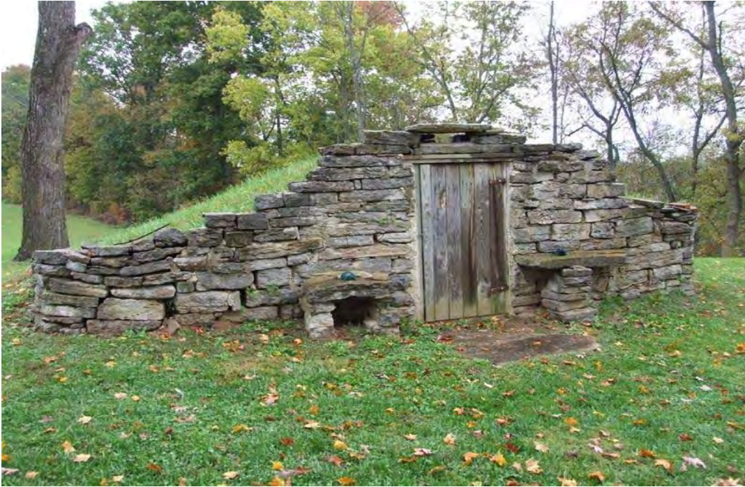
Figure 194: WS 365, Dry-laid Stone Cellar, late nineteenth century, Maud Vicinity.
