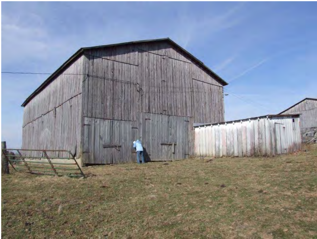
Figure 286: WS 476, Tobacco Barn with attached Stripping Shed, 1950-70, Mackville vicinity.
