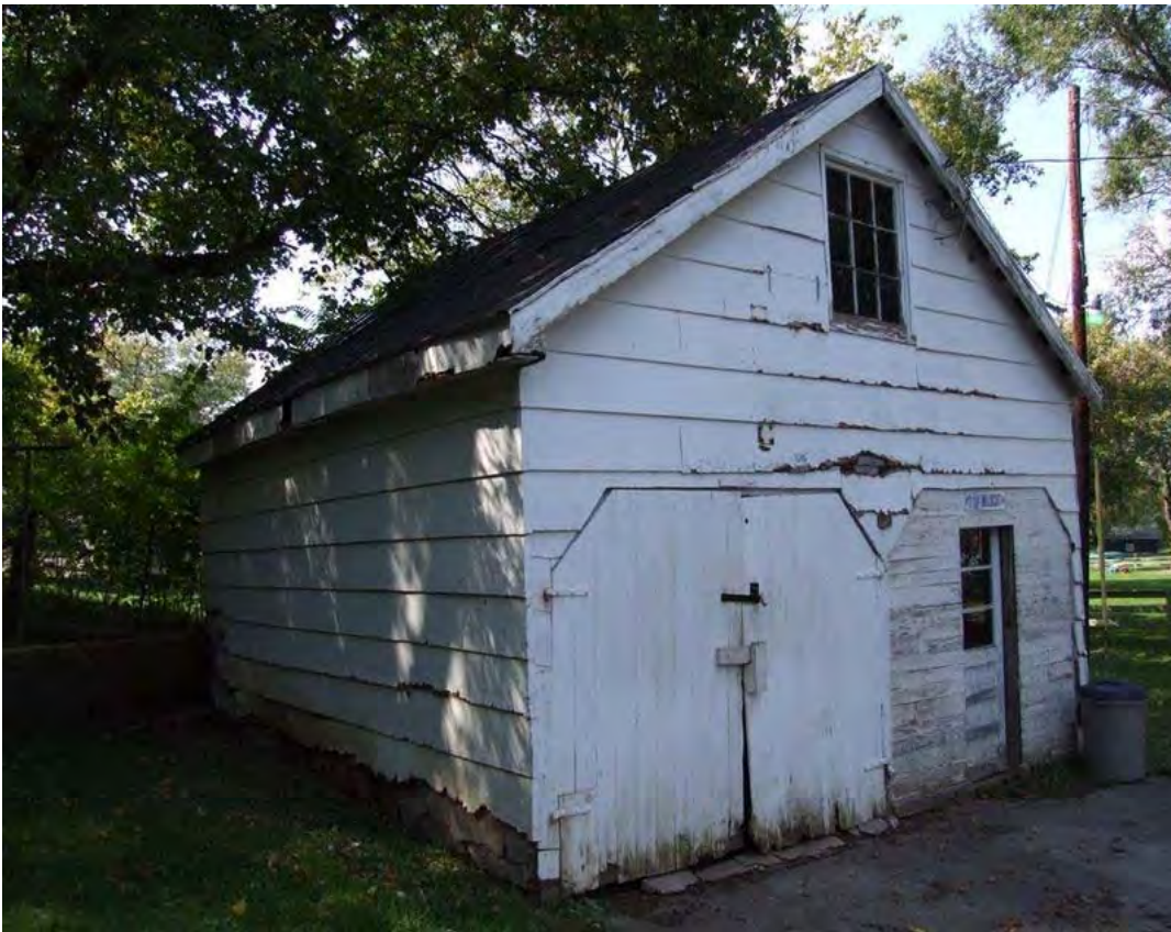
Figure 101: WS 349-50, shared garage, 1949. Built at the time the two houses were moved here from Fort Knox, the garage has no particularly stylistic details beyond the 6-pane window sash on the front gable. See also Figure 99 and Figure 100.
