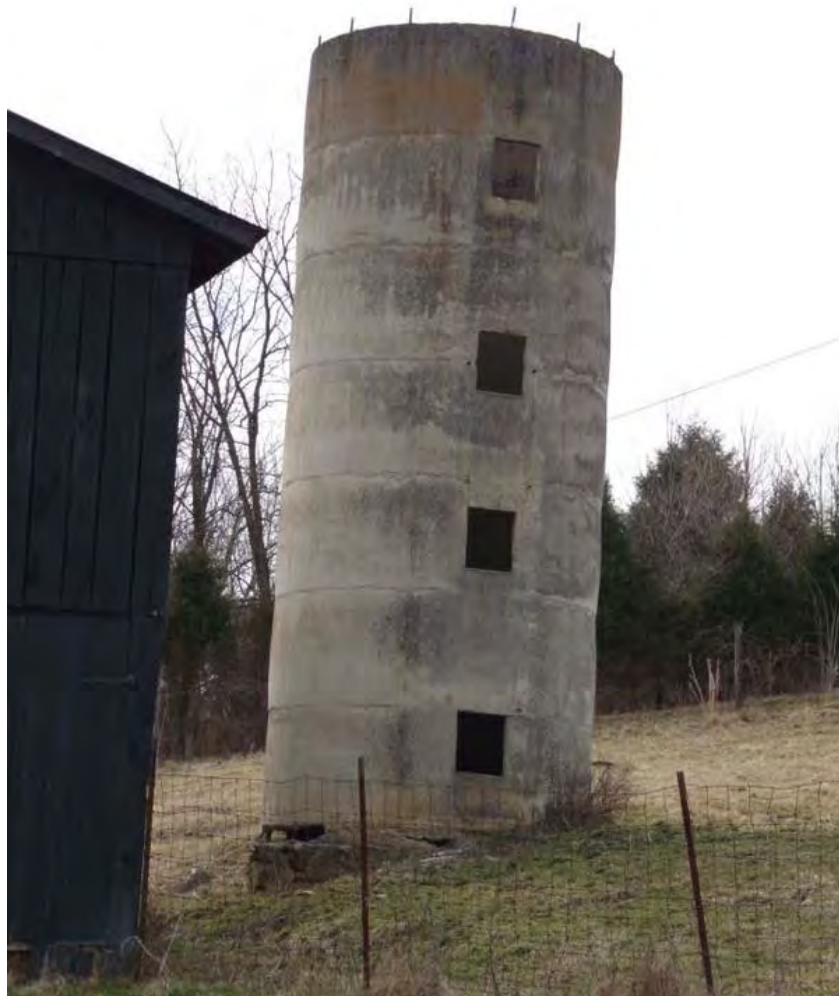
Figure 315: WS 580, Poured Concrete Silo, mid twentieth century, Texas vicinity.
