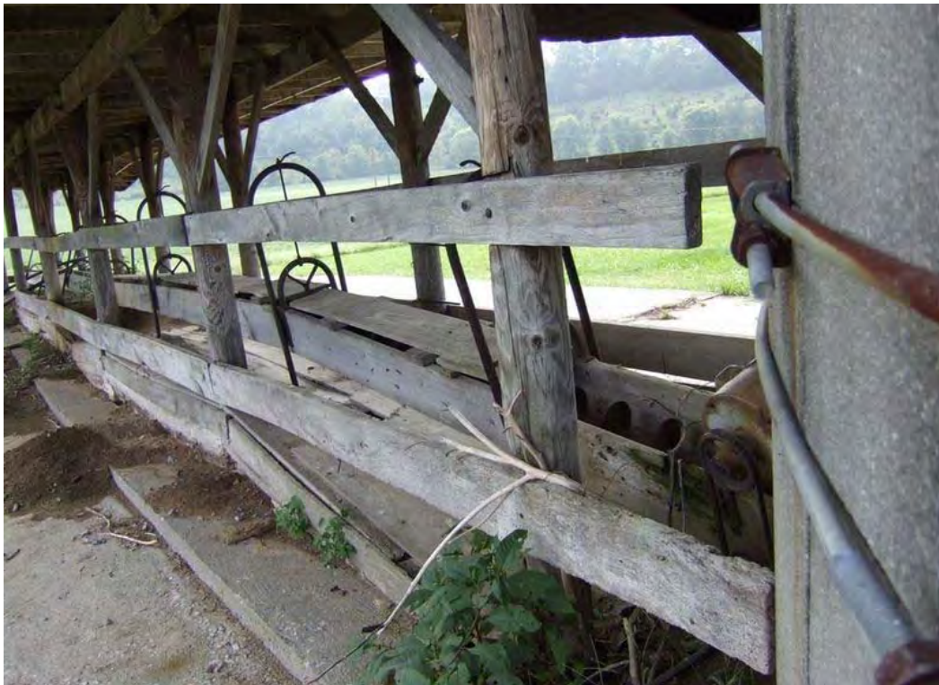
Figure 317: WS 27 Feed Carrying Mechanism and Feed Shed attached to Silo, mid twentieth century, Maud vicinity.
