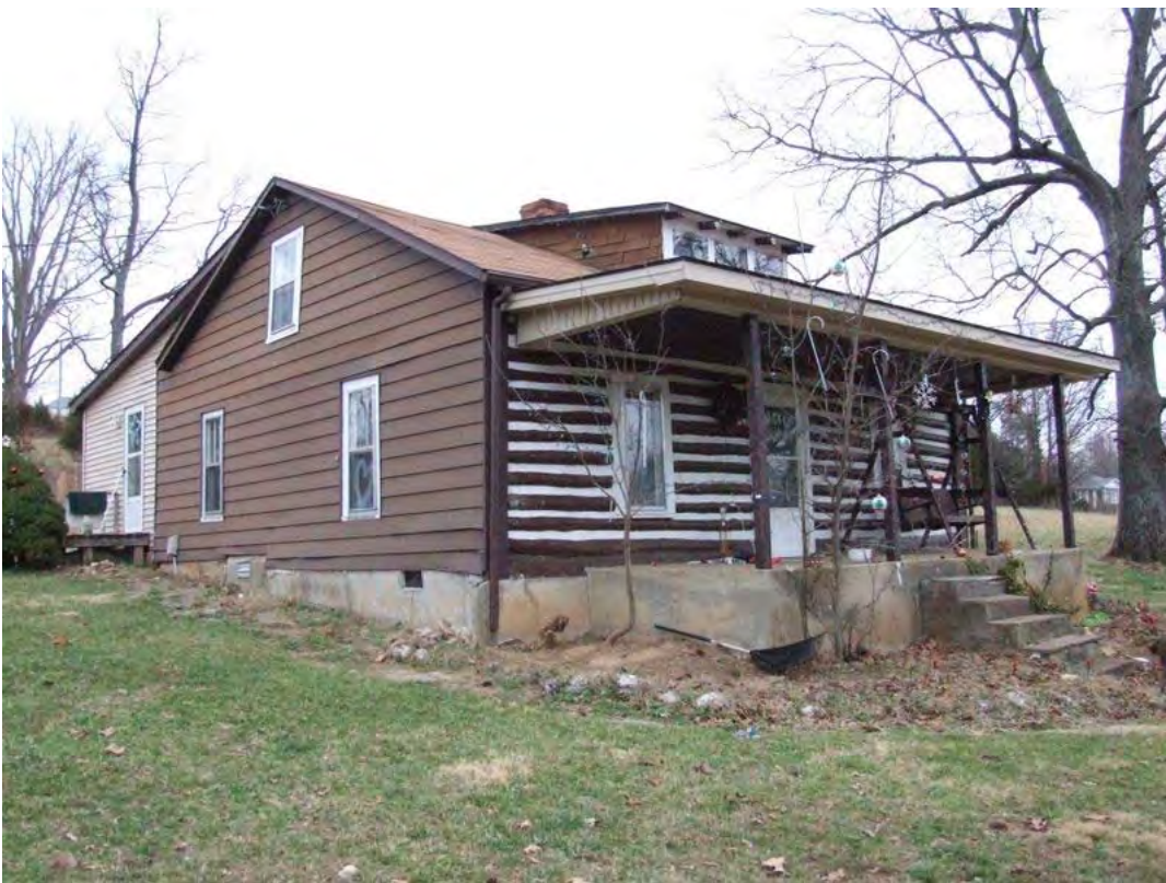
Figure 115: MN 323, early –mid twentieth century, Dant vicinity. The log wall on the front is an applied veneer to the frame building.
