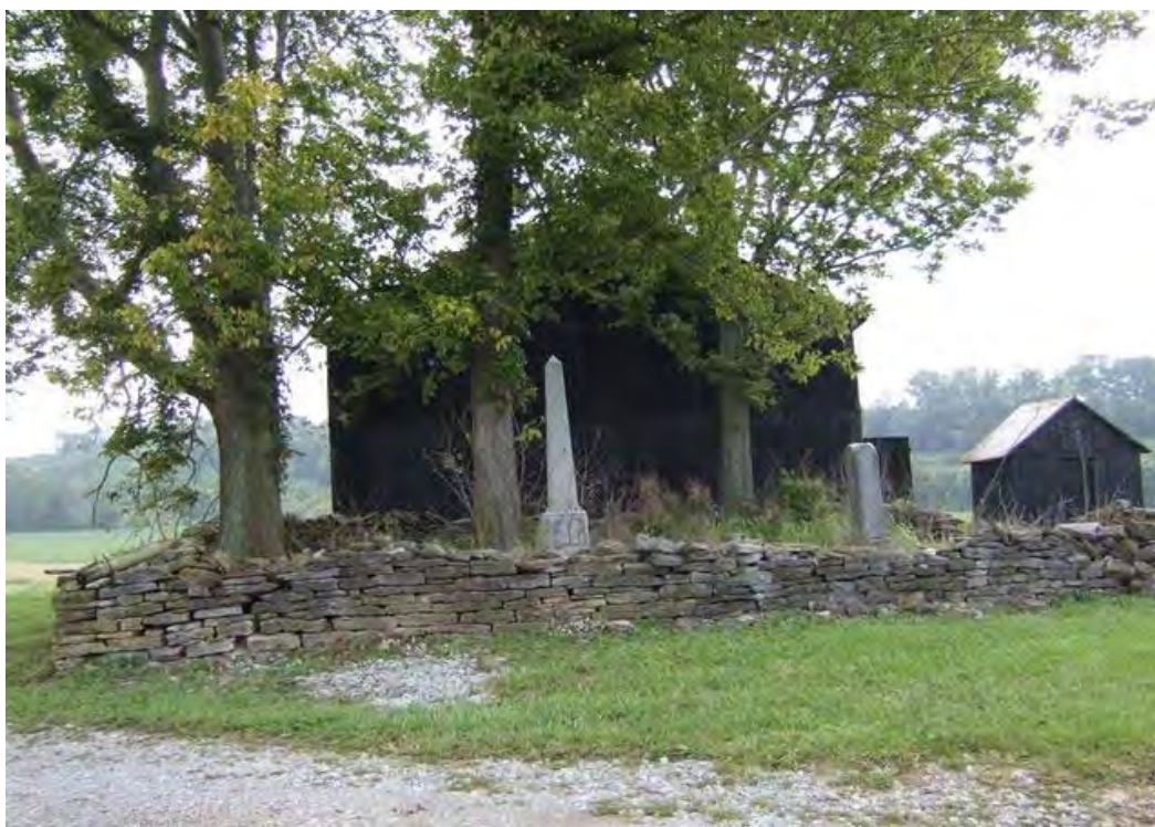
Figure 326: WS 27, Cemetery, Maud. This cemetery is located at the Benjamin Pile House, a previously surveyed National Register listed property (see Figure 25). Benjamin Pile's 1851 grave is here, along with his wife, members of his family, and later descendents. Family cemeteries were often surrounded by stone fences to keep livestock out.
