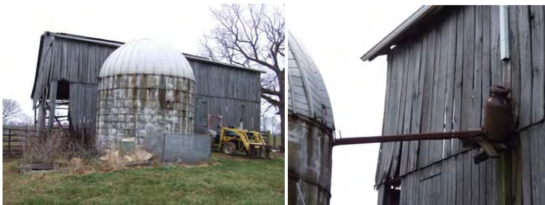
Figure 230: MN 474, Multi-purpose Barn, early-mid twentieth century, with adjacent concrete Cistern, and detail right, Pottsville vicinity. Note the milk can used to connect the guttering.
