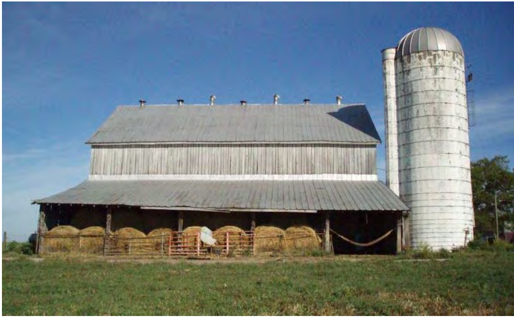
Figure 314: WS 287, Concrete stave Silo and Feed Barn, Mooresville vicinity.
