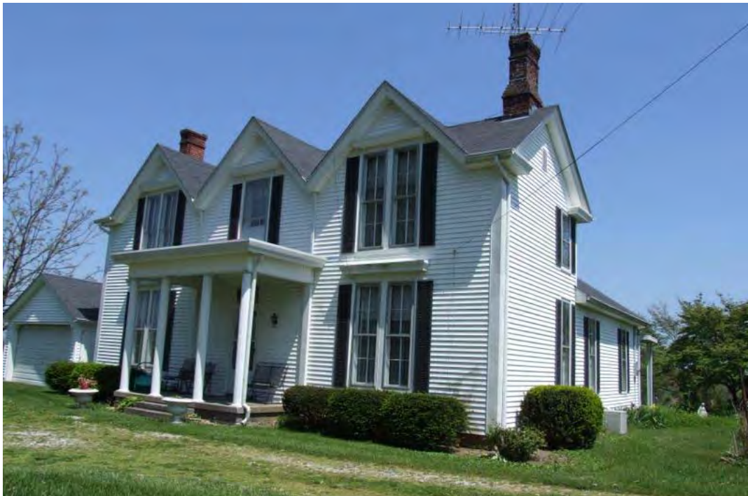
Figure 66: MN 552, Cecil house, late nineteenth century, St. Mary vicinity.
