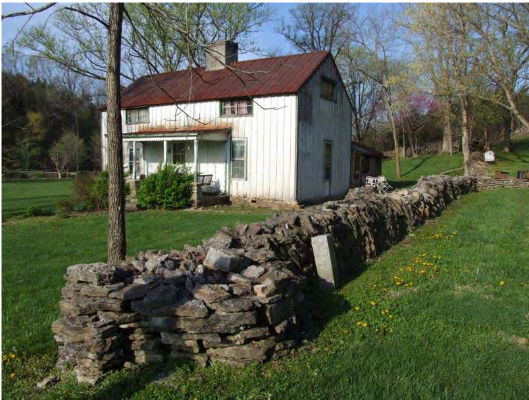
Figure 344: WS 720. Center chimney double pen House with board and batten siding, early-mid nineteenth century, Manton vicinity. Extensive stone fencing separates domestic and agricultural spaces. See also Figure 345 and Figure 346.
