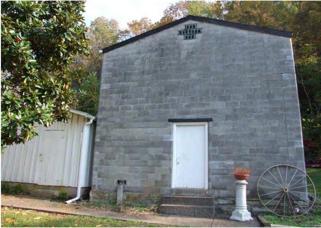
Figure 208: WS 333, Leo Mudd's Smokehouse. Built in the 1950s by Leo Mudd in concrete block, on the cut stone foundation of an earlier smokehouse. Leo was known for the high quality of the hams he smoked here and sold from his store. The ventilators at the peaks and at regular intervals above the foundation were created by turning the blocks sideways.
