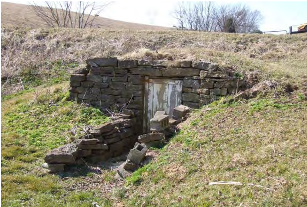
Figure 193: WS 633, Dry laid Stone Bank Cellar, late nineteenth century, Deep Creek vicinity.
