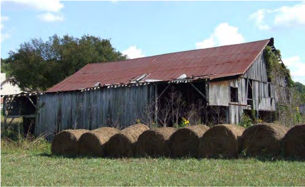
Figure 259: WS 98, Multi Purpose Barn, early twentieth century, Fredericktown vicinity.
