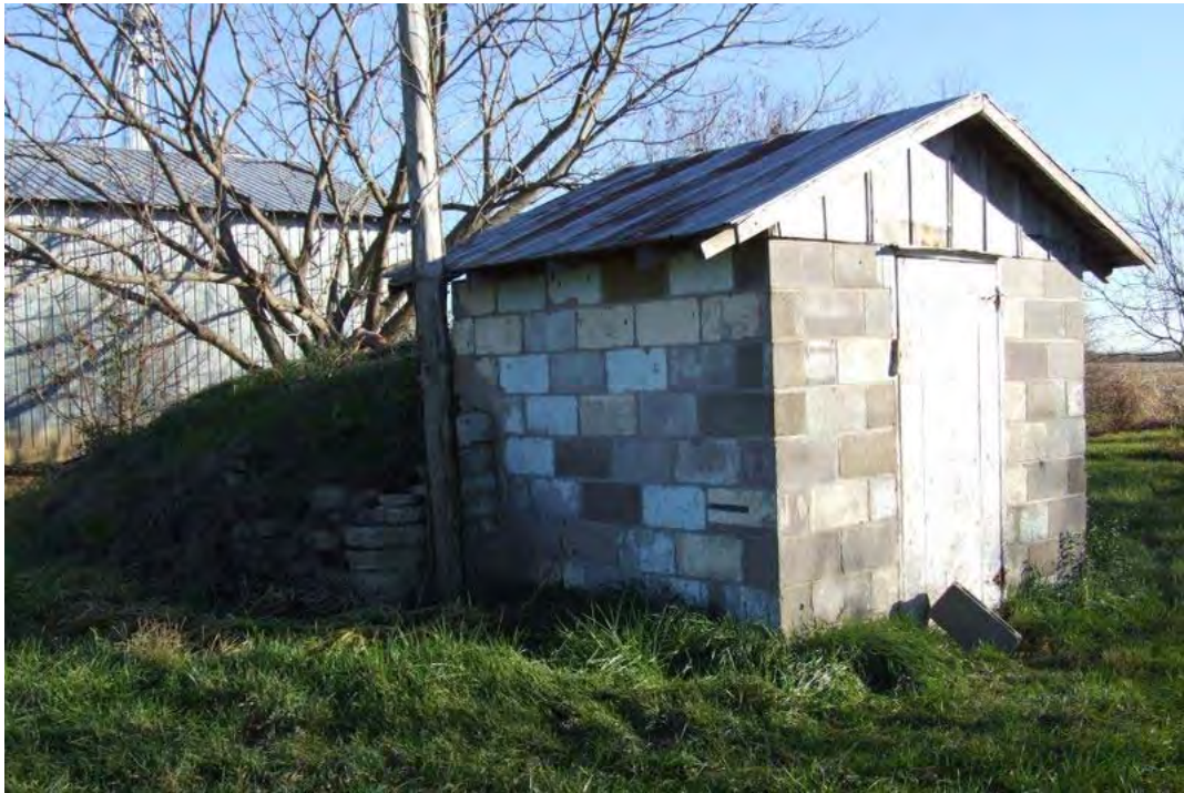
Figure 198: MN 205, Mid-twentieth century Concrete Block Entry Shed over older Brick-lined Cellar, Holy Cross vicinity.
