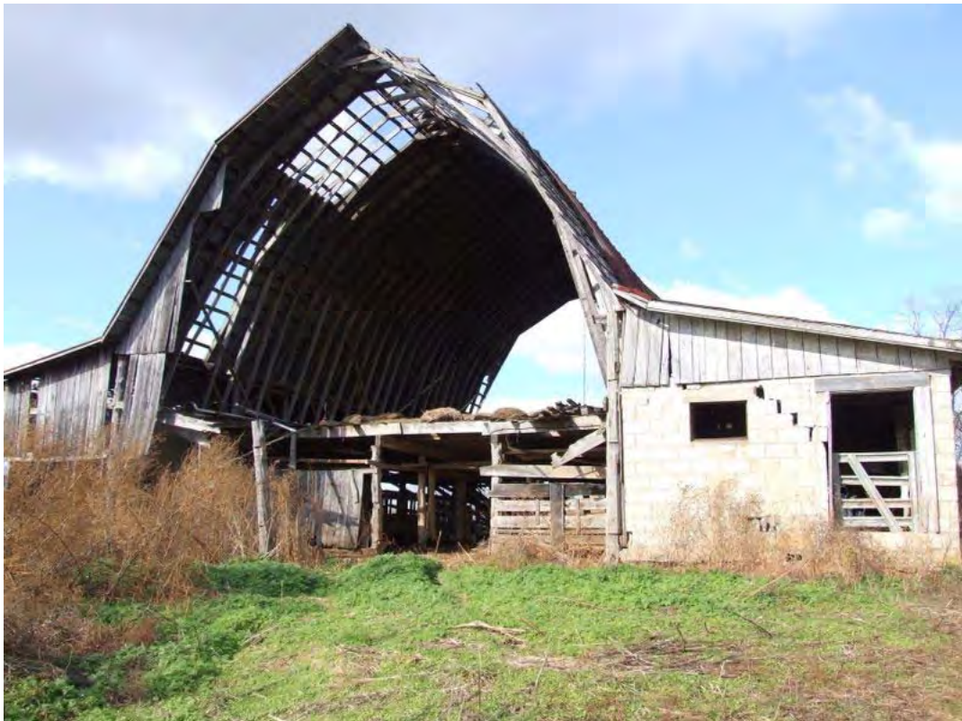
Figure 253: MN 188, Multi-purpose or Dairy Barn, 1920s, Holy Cross vicinity.
