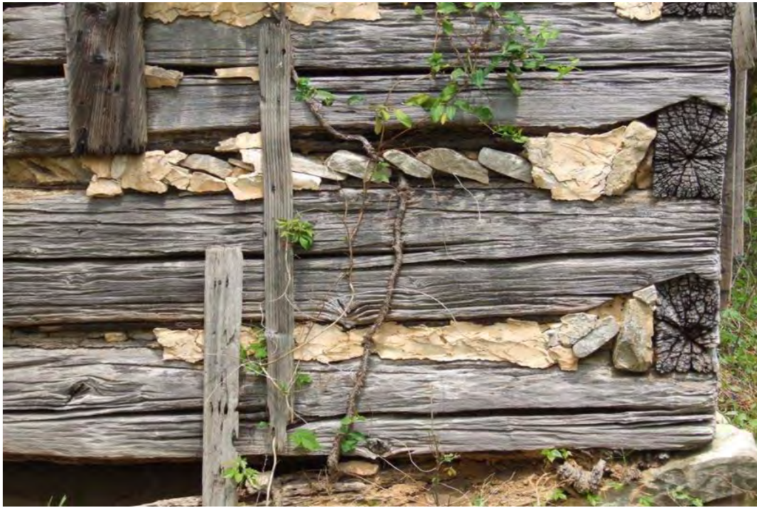
Figure 14: MN 80, Log House, early nineteenth century, Mt. Gilboa vicinity: detail of wall and corner notching.
