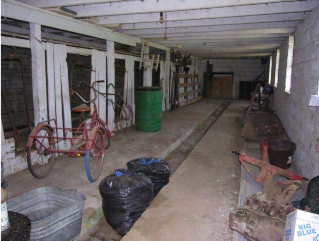
Figure 22: WS 974, Cheser Dairy Barn, 1949, Willisburg. Interior view of milking parlor with poured concrete floor and concrete block walls. See also Figure 276.
