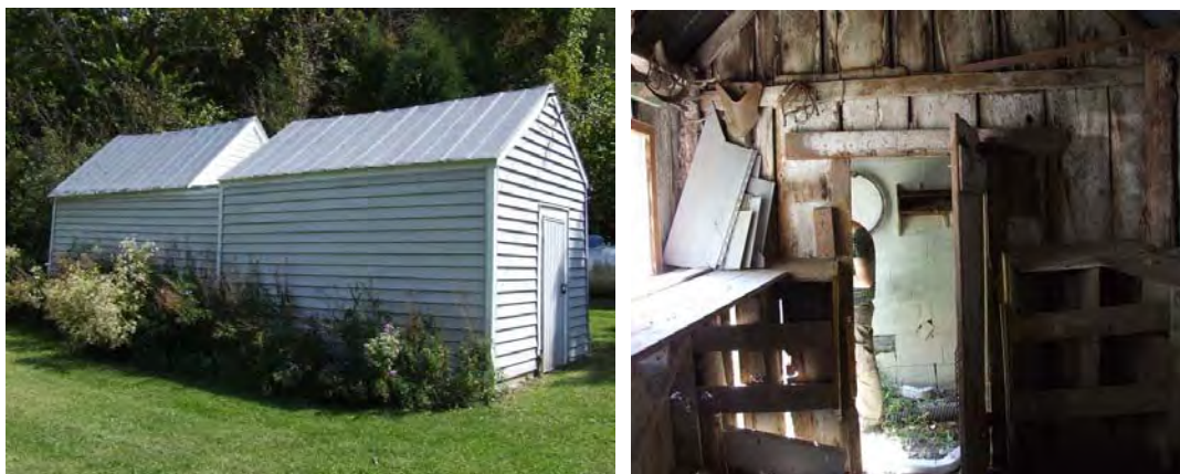
Figure 290: WS 307, Exterior, left, and interior, right. Early-mid twentieth century vertical plank frame Chicken House adjacent to a Well House behind. Laying boxes are visible in the interior, right.
