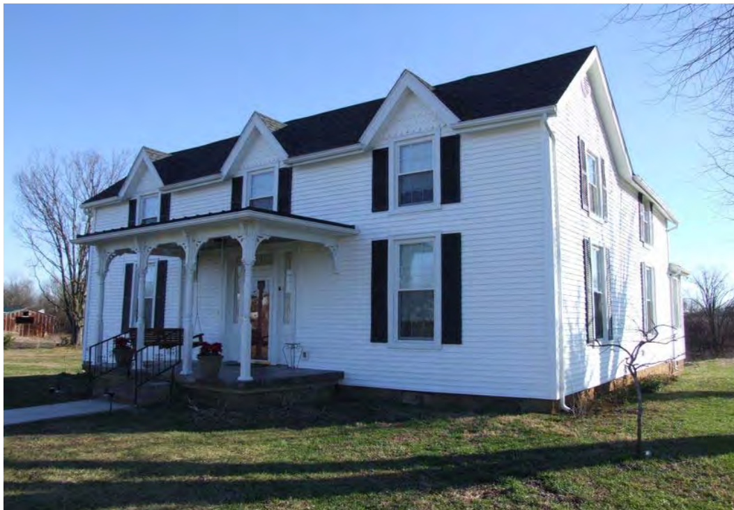
Figure 31: MN 336, exterior. The survey forms codes its stylistic influences as mid 19 th century Romantic and Gothic Revival, but the exterior also shows influences of Queen Anne and Shingle style, due to a series of alteration and renovation. See also Figure 30.
