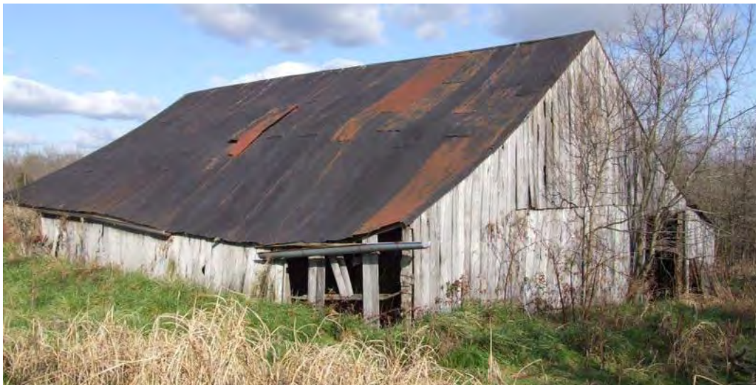
Figure 258: MN 189, Multi-purpose Barn , late nineteenth-early twentieth century, Manton vicinity
