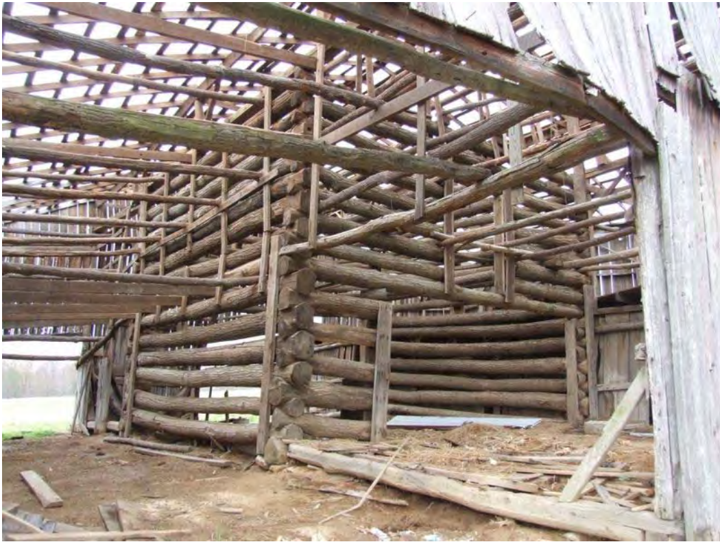
Figure 247: MN 509, interior. See also Figure 246.
