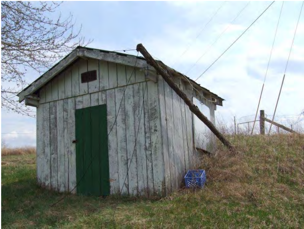
Figure 197: MN 480, Cellar with Frame Entry Shed, early-mid twentieth century, Pottsville vicinity.
