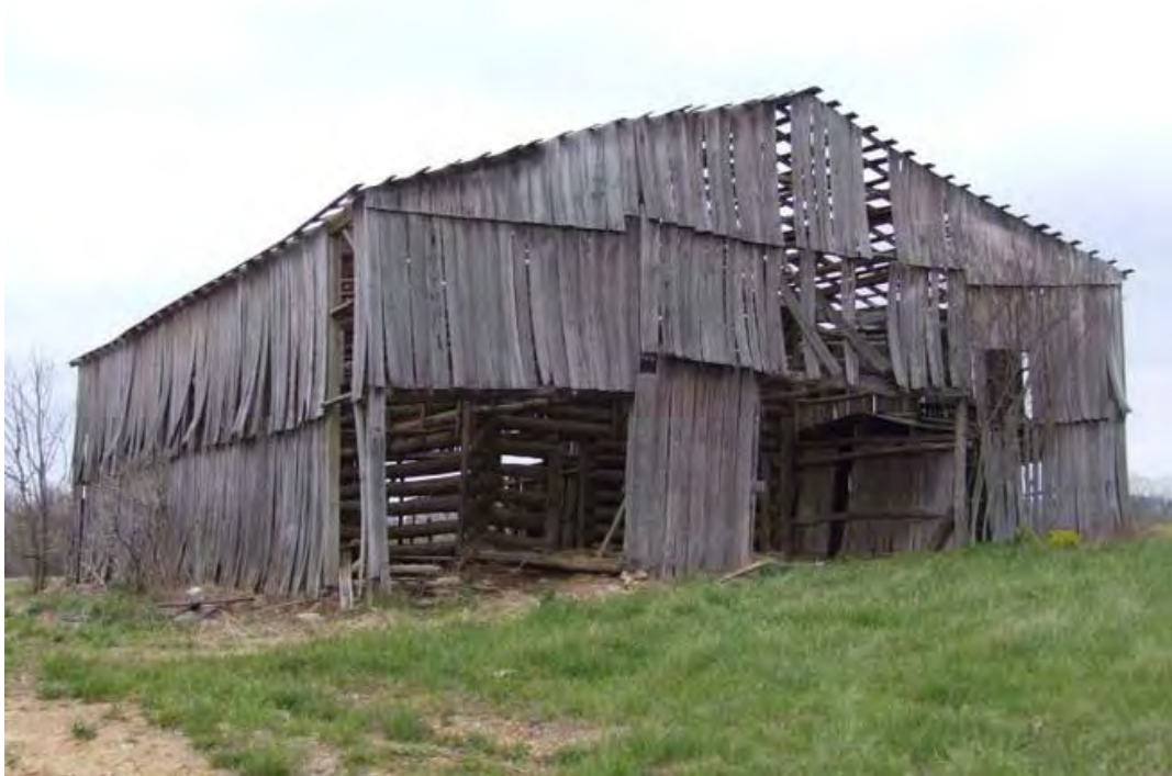
Figure 246: MN 509, Log crib barn, early twentieth century, Raywick vicinity, exterior. See also Figure 247.
