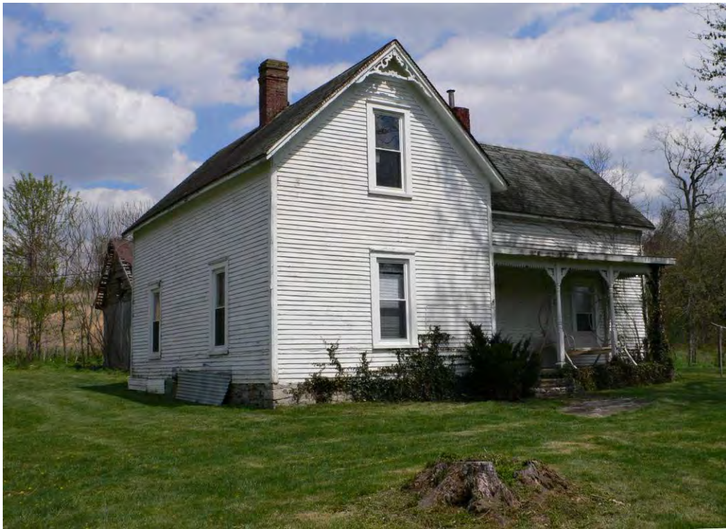
Figure 87: MN 666, Late nineteenth-early twentieth century, Gravel Switch vicinity. The outbuilding just visible behind the house to the left is found in Figure 132.
