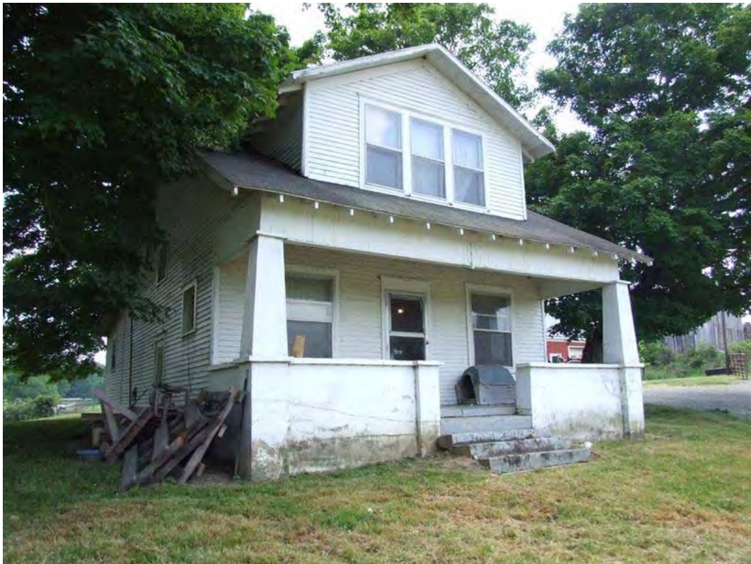
Figure 113: WS 891, early twentieth century, Simstown.
