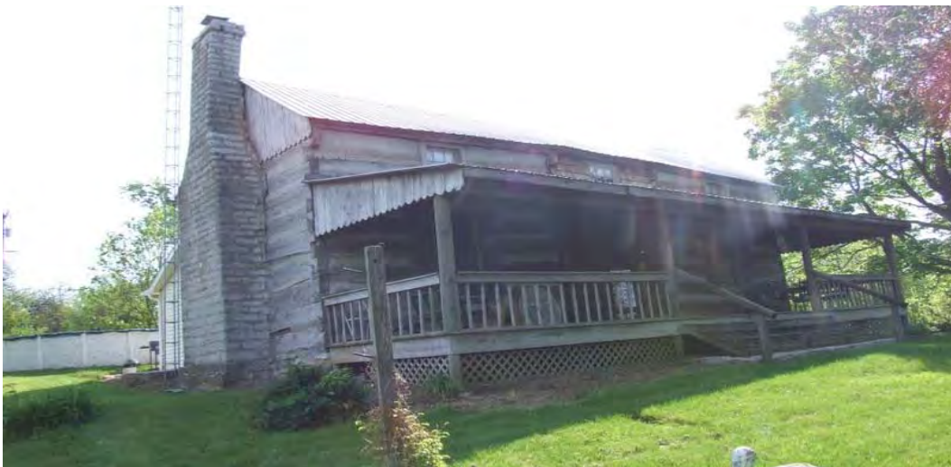
Figure 154: MN 554, Dogtrot type house. A log house constructed in the first half of the nineteenth century, St. Mary vicinity.
