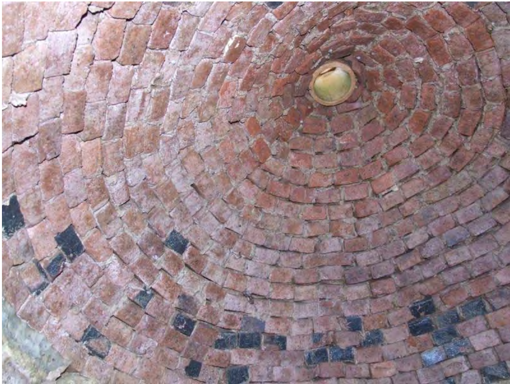
Figure 196: MN 273, Cellar, ca 1860-1900, Holy Cross. Interior view of brick dome ceiling.
