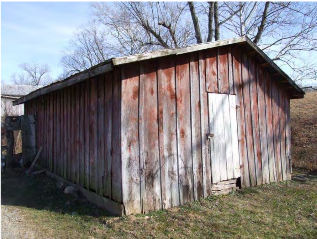
Figure 216: WS 476, Workshop or Tool Shed, mid-twentieth century, Mackville vicinity.
