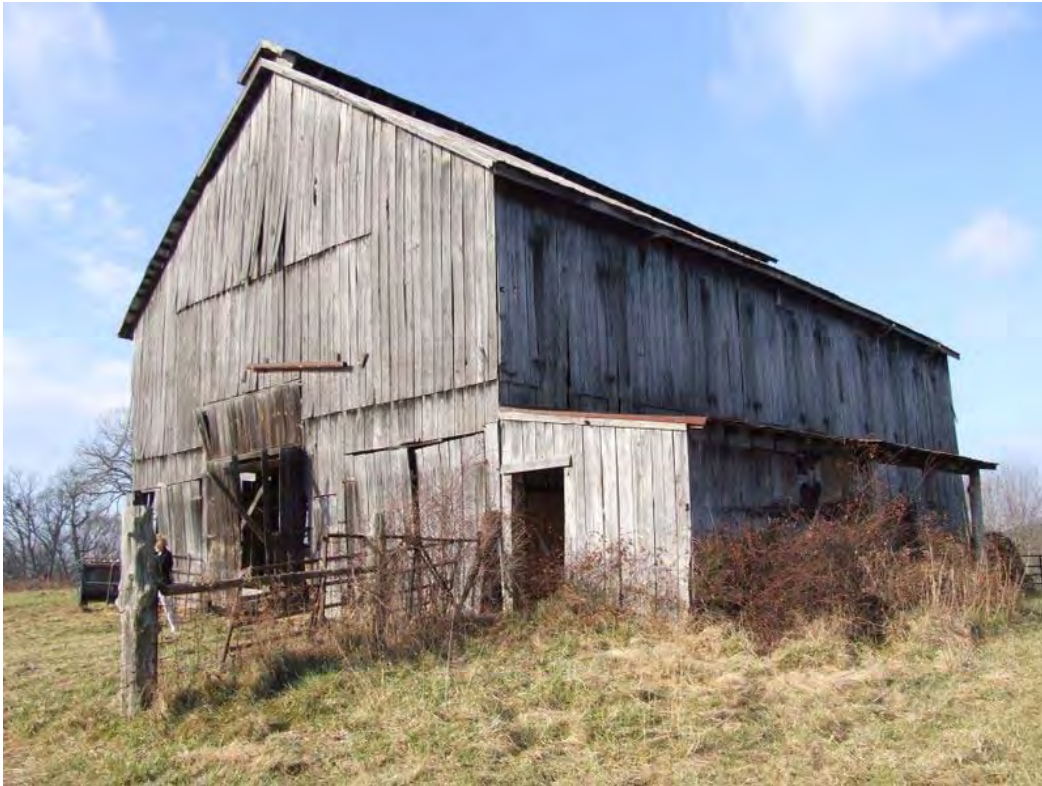
Figure 281: MN 273, Caleb Ballard Farm, Frame Tobacco Barn with roof ventilator, 1939, Holy Cross.
