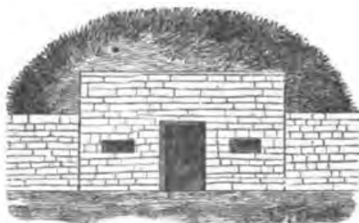
Fig. 233.—STONE FACING OF HILLSIDE CELLAR.
