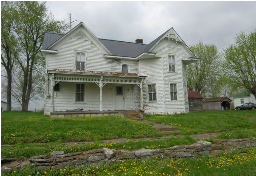
Figure 82: WS 171, John Harmon House, late nineteenth century, Mackville.
