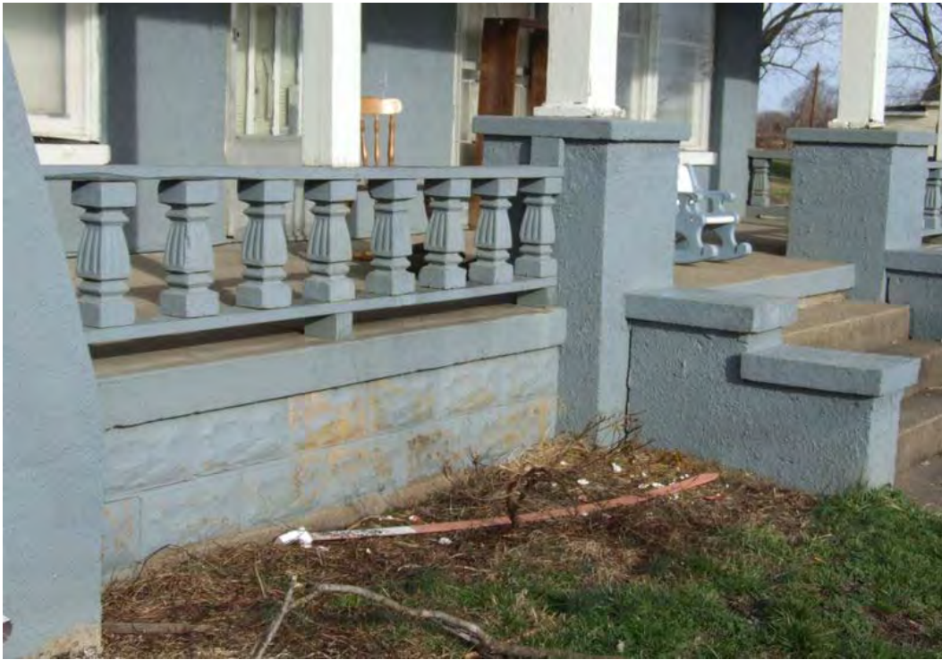
Figure 106: MN 359, detail of porch. See also Figure 105.
