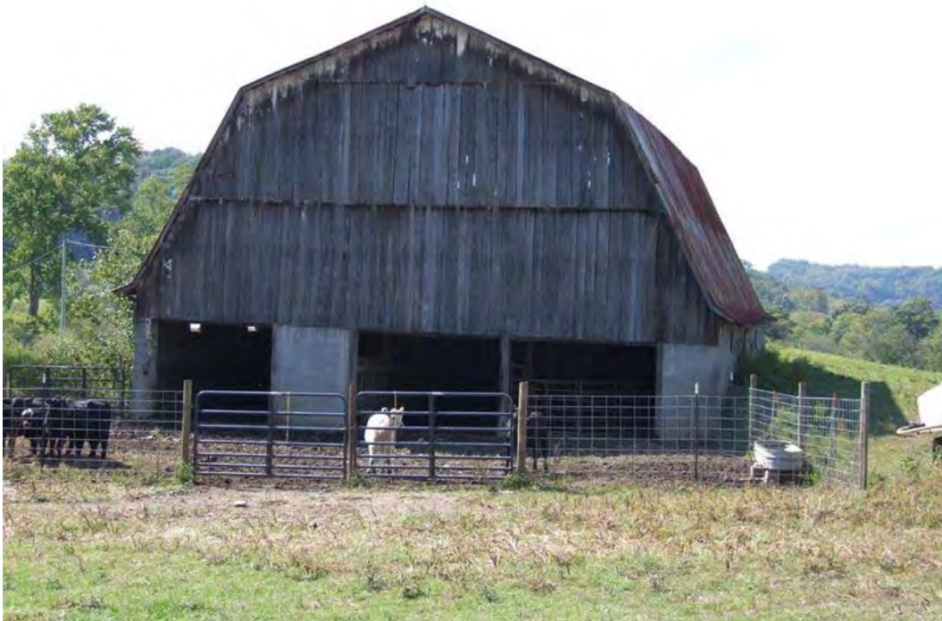
Figure 273: WS 98 Dairy Barn, downhill façade. See also Figure 271 and Figure 272.
