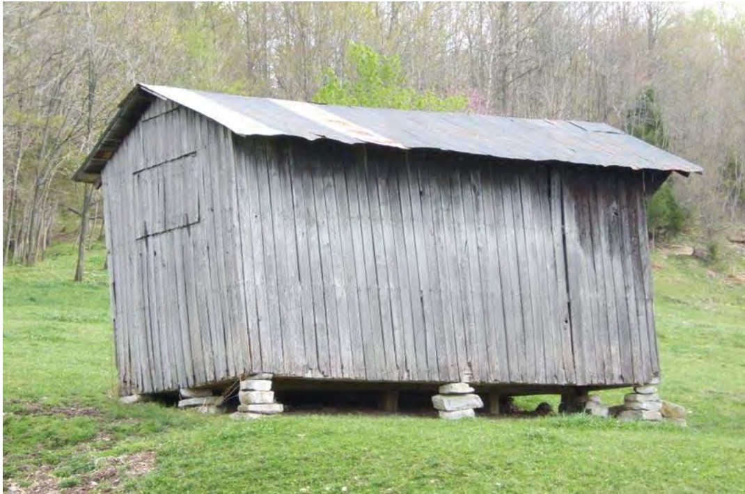
Figure 307: MN 655, Ellis Farm: frame, single pen Corn Crib, late nineteenth-early twentieth century, Bradfordsville vicinity.
