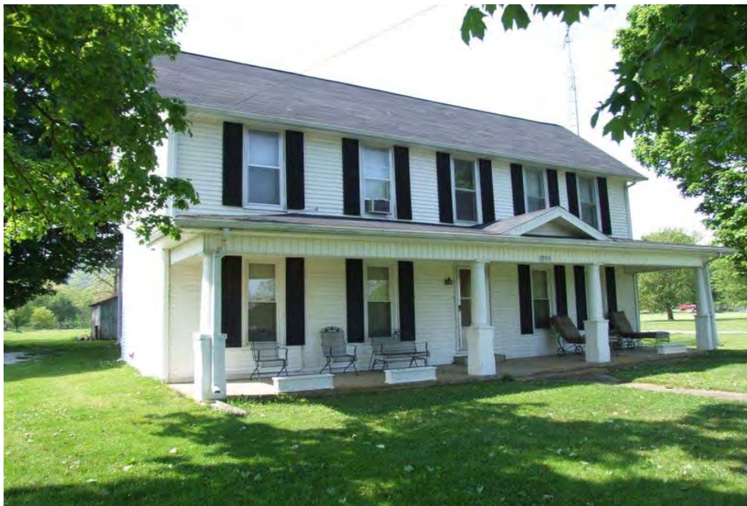
Figure 157: MN 567, center passage, single pile house, late nineteenth-early twentieth century, New Market.
