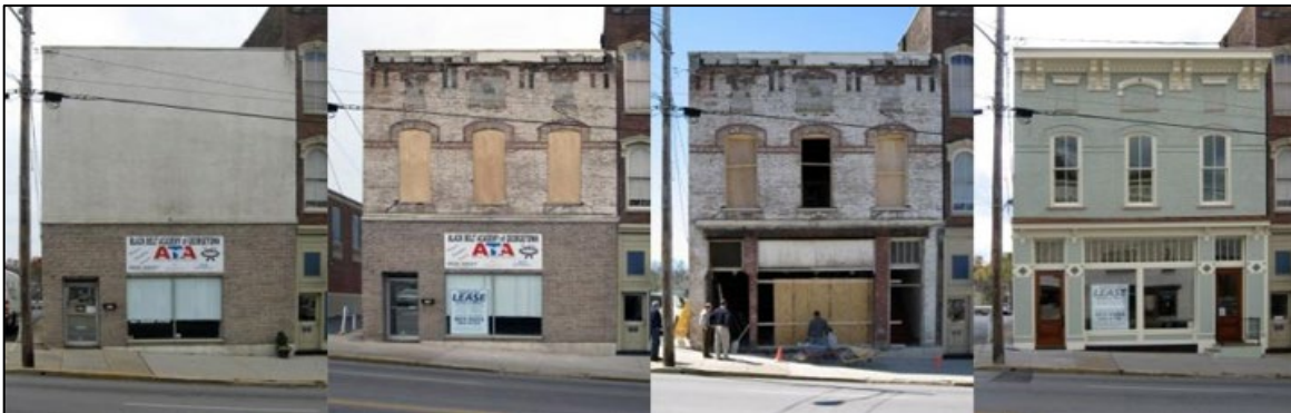
Figure 1 – Photo-Documentation for State & Federal Rehabilitation Tax Credits in Georgetown, KY
