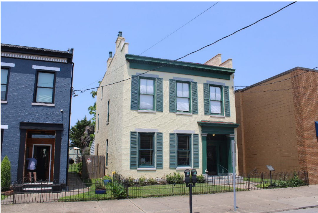
Locally Designated Landmark and Contributing Resource at 17 E 6 th St., facing north.
