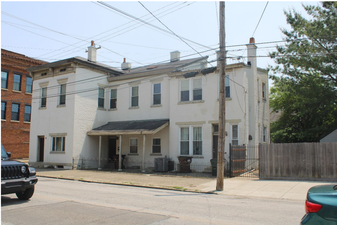
Contributing Resource at 14-22 E 9 th St., facing east.
