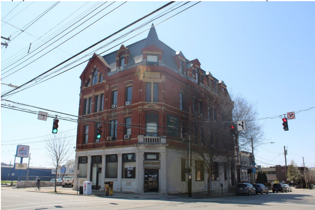
Contributing resource at 4 W 4 th St., facing south.
