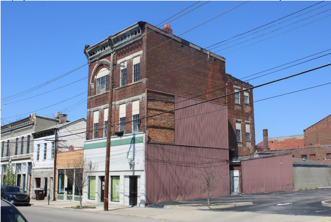
Streetscape of Contributing Resources along east side of York St., facing north.
