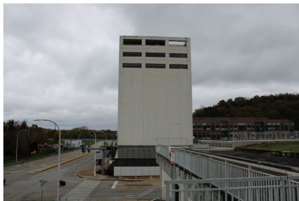
South Façade, camera facing northeast
