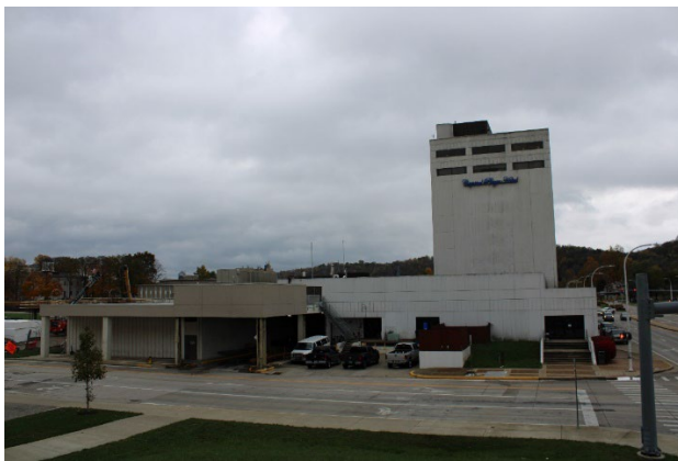
North Façade, camera facing southwest
