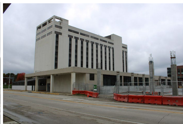
East Façade, camera facing north
