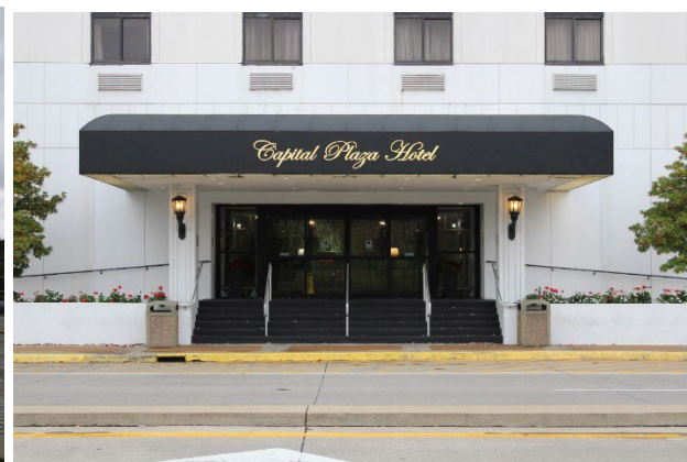
Front entrance, West Façade
