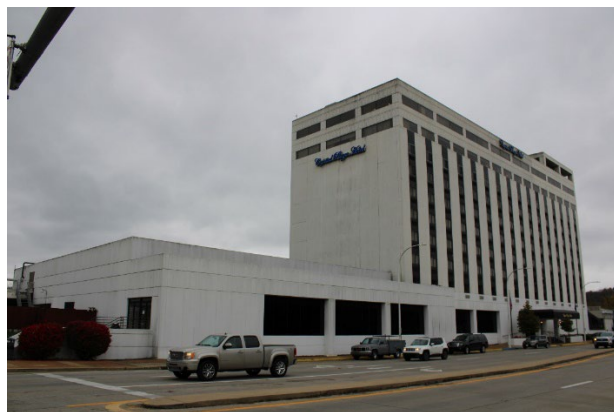
North and West Façades, camera facing south
