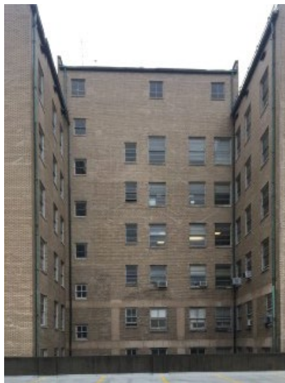
Windows on north elevation, 2018
