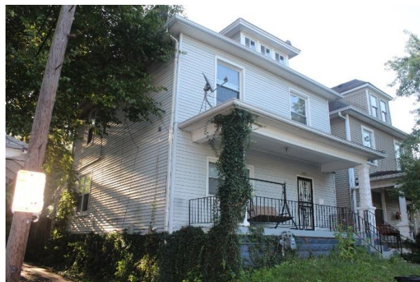
Foursquare type, 1223 S. Clay Street
