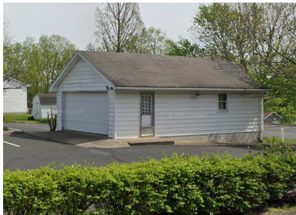
Garage near the Southwest corner of site
