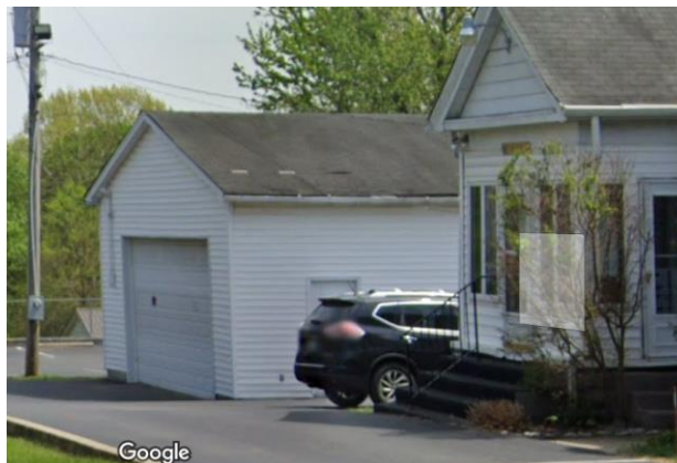
Garage behind rectory
