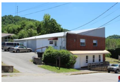
Resource 37 (Photo # 36), looking SE.
