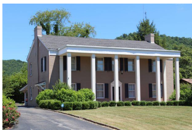
Resource 21 (Photo #24), looking SE.
