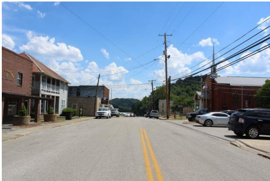
Figure 4. Overview of Main Street, looking south (Photo #3).
