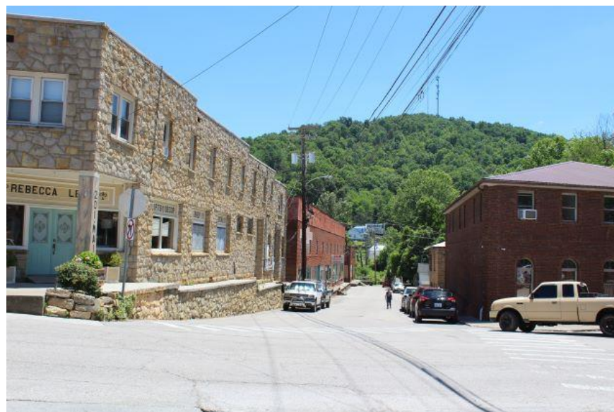
Figure 3. Overview of Bridge Street, looking east (Photo #2).
