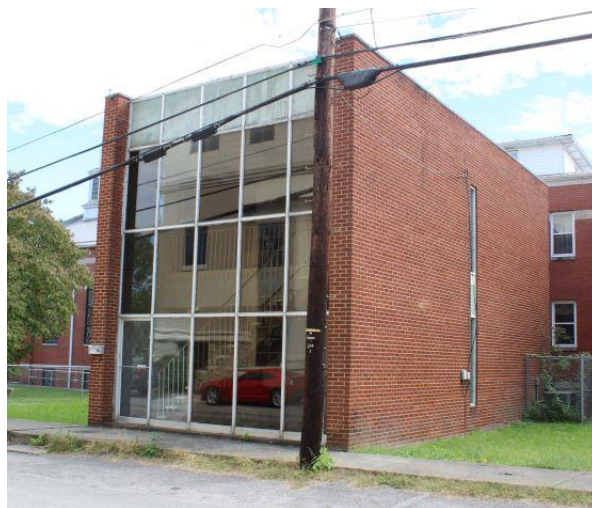
Resource 27 (Photo #30), looking SE.
