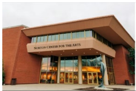
West side entrance
